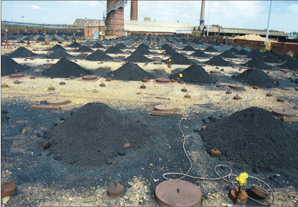
Figure 14 CK1, roof © Historic England
