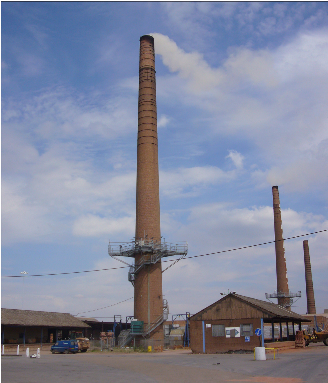
Figure 1 General view of site with chimneys. © Historic England Archive (P1000268)
