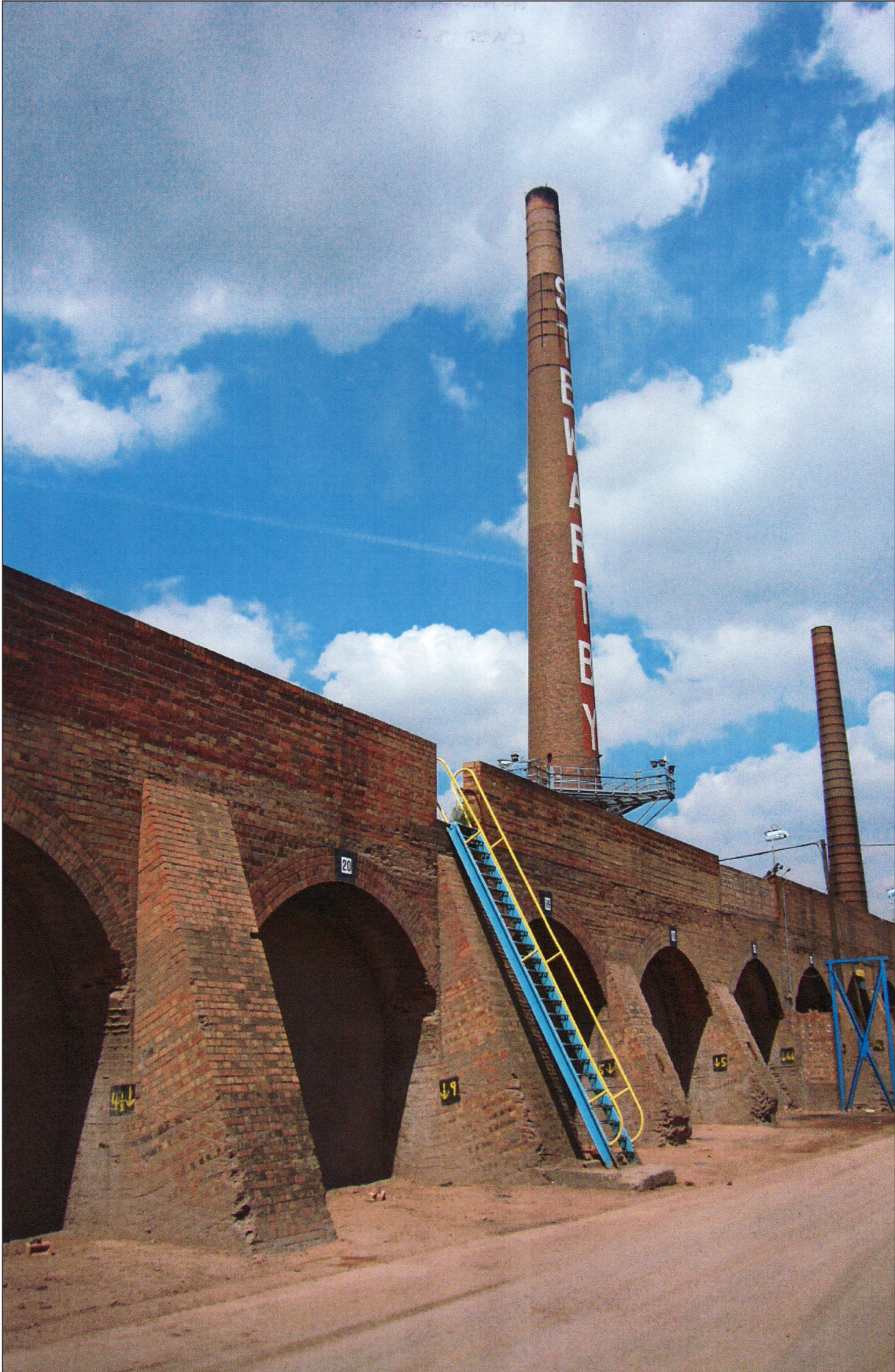
Figure 13 CK1, general view © Historic England
