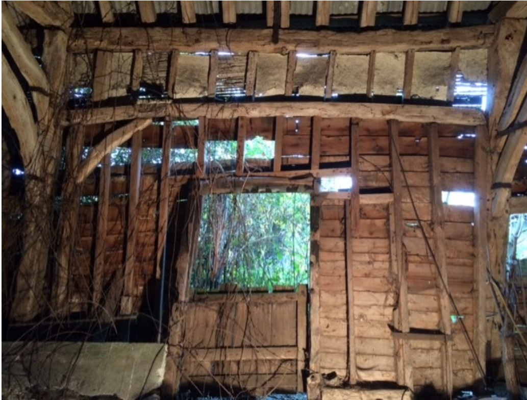
Figure 9: Doorway D4, photograph taken from the west (Alison Arnold)
