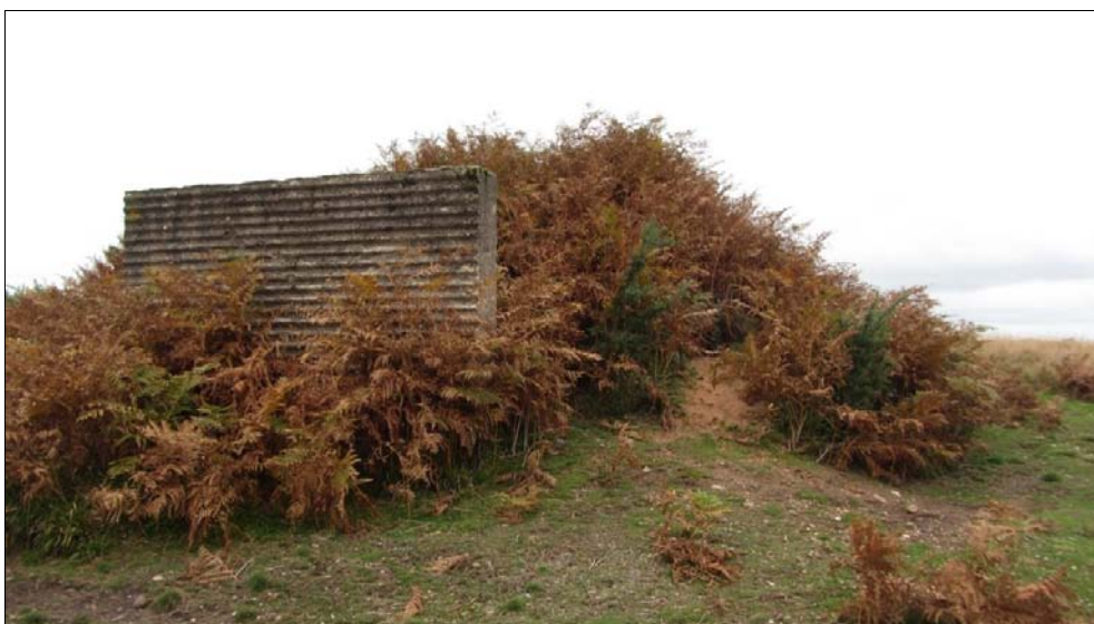
Figure 64. Concrete blast wall and embankment of the control centre MDV70415. Photograph by Stephanie Knight, October 2015.
