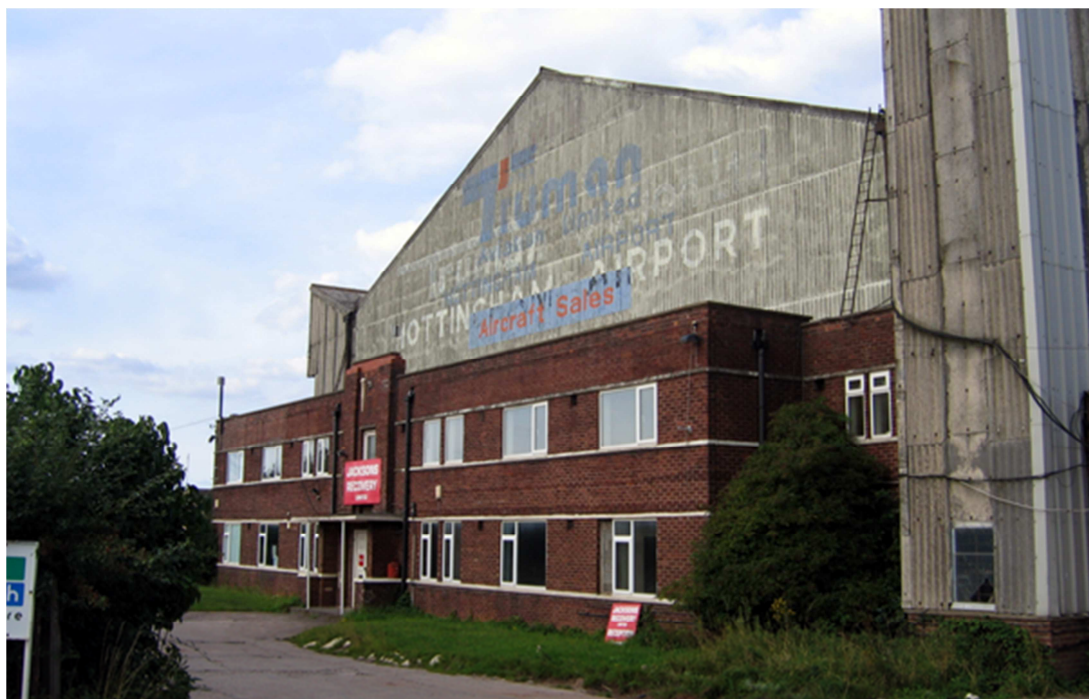
Figure 6: There are two ladders, one at either end of the roof truss, allowing access to the pair of roof gullies. [Milan Petrovic 07-08-2009]
