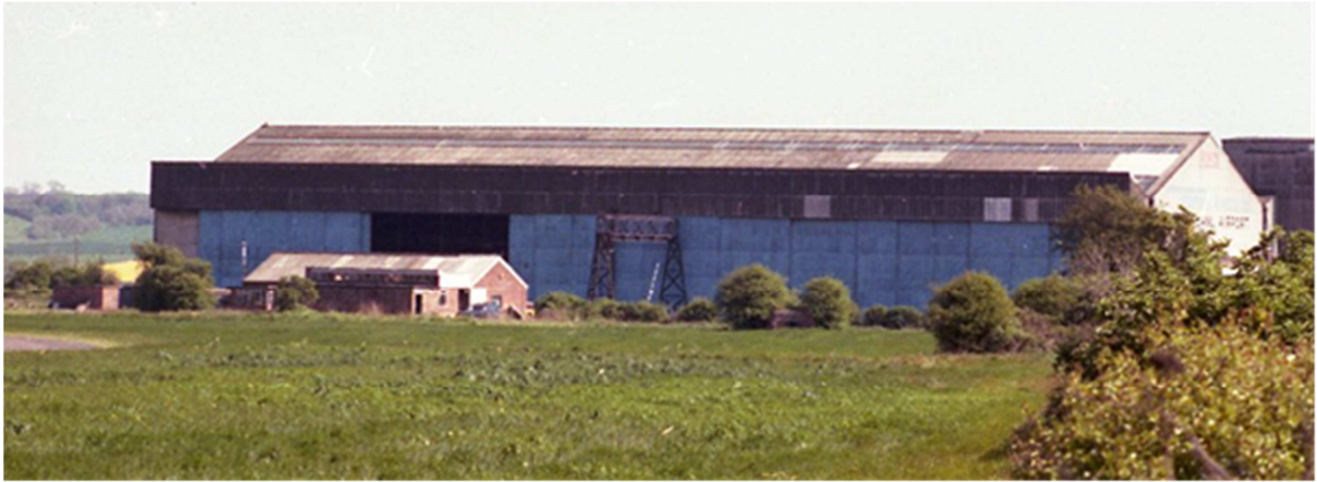
Figure 27: Main hangar (Bldg.43) with engine gantry. [Paul Francis 1987]
