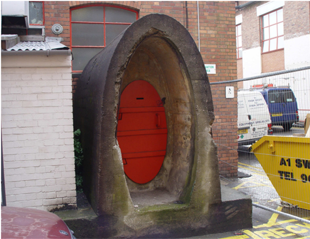
Figure 24: Concrete fire watcher's shelter at the Bristol Aeroplane factory – NGR: ST 59969 79218, Filton (one of many built there). [Paul Francis 22-06-2005]
