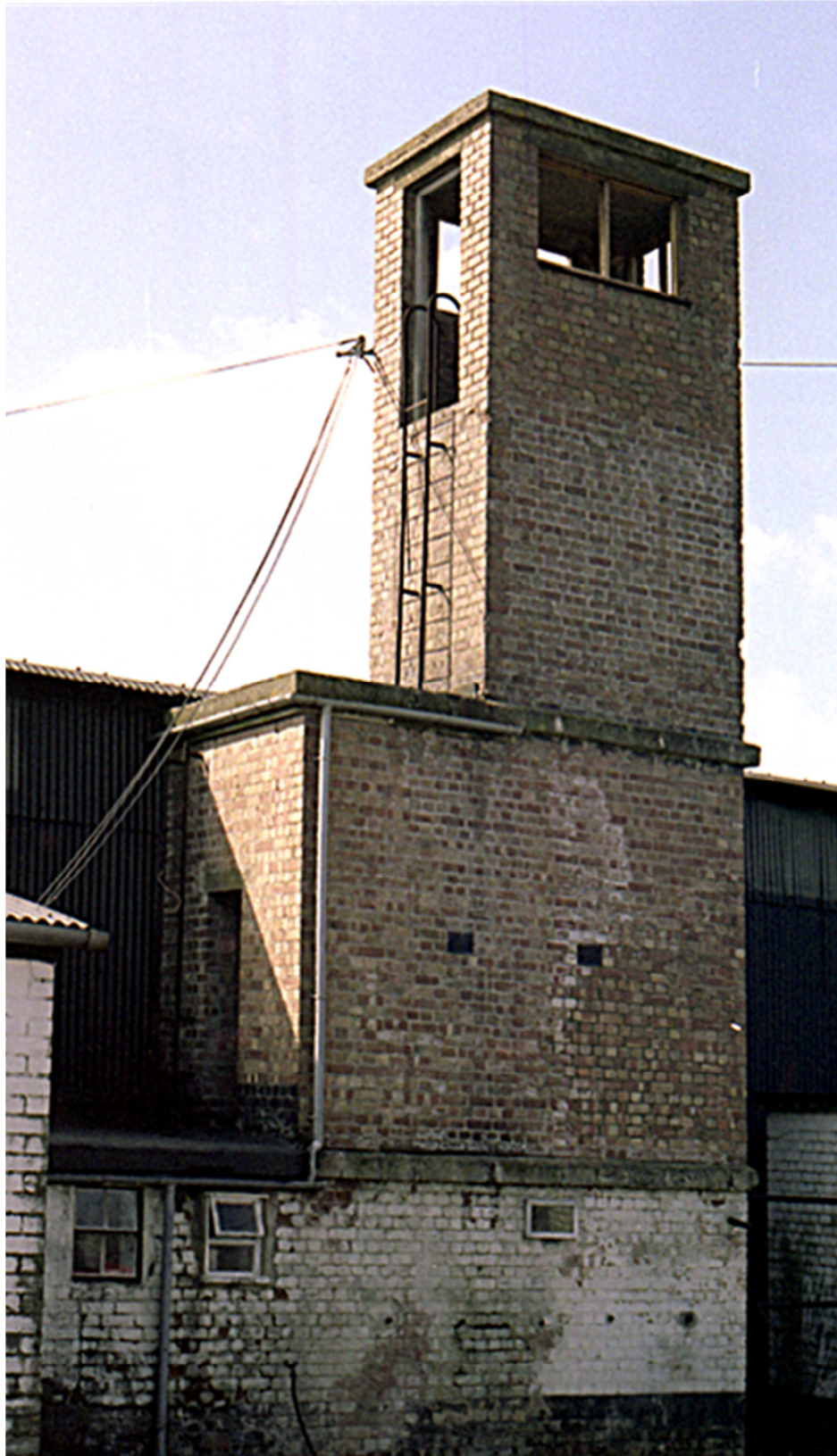
Figure 22: Built above the toilet annexe is this external example - NGR: SP 33466 61235, at Bishop's Tachbrook - a Stirling aircraft repair factory. The extra height enabled good views over two Bellman hangars. [Paul Francis 1993]
