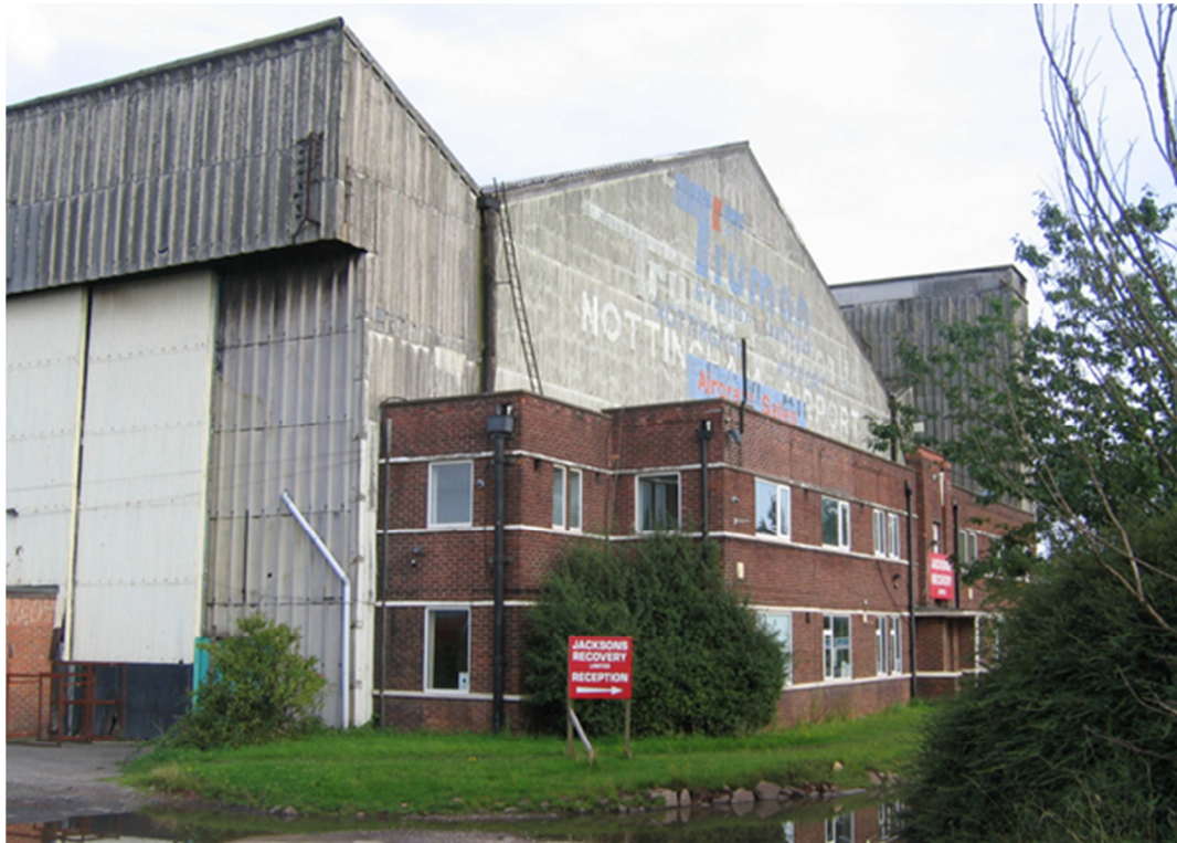
Figure 5: To the left of the rainwater pipe a slightly raised portion of cladding indicates the position of the door that was used by the fire watchers to gain access to the roof. [Milan Petrovic 07-08-2009]
