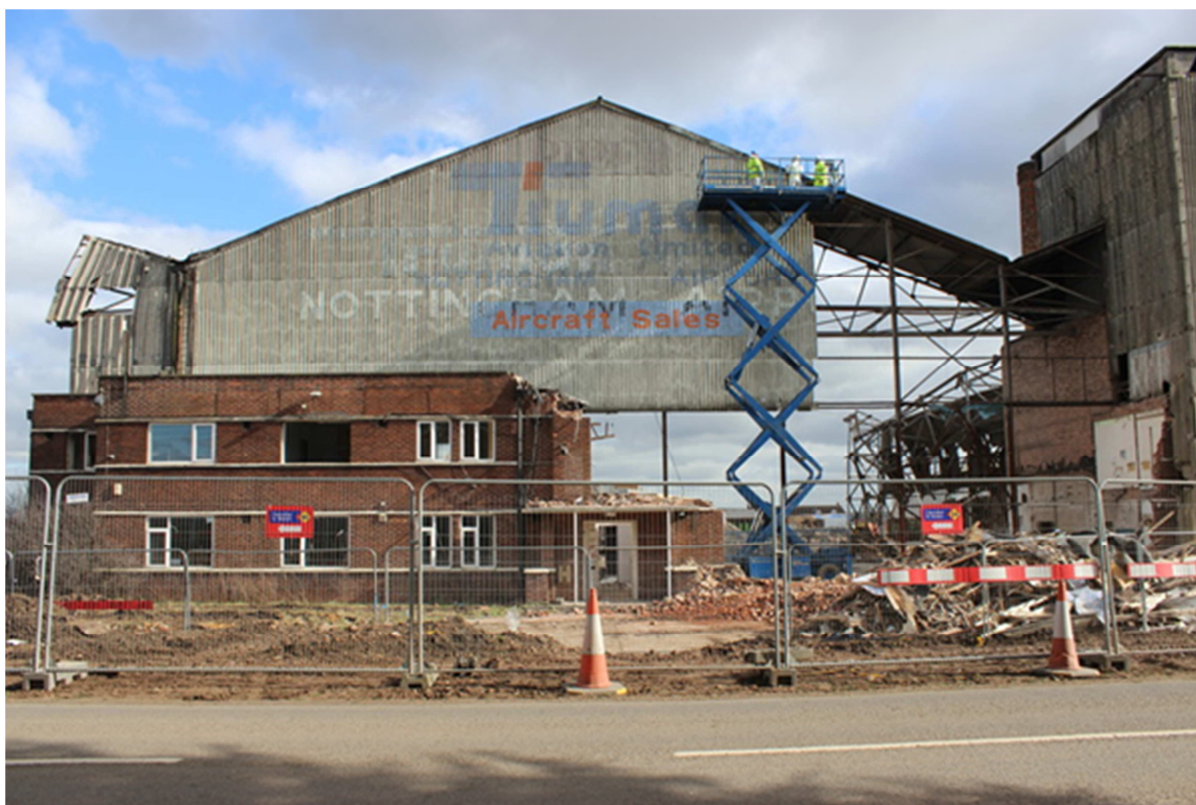
Figure 4: Main hangar during demolition. [Milan Petrovic February 2017]
