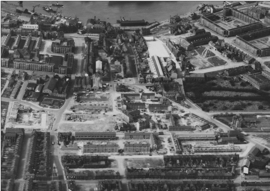
Fig 27: The first phase of post-war development in the East End under construction in 1958. RAF /58/2425 PSFO-0107 23-APR-1958 Historic England Archive RAF Photography (detail).
