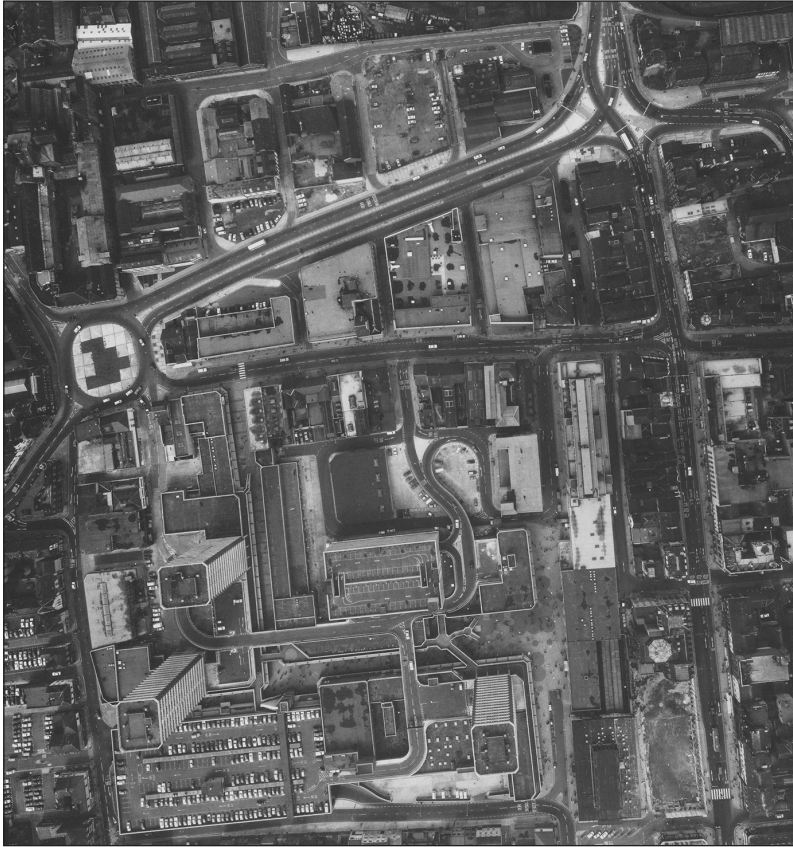
Fig 35: The completed Town Central Area development in 1971 including the new A138 dual carriageway. MAL/71025 V 042 17-APR-1971. © Sunderland City Council (detail).
