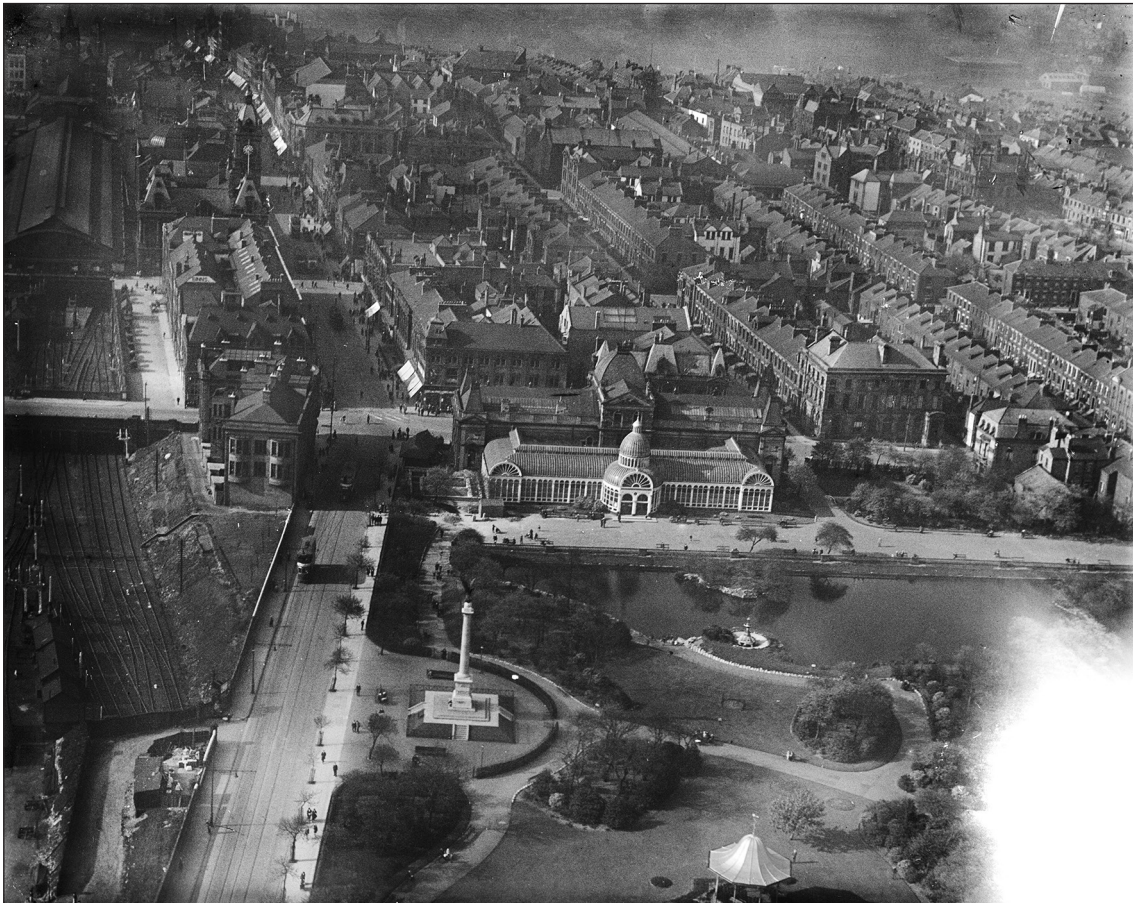
Fig 2: An Aerofilms Ltd photograph from April 1924 of the museum and library looking towards the railway station. © Historic England Archive. Aerofilms Collection EPW010379.
