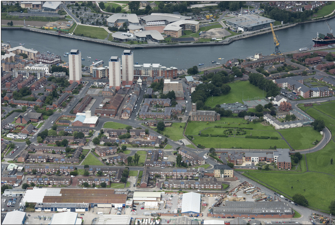
Fig 28: The area of the 1958-9 development photographed in 2017. Although retaining the same plan, the housing has now been replaced with two-storey terraces. 28946_064 04-AUG-2017 © Historic England Archive.
