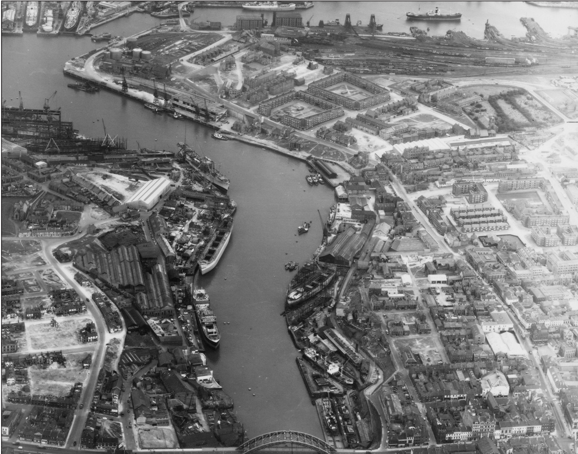
Fig 37: View looking east along the Wear. RAF /58/2425 PSFO-0085 23-APR-1958 Historic England Archive RAF Photography (detail).
