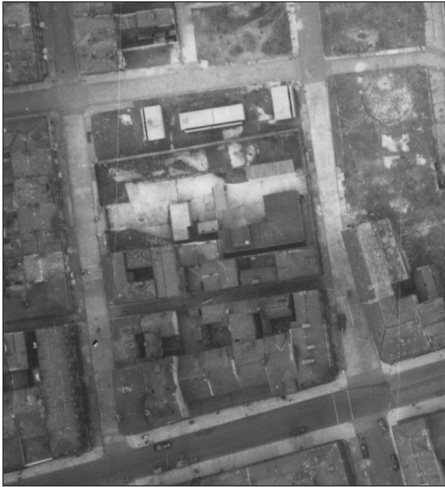
Fig 14: Communal surface shelters on Charles Street visible as flat-roofed rectangular structures with a long blast wall. The circular scar in the top right hand of the photograph is the former site of an Emergency Water Supply. RAF/106G/UK/873 RV 6223 01-OCT-1945 Historic England Archive RAF Photography (detail).
