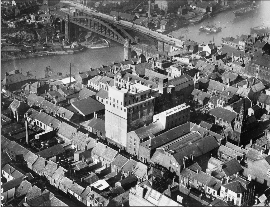
Fig 4: An Aerofilms Ltd photograph from April 1924 of Robsons Flour Mills looking north-east towards the Wearmouth Bridge. © Historic England Archive. Aerofilms Collection EPW0103760
