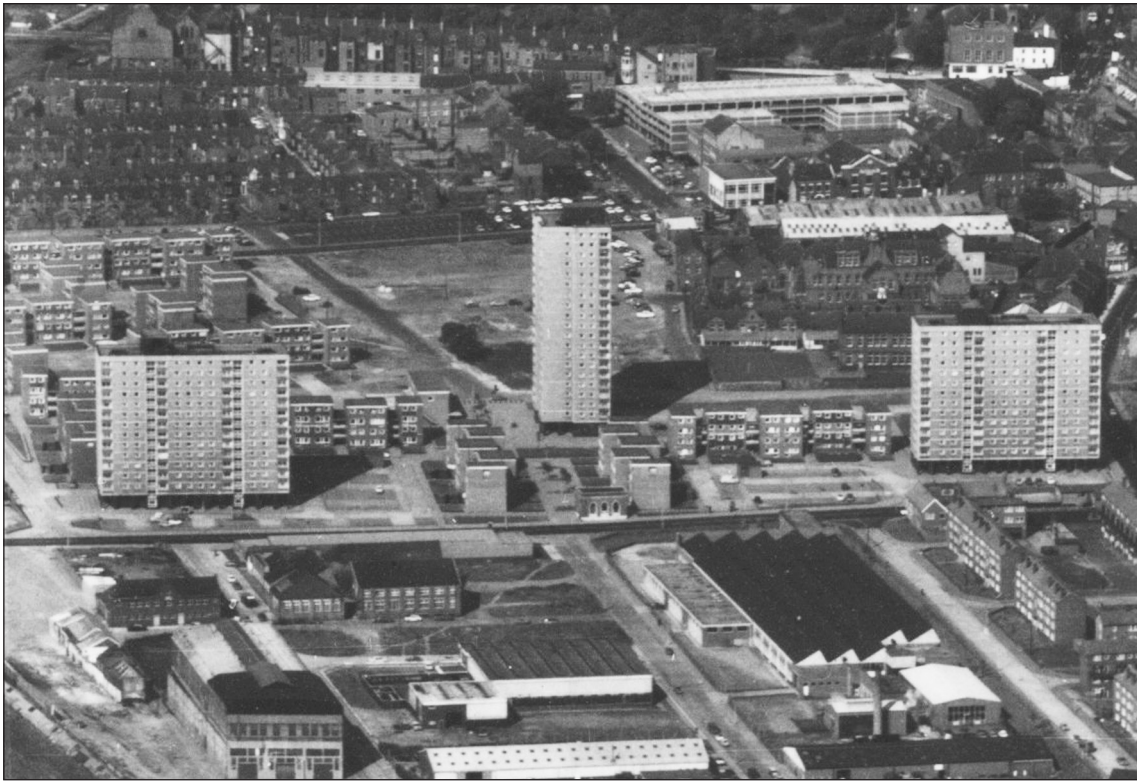
Fig 30: The Hendon Road development in 1970. The multi-storey towers are the only surviving elements of the scheme. RAF /58/0582 PO-0008 22-JUN-1970 ©Crown Copyright. MoD (detail).
