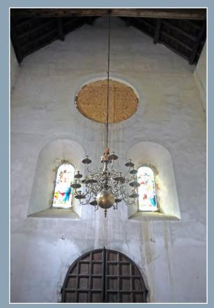
Water ingress and the damaged stained glass window
