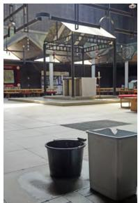
Minor leaks in the roof affecting the interior of the church
