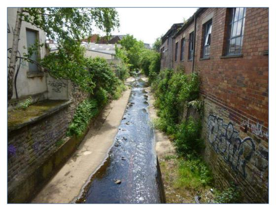
Plate 38:Section of the Porter showing extent of canalisationDeculverting and Decanalising
