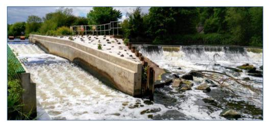
Plate 35: Sprotbrough Weir fish and eel pass
