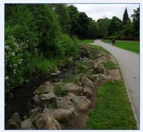
Plate 46: Millhouses Park fish bypass channel
