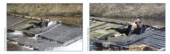
Plates 29-30: Illustration of the damage at Ward End Weir
