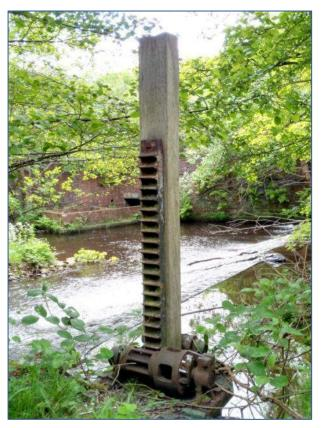
**Plate 7:** Ratchet and pinion shuttle mechanism in place at the entrance to the leat above the weir at Storrs Bridge on the Loxley.
