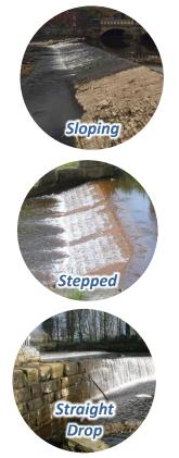
A weir with downstream, and often upstream, glacis – reduces water turbulence from undermining the foundation through reducing scouring action and buttresses the weir increasing stability. The slope may be parabolic to reduce hydraulic jump.
