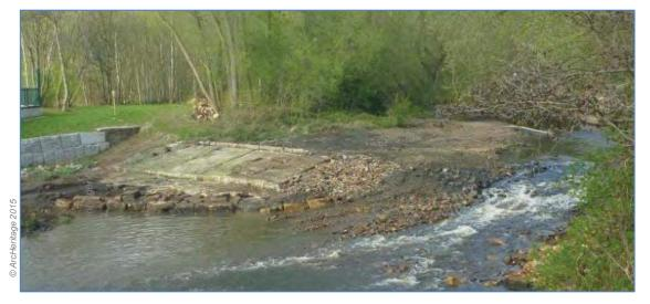
Plates 31: Ward End Weir following partial removal
