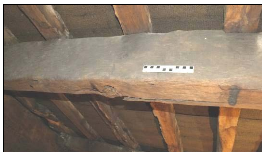
Fig 35: Taper burn marks on purlin on the east side of Bay 2 (© Historic England, photograph: Dan Elsworth)
