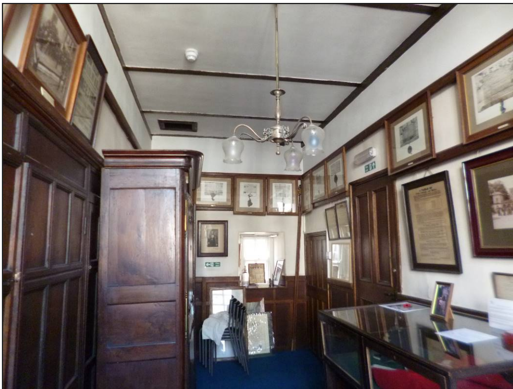
Fig 23: mayor's parlour from the east with re-set panelling to left and an inserted doorway to right (© Historic England, photograph: Marion Barter)
