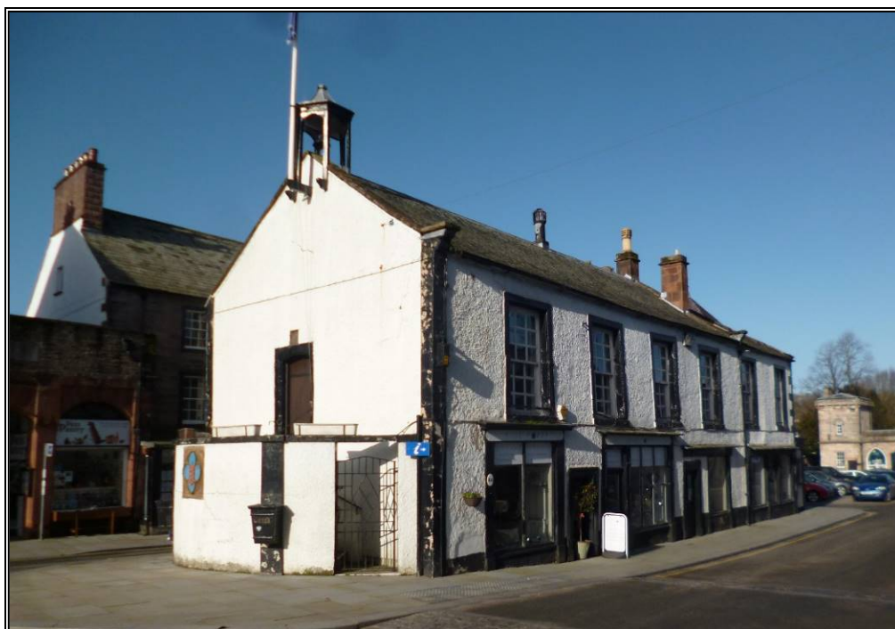
Fig 11: The south and east elevations with the principal 4-bay range to left and later north range to right (© Historic England, photograph: Marion Barter)
