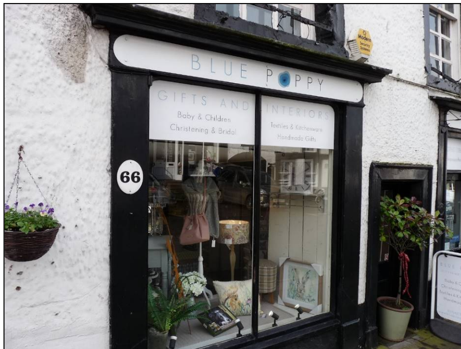
Fig 13: late 19th century shopfront with earlier doorway to right (© Historic England, photograph: Marion Barter)
