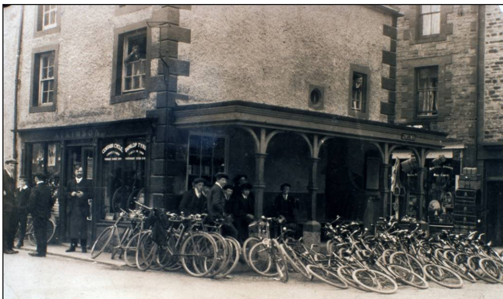
Fig 10: Atkinson's cycle shop and the shelter, built in 1911, in an undated view from the north-east (Appleby-in-Westmorland Society)
