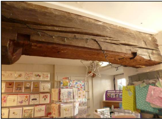
Fig 17: south beam in Number 66, altered for a doorway, from the south (© Historic England, photograph: Marion Barter)
