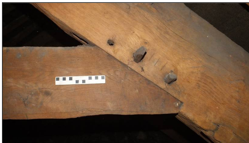
Fig 40: Assembly marks at the west end of Truss 3, viewed from the north (© Historic England, photograph: Dan Elsworth)
