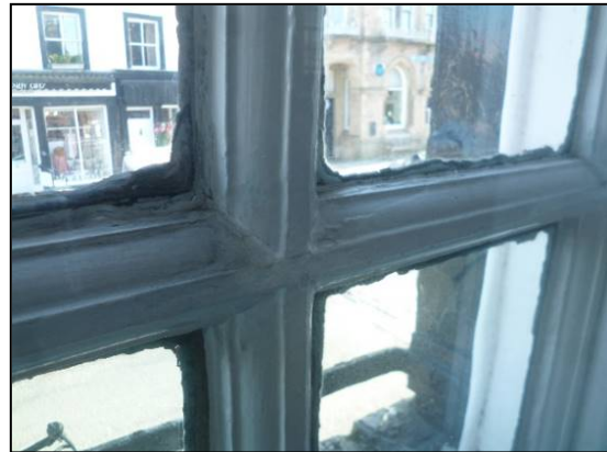
Fig.15: detail of ovolo-moulded glazing bars (© Historic England, photograph: Marion Barter)
