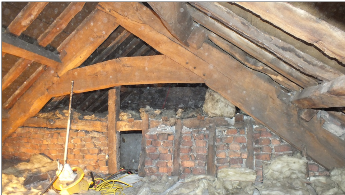
Fig 30: The south face of Truss 1, showing the timber stud partition with brick infill (© Historic England, photograph: Dan Elsworth)
