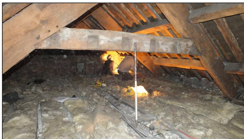
Fig 41: The re-used collar of Truss 3, viewed from the south-west (© Historic England, photograph: Dan Elsworth)
