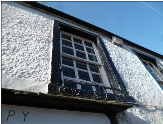
Fig 14: sash windows to Council Chamber (© Historic England, photograph: Marion Barter)
