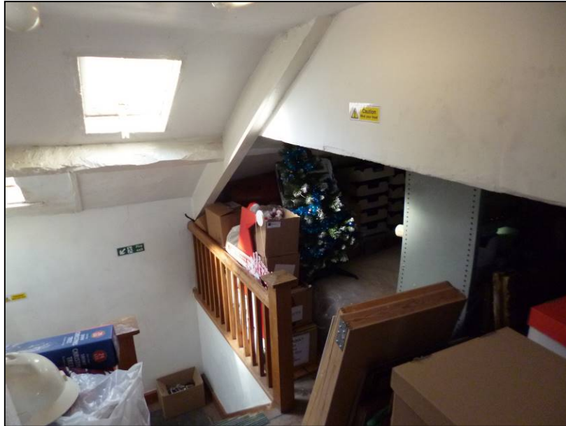
Fig 56: second floor store in the north range, from the east (© Historic England, photograph: Marion Barter)
