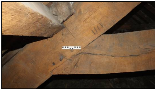
Fig 43: Carpenter's marks at the east end of Truss 4, viewed from the north (© Historic England, photograph: Dan Elsworth)
