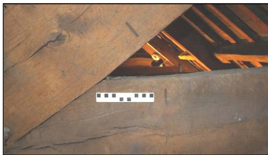
Fig 27: Carpenter's marks on east side of Truss 1, from the north (© Historic England, photograph: Dan Elsworth)
