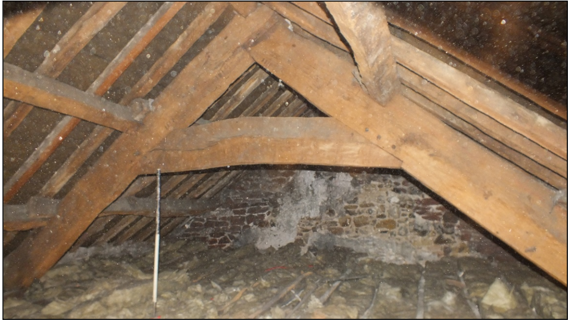
Fig 42: Truss 4, viewed from the north-west (© Historic England, photograph: Dan Elsworth)
