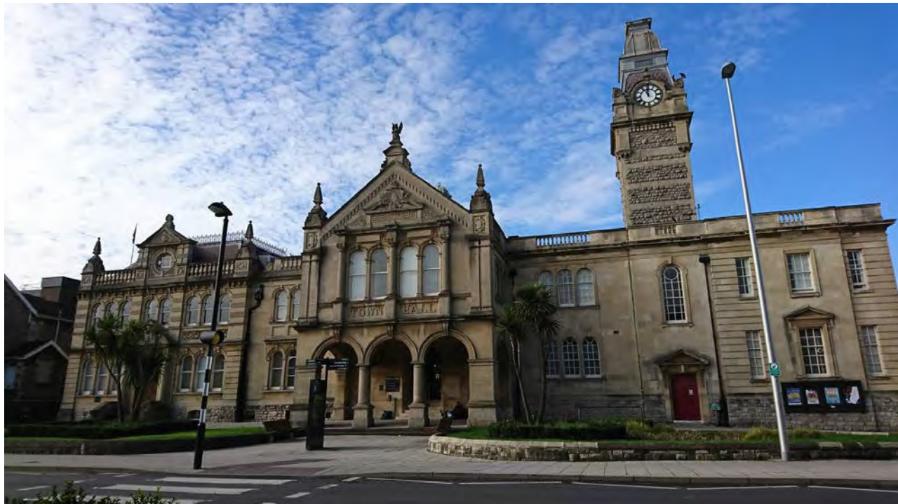
Photograph 1: Weston Town Hall frontage
