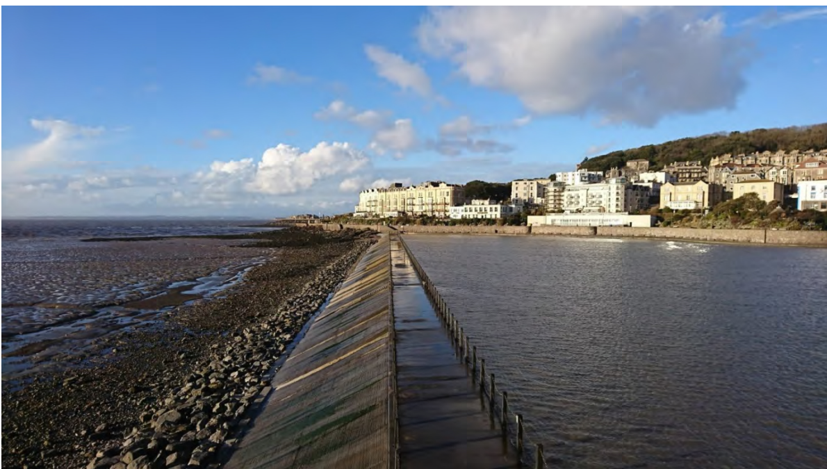
Photograph 2: Marine Lake retaining structure
