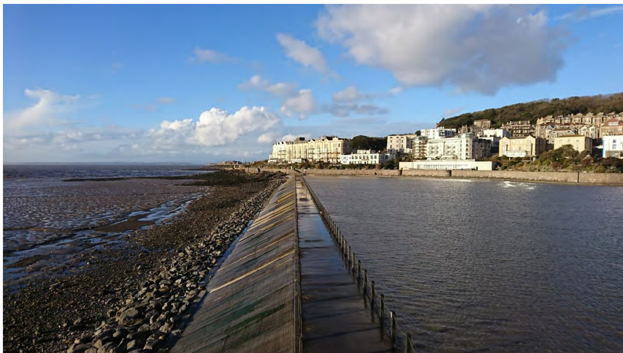
Photograph 2: Marine Lake retaining structure
