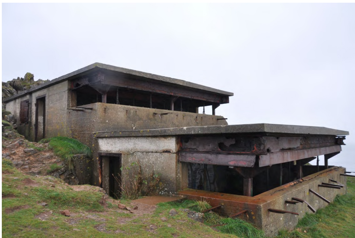
Photograph 1: Brean Down Fort – WWII Observation Post, showing recent reinforcement scaffolding
