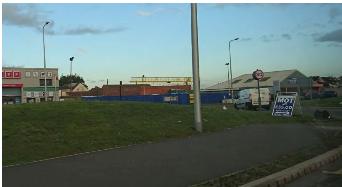
Photograph 1: Former Royal Potteries kiln building (brick structure in centre ground), Winterstoke Road
