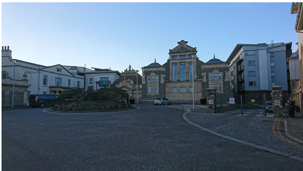
Photograph 2: The former Knightstone Baths, now flats, showing later purpose-built flat block inserted into the historic complex
