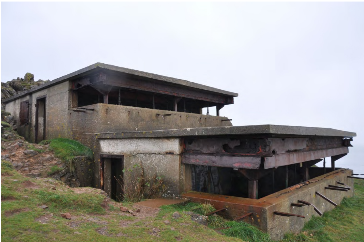
Photograph 2: Brean Down Fort – WWII Observation Post, showing recent reinforcement scaffolding
