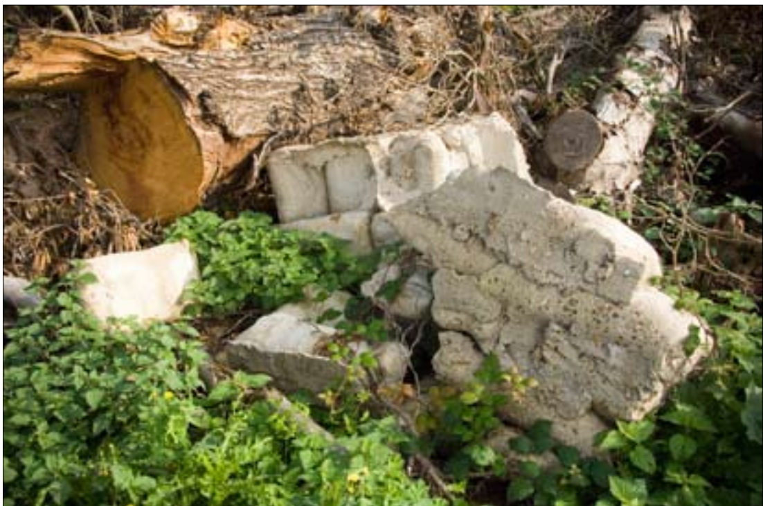
Remains of Light Anti-Aircraft Post, showing construction of cement-filled sandbags.
