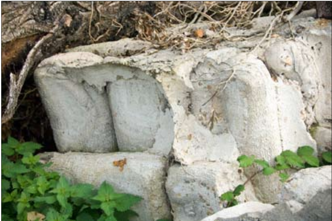
Remains of Light Anti-Aircraft Post, showing detail of sandbags.
