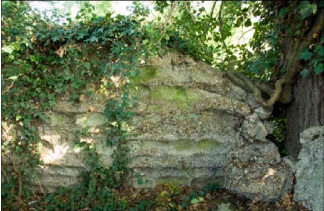
Gun Post, interior of east wall.
