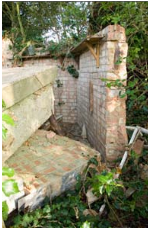
Battery Observation Post from the north west (detail).
