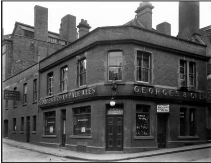
The Cat and Wheel, Castle Green, a city centre corner pub of 1900 by Thomas Scammell, had a window display of this type, showing the side on which off sales could be purchased © Hartley Collection, Bristol Museum
