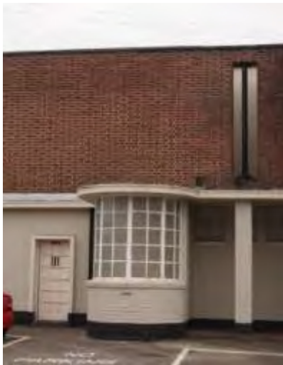
The remains of the 'Off Licence' at the Merchants Arms, Bell Hill, Stapleton. Architects: R. C. James and H. E. Meredith for The Bristol Brewery Georges and Company, Limited. Fiona Fisher and Rebecca Preston, 2014
