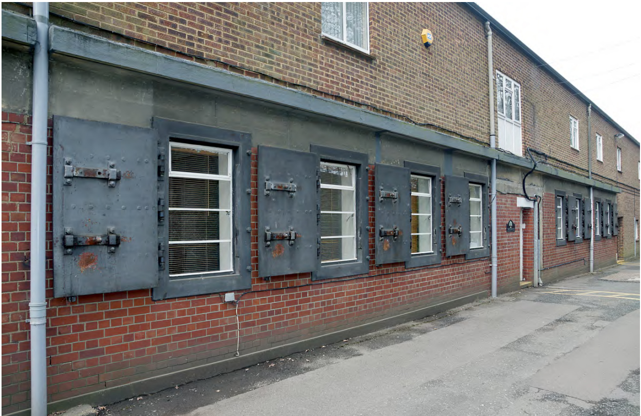
Plate 19: The dispersed 'Whitegates', Shenfield LNER New Office Building
