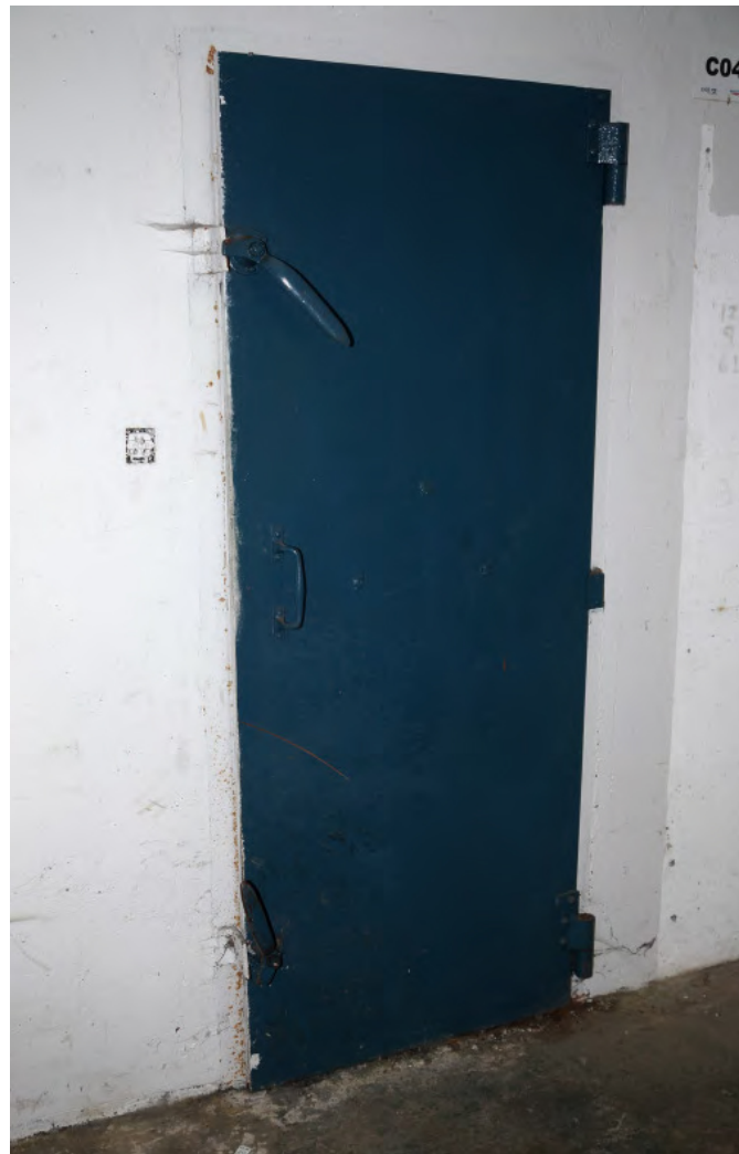
Plate 28: Type S.2 splinter-proof door
