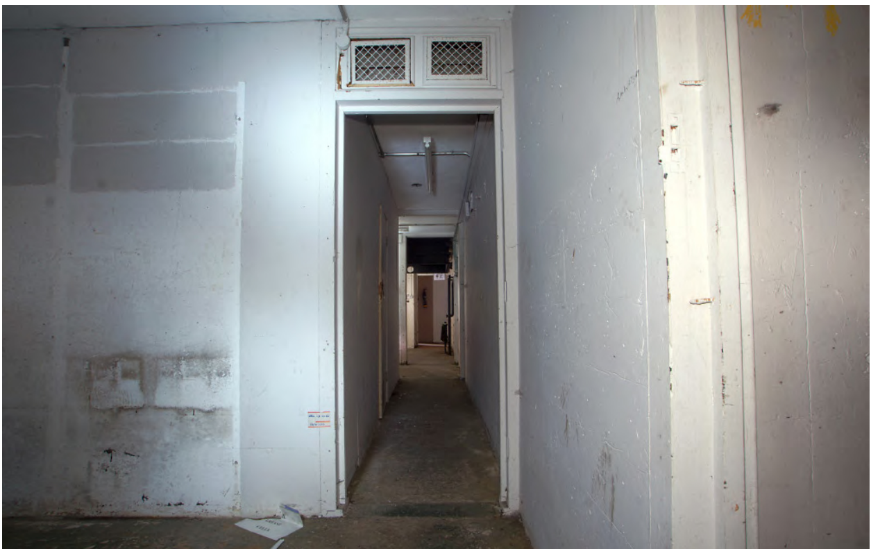
Plate 27: View from exit air-lock along 'new' corridor
