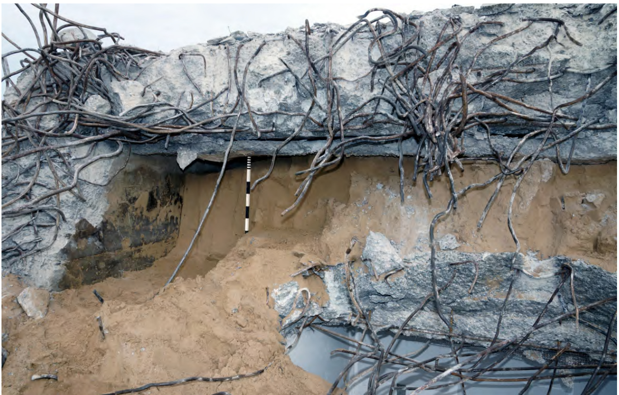
Plate 52: The emergency exit air-lock which can be seen below right
