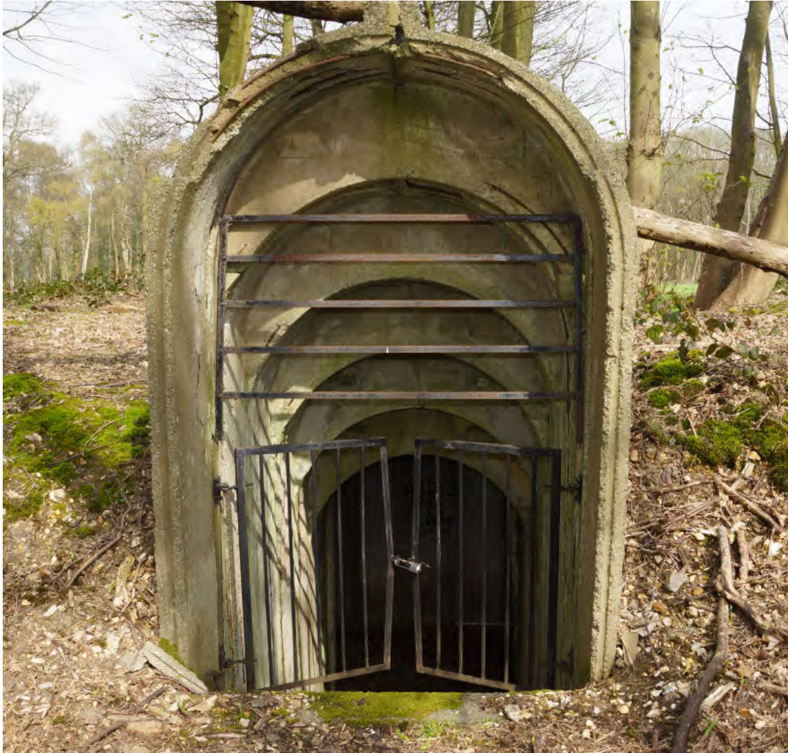
Plate 8: One of several entrances to the air-raid complex at The Grove, Watford
