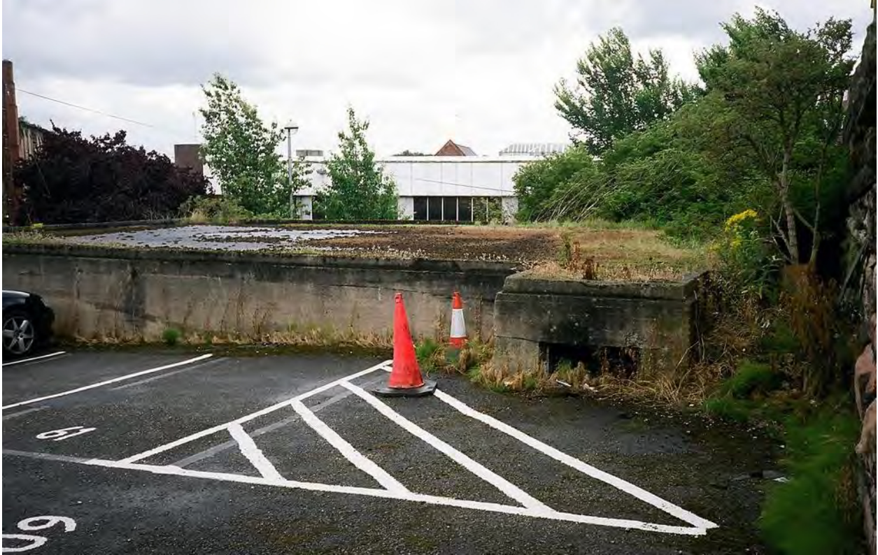
Plate 10: The Carlisle District Control Room
