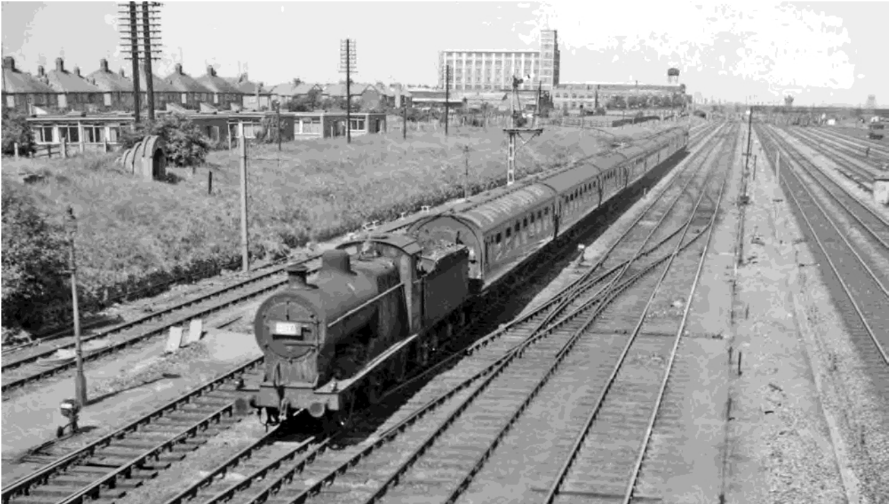
Plate 7: View from Spital Bridge, Peterborough showing a monolithic concrete LMS style air-raid shelter entrance The entrance on the left embankment was one of two to a semi-underground air-raid shelter which was 76 ft long. Photo: Dr. BWL Brooksbank
