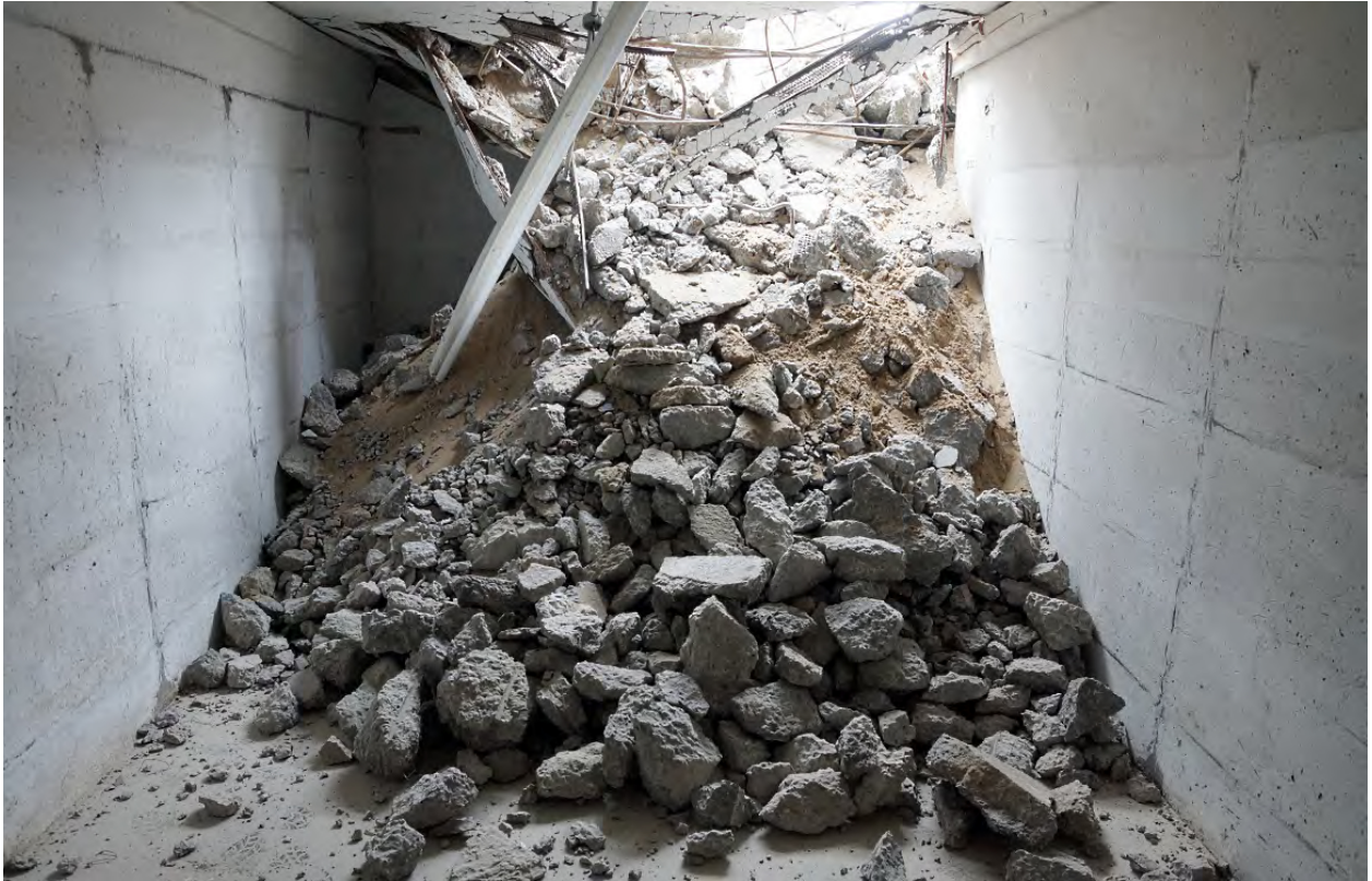
Plate 55: A last look at the control room
