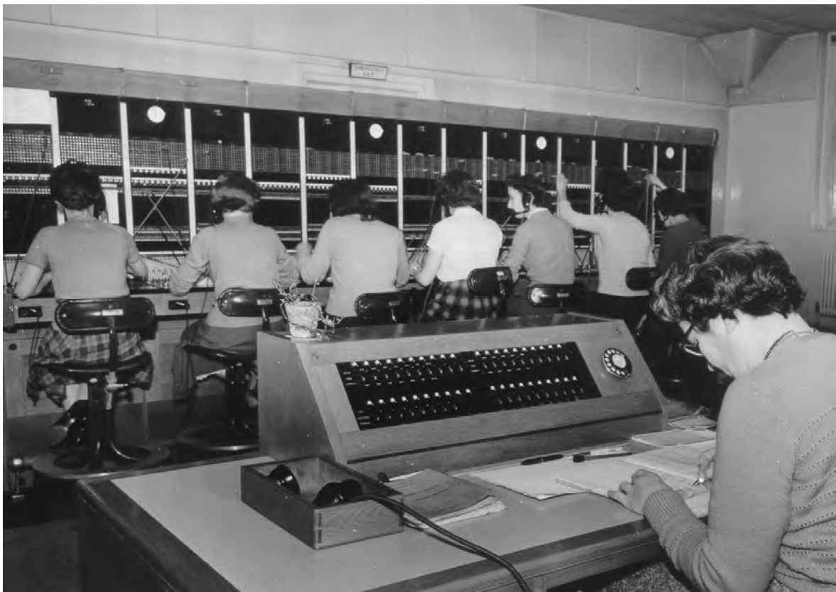
Plate 2: Crewe telephone switchboard and supervisor's desk. Photos: Bob Freshwater
