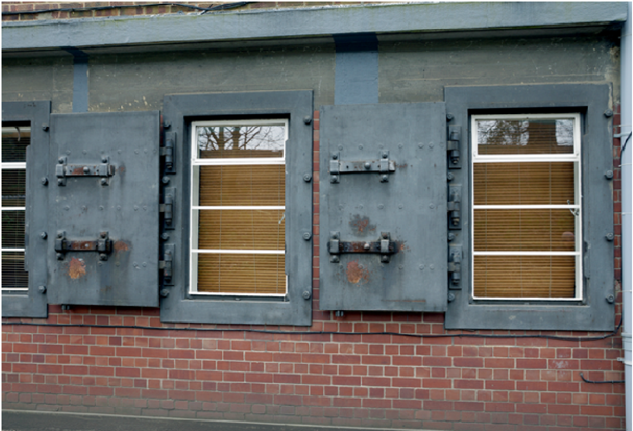
Plate 18: The dispersed 'Whitegates', Shenfield LNER New Office Building shutters open
