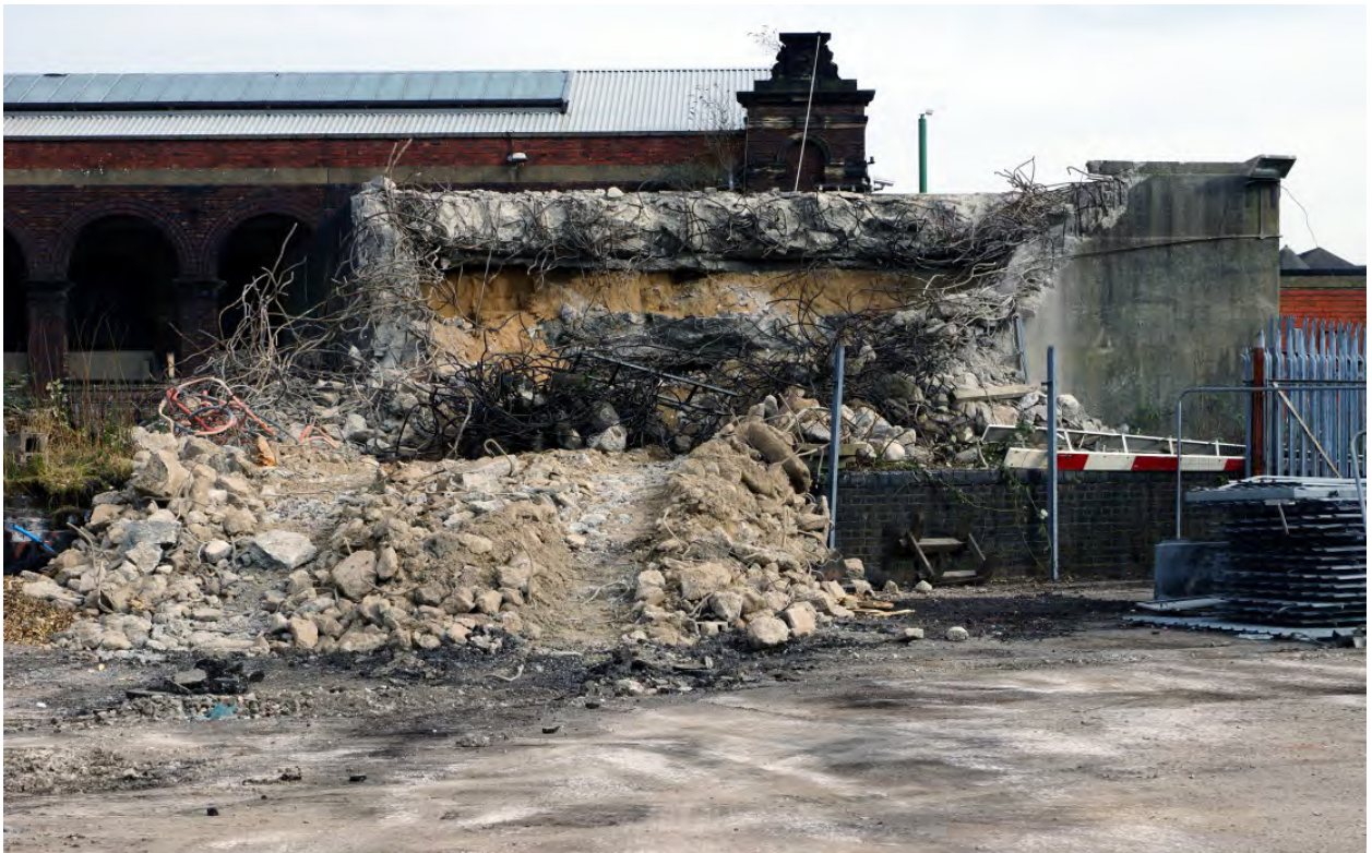
Plate 54: General view of the demolition site
