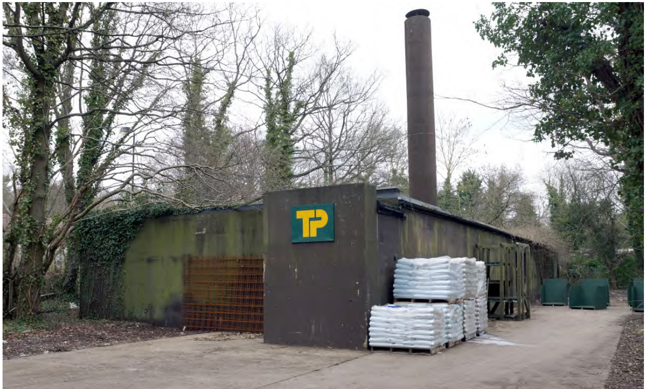
Plate 45: The Standard District Control Centre Type 'L' at Bricket Wood Now used as a store for Travis Perkins Ltd
