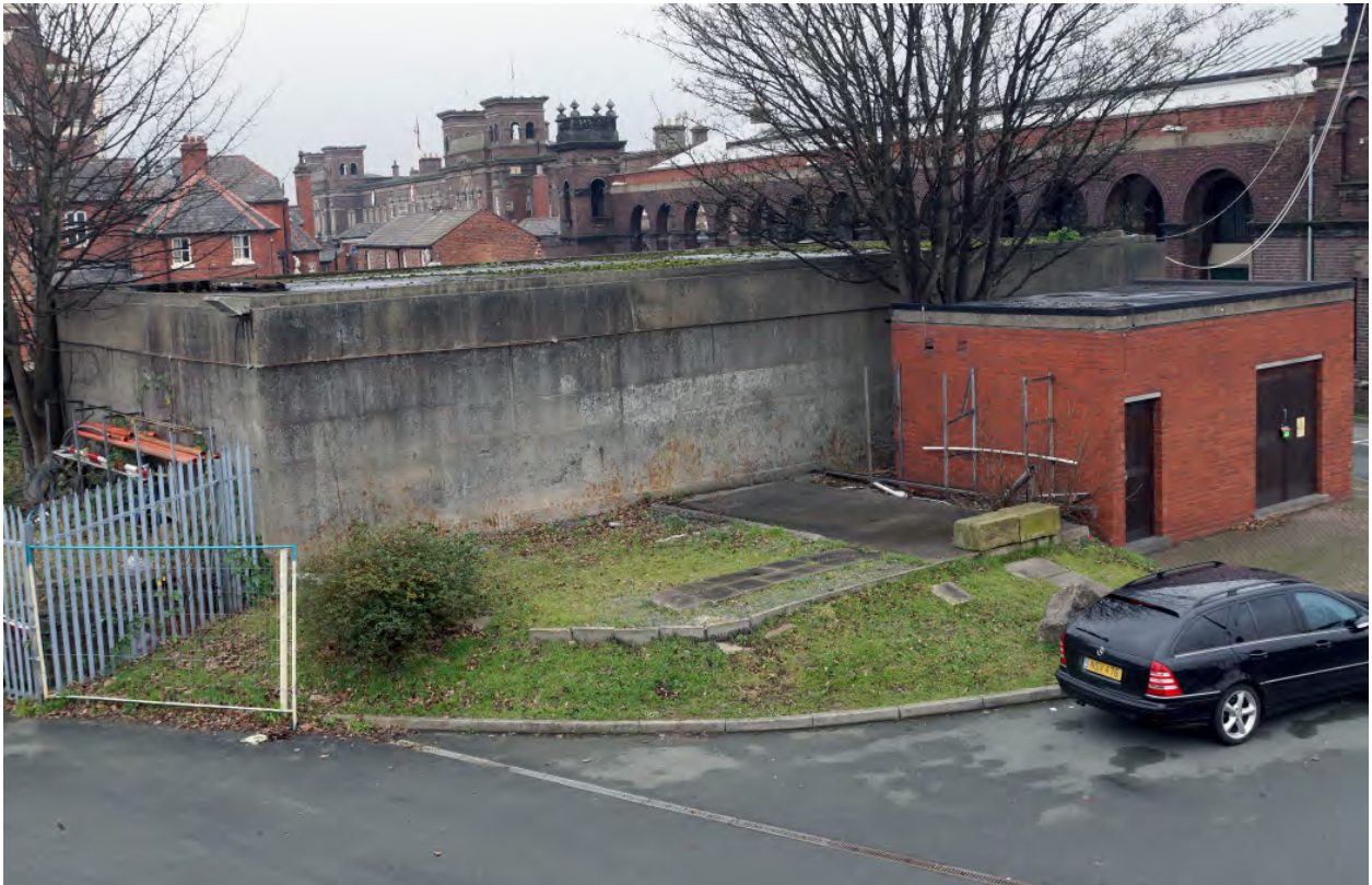
Plate 22: Distant view looking towards Chester Railway Station with the control room in the foreground There is a concrete slab adjacent to the modern electric sub-station of unknown function
