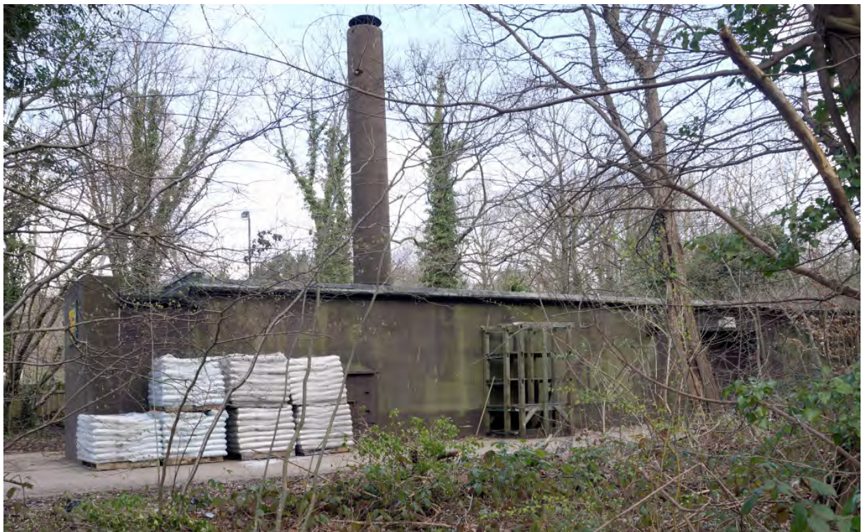
Plate 46: Bricket Wood – view looking towards the plant side elevation
