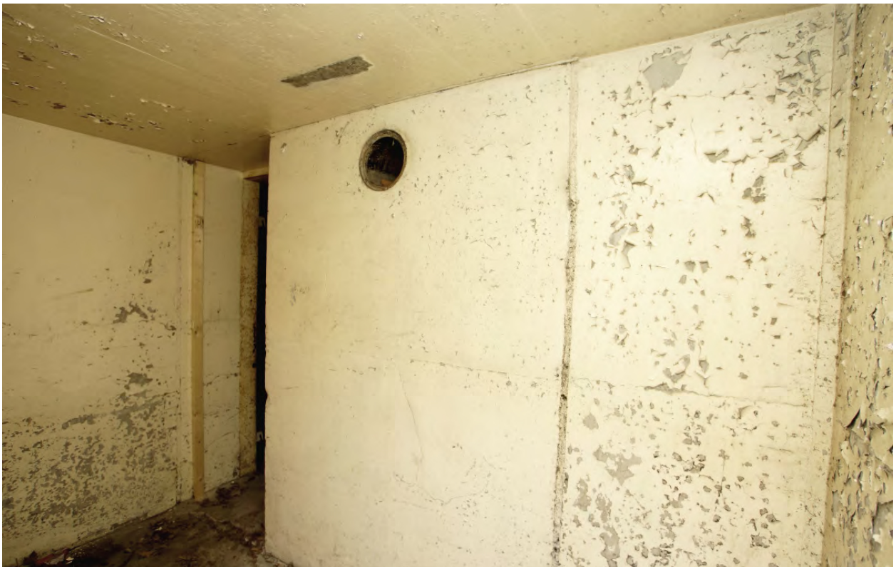
Plate 44: Main entrance baffle
