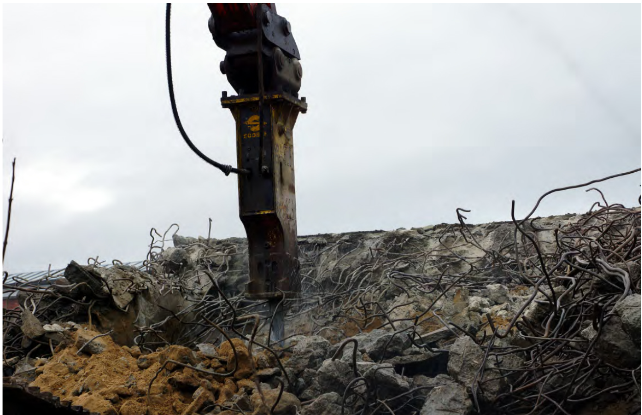
Plate 58: Hydraulic hammer in action
