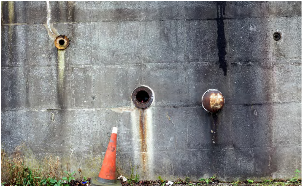
Plate 13: Type A1 Divisional Control Room, Crewe – services -
