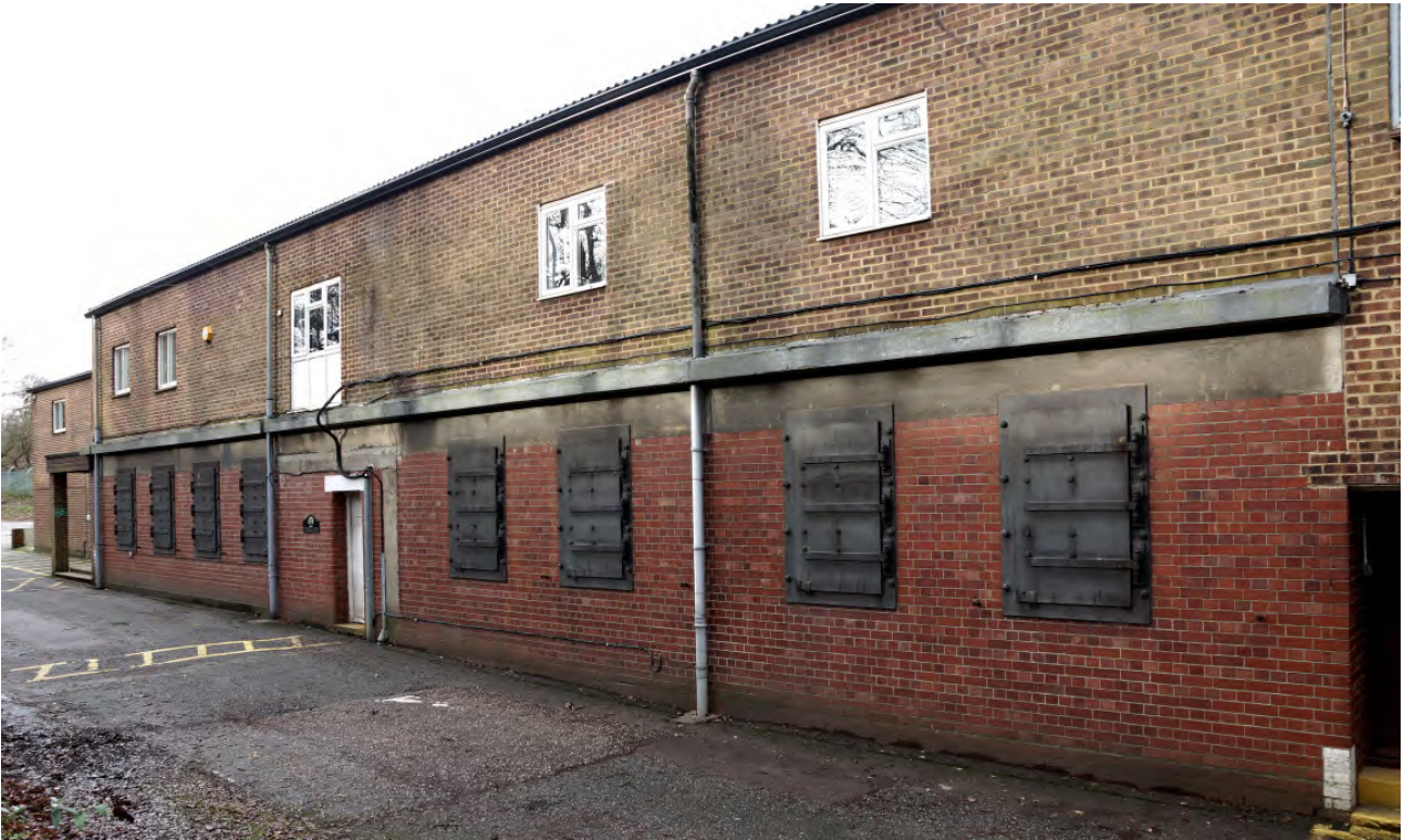
Plate 16: The dispersed 'Whitegates', Shenfield LNER New Office Building Now with additional floor but clearly showing the original single-storey building. It is unknown when the first floor was added or the end extensions but is presumably post Second World War
