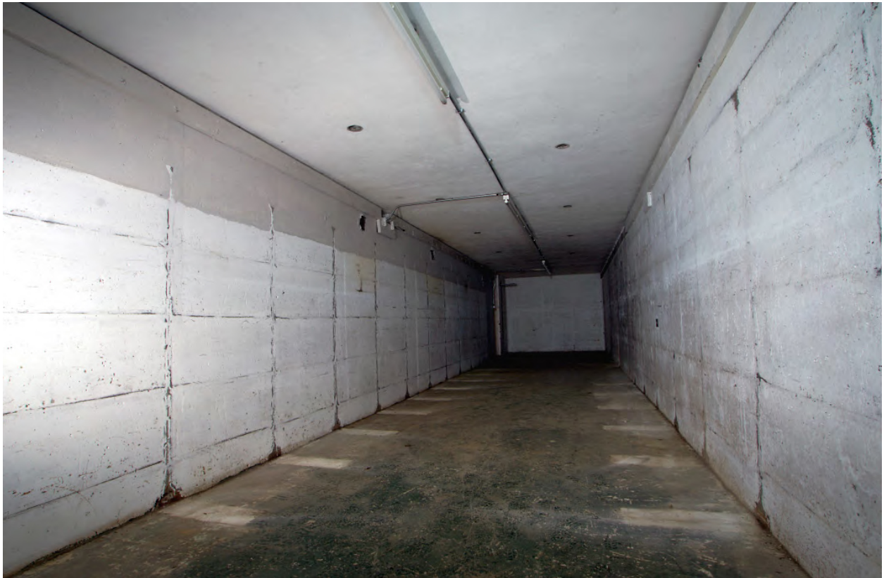
Plate 24: Interior of main room looking north towards the entrance
