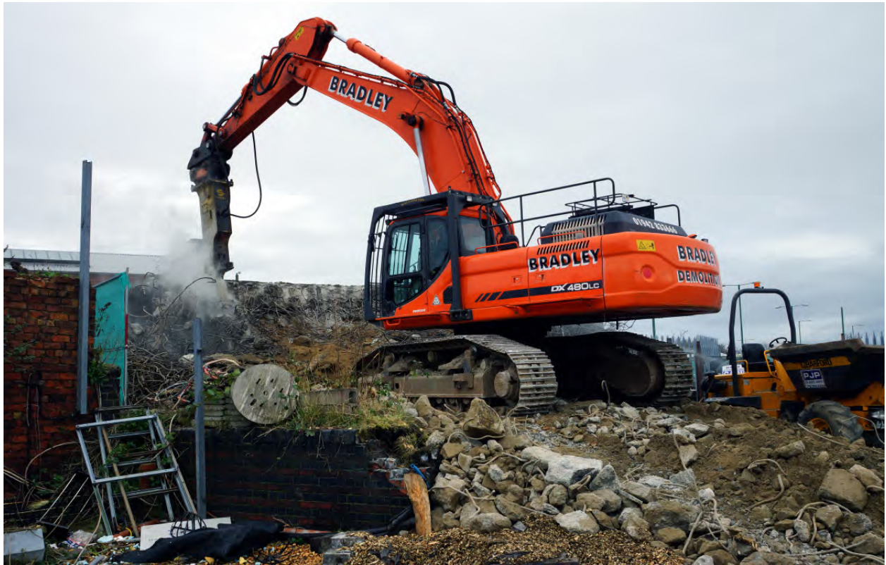
Plate 57: The demolition process
