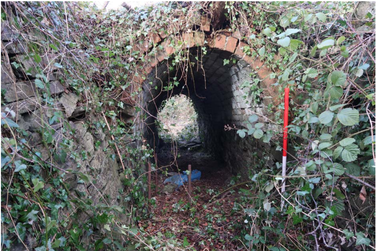
Fig 3: tunnel from pit (d) (foreground) looking north-west to chamber (e)
