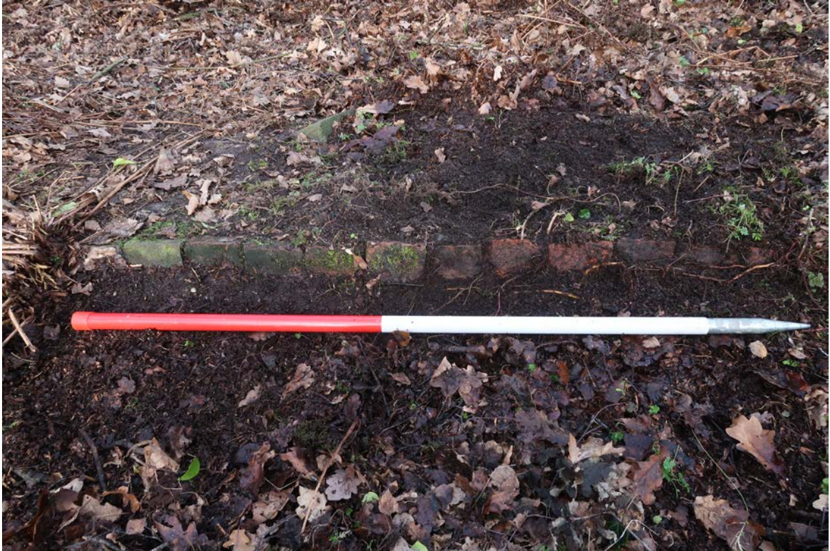
Fig 9: retaining wall along the northern side of pond 2
