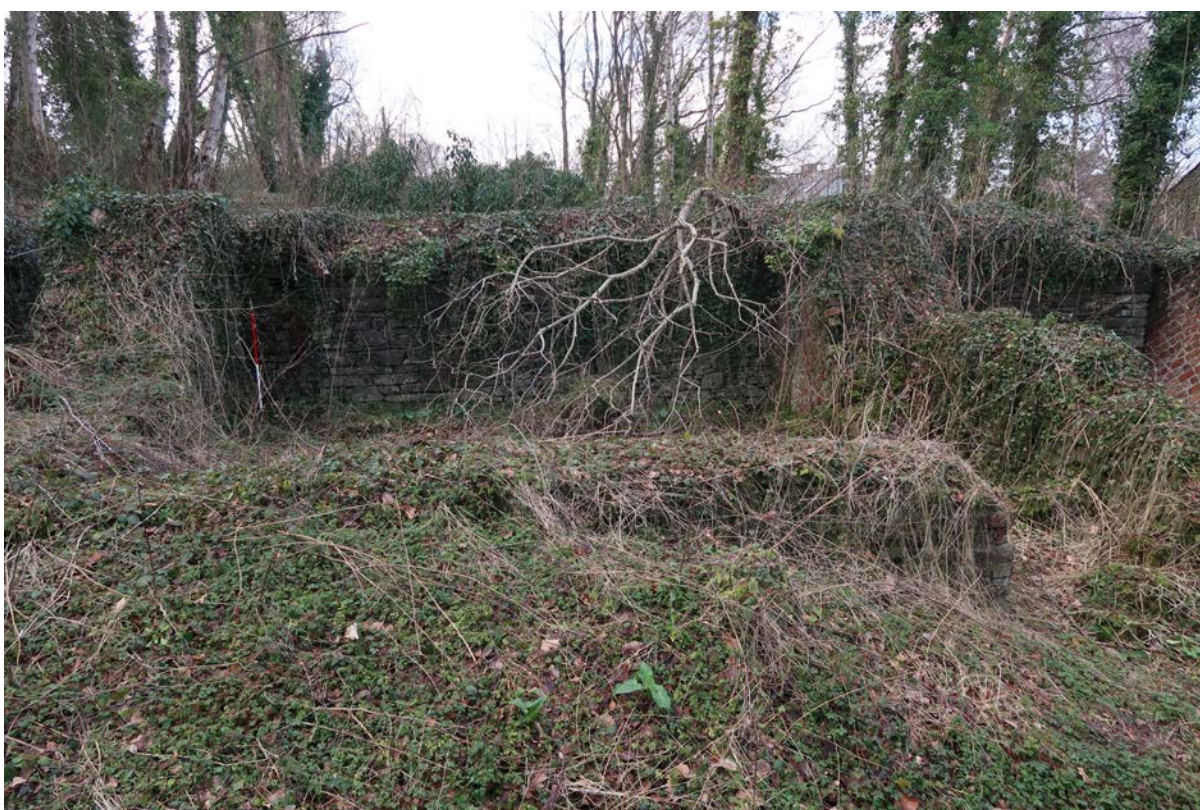
Fig 2: structure (c) at the north-east end of the smelt house, looking south-west
