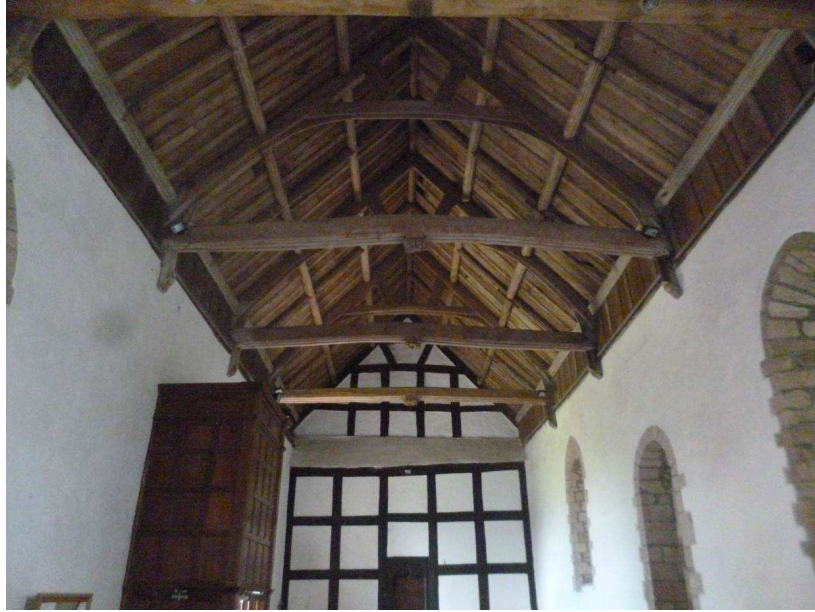
Figure 7: Nave roof with timber-framed partition at the west end, photograph taken from the east (Alison Arnold)
