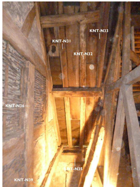
Figure 14: Portion of roof between nave and tower (south side), showing the location of samples KNT-N31–33, KNT-N35, KNT-N36, and KNT-N39
