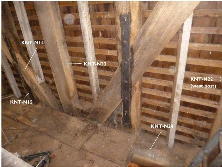
Figure 11: South wall of tower at bellframe level, showing the location of samples KNT-N14, KNT-N15, and KNT-N22–24
