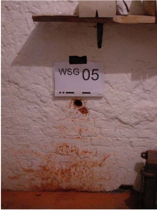
Figure 17: section of west-facing interior wall of engine room showing sampling location WSG-05
