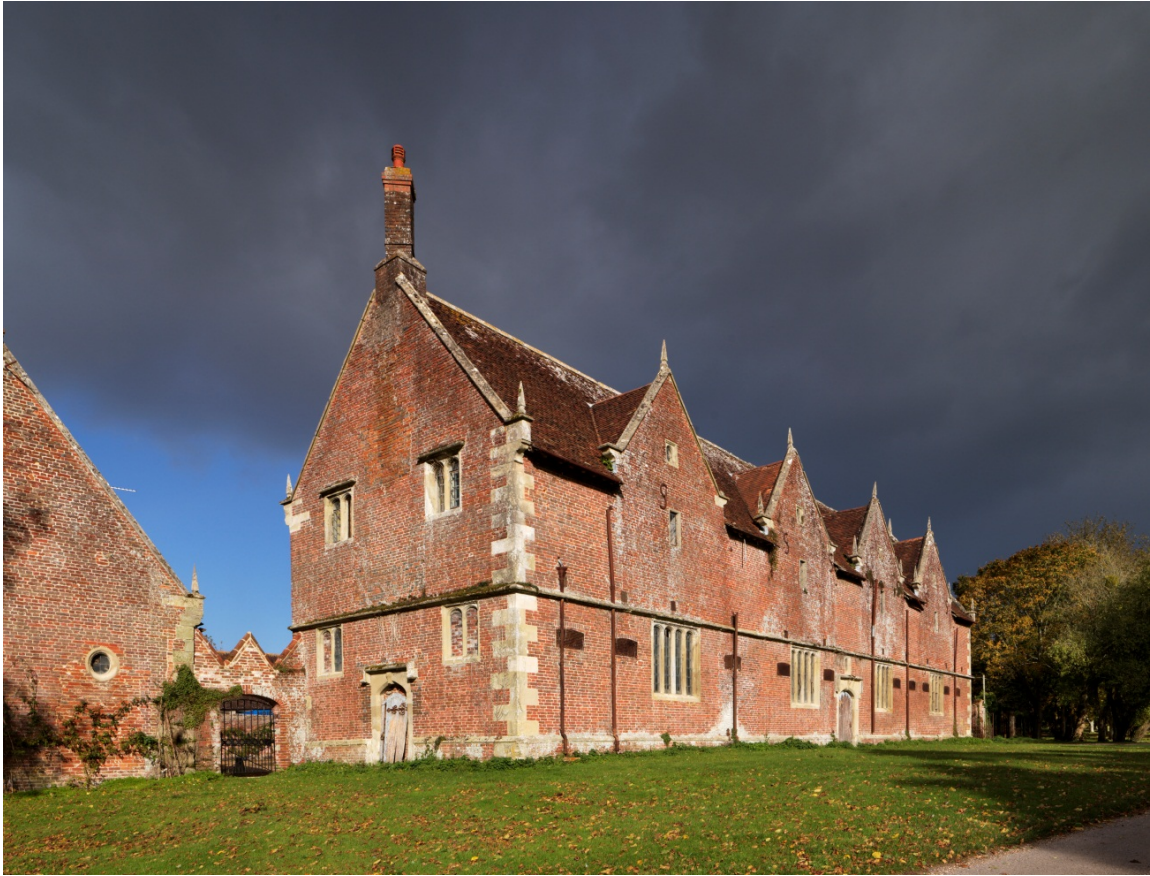
Figure 5: The 'Riding House' (© Historic England, DP166132; photograph by James Davies)
