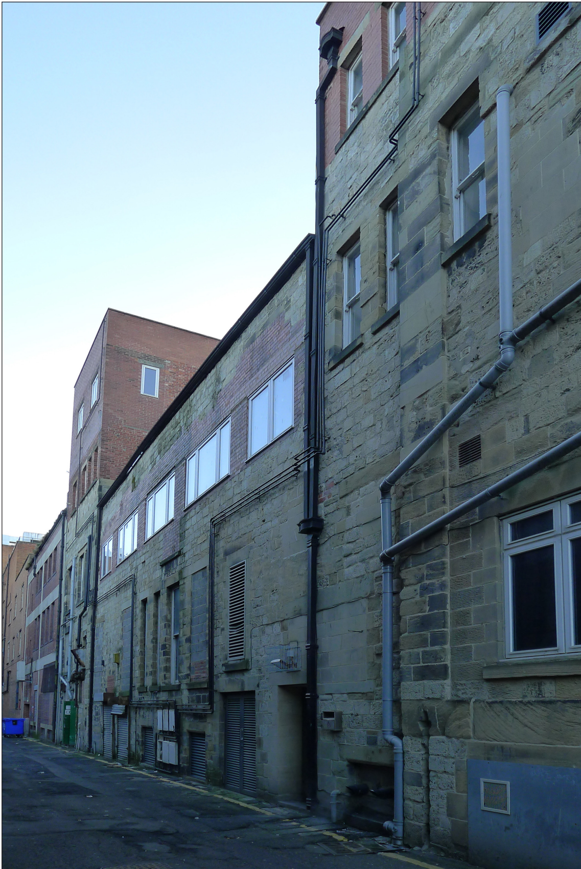
Fig 8: The eastern elevation, facing the rear alleyway. The red brick 'towers' are an addition of 1900, and the brickwork added to the wall of the billiard room may suggest that it was also refenestrated at this time (replacement windows have been recently inserted). © Historic England / Lucy Jessop.
