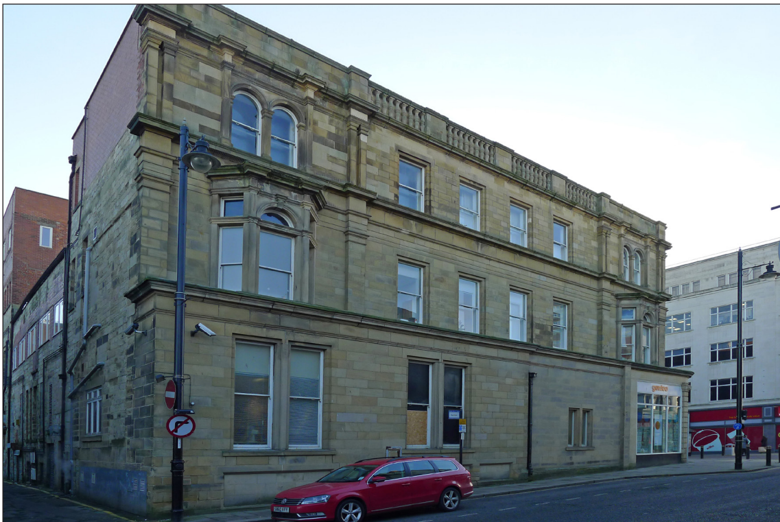
Fig 5: The Athenaeum Street elevation of Athenaeum Buildings. © Historic England / Lucy Jessop.
