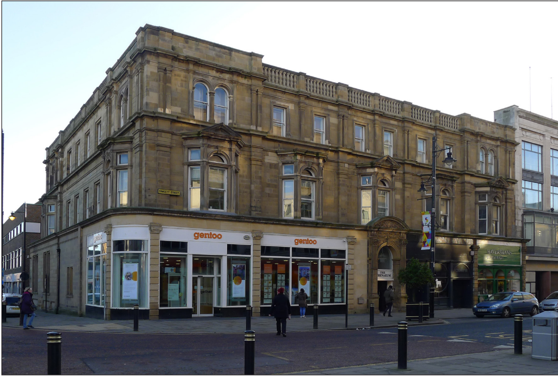
Fig 4: The Fawcett Street elevation of Athenaeum Buildings. © Historic England / Lucy Jessop.
