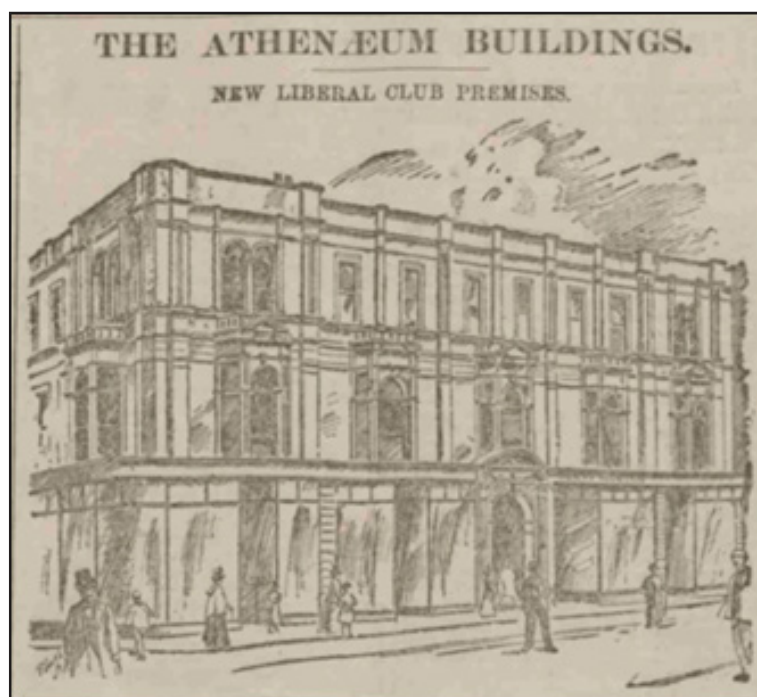
Fig 6: Illustration showing the rebuilt Athenaeum Buildings from the Sunderland Daily Echo , 25 August 1900, p3. © www.britishnewspaperarchive.co.uk.
