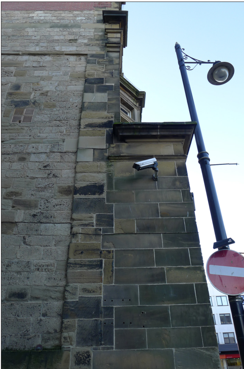
Fig 9: The corner of the alley and Athenaeum Street, showing the basic 1840s walling with the 1900 façade grafted onto it. © Historic England / Lucy Jessop.
