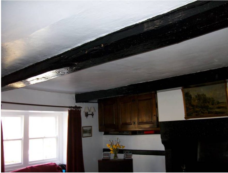
Figure 6c: First floor ceiling beams to Present Farmhouse (photograph Robert Howard)
