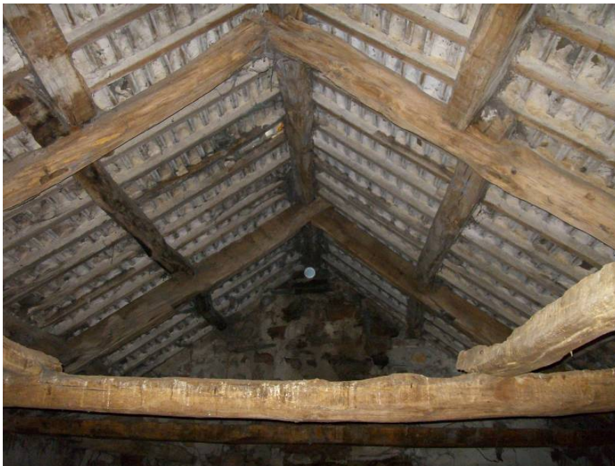
Figure 5c: View of the roof to the former farmhouse (photograph Robert Howard)
