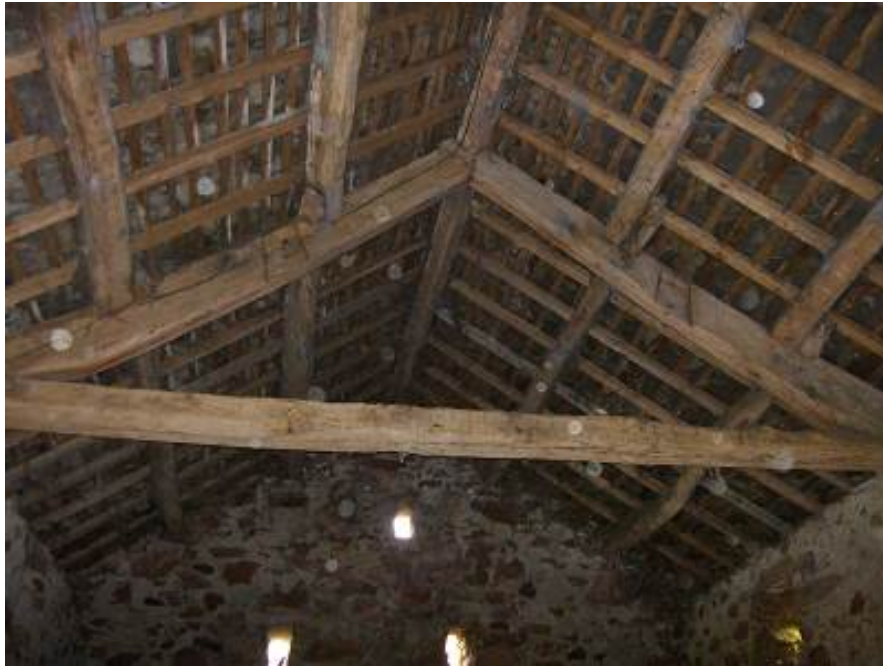
Figure 9b: The roof of the Back barn (photograph Robert Howard)
