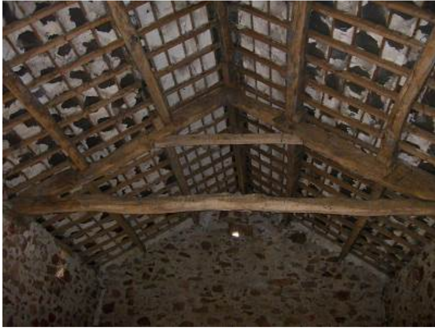
Figure 8b: The roof of High Leys barn (photograph Robert Howard)
