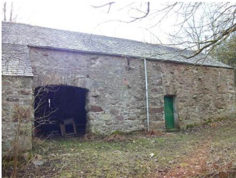
Figure 9a: The Back barn from the north (photograph Robert Howard)
