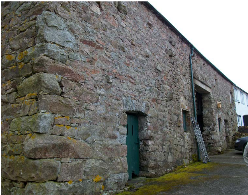
Figure 7a: View of the Garage barn (photograph Robert Howard)
