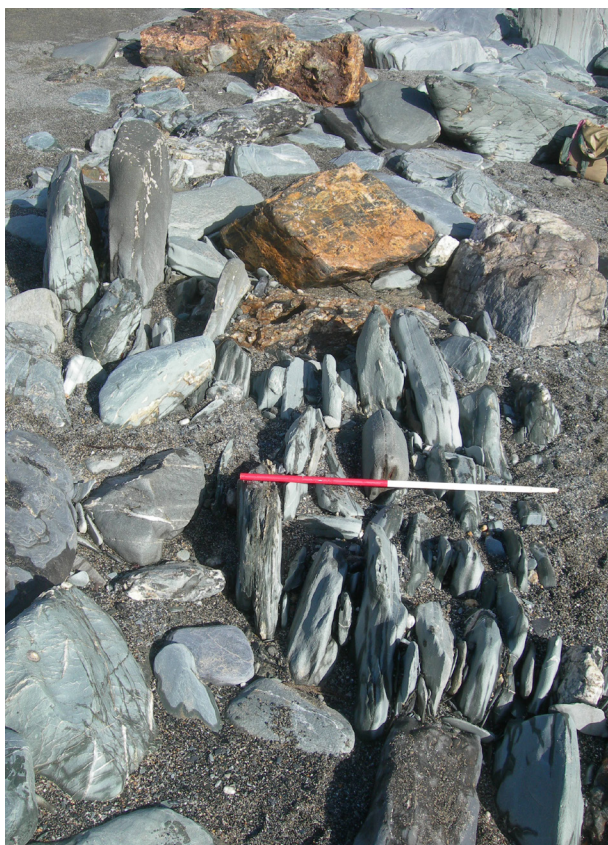
Figure 7: Detail of the vertically set and closely fitted packing stones between the two faces of the ruined quay; the remnants of the inner face being visible towards the top.
