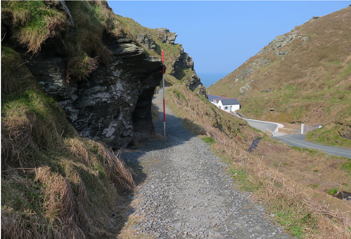
Figure 22: The lowest stretch of the zigzag track (A) was run to this rock outcrop, which was then chiselled to create a concave profile that allowed passage for laden packhorses but prevented easy movement for ridden horses.
