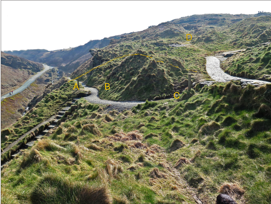
Figure 25: The highest stretch of the zigzag track looking south from the edge of the Great Ditch; the third and steepest stretch is marked by the steps on the left. Two later medieval cuts were made through the sweeping curve of the carefully engineered bend (whose top is indicated by a yellow line), the track to Borough Mill (right of A) and the cut-through (left of B) linking to the early medieval hollow-way (D). The barbican protecting the gate to the Lower Ward of the 13th-century castle was reached by a third cut (C). The nearer stretch of the track was effectively made redundant by this cut through at C and was itself later cut through by the extension of the Great Ditch to run alongside the barbican (Figures 26 and 27).
