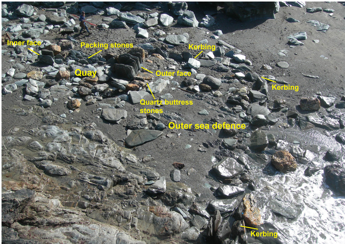
Figure 5: Details of the ruined quay viewed obliquely at low tide from the Black Rock peninsula, to its north-west. The person carrying the ranging pole and accompanied by a dog (top left) is passing the rounded south-eastern end, beyond the short surviving stretches of the inner and outer faces. Outer sea defences of set quartz blocks (buttress stones) and kerbed cobbled area are also visible.
