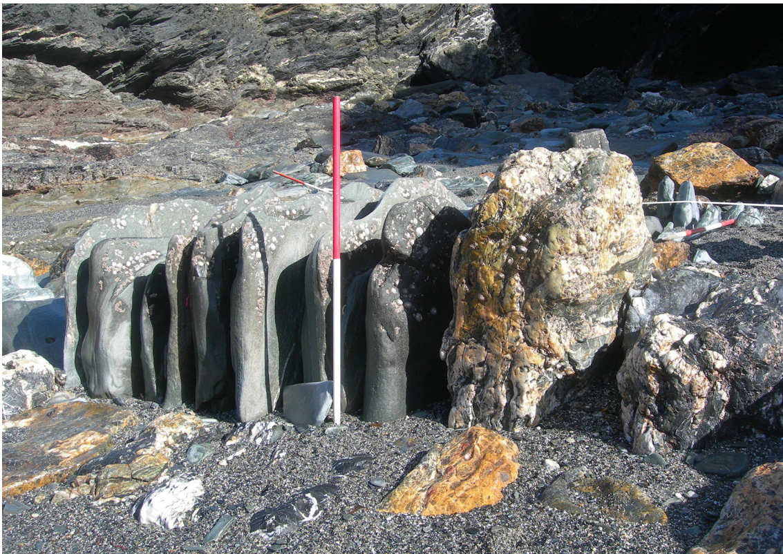
Figure 6: Surviving remains of outer face of quay, viewed from west. Ranging pole is 1m long. The tops of quartz blocks placed as a sea defence against the feet of the upright stones in the face are also visible.
