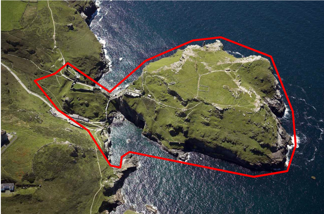
Figure 30: The Post-Roman port of trade at Tintagel comprised the Island (with scores of sub-rectangular structures), Haven, zigzag track, Great and Outer Ditches and the crag later reused for the Upper Ward of Tintagel Castle, as delineated in red in this aerial photo. (Photo by Steve Hartgroves, Cornwall and Scilly Historic Environment Record, F77-037, 8th August 2007; copyright reserved.)
