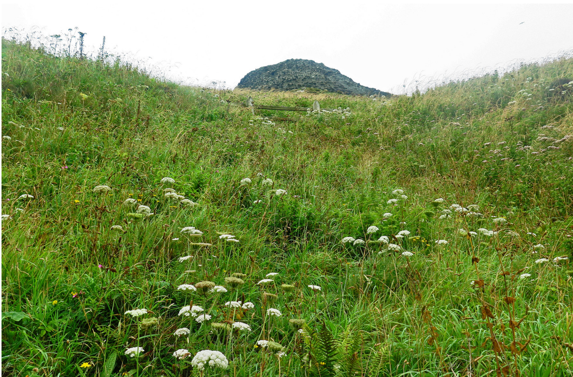
Figure 23: The outer ditch viewed from below, from the lowest stretch of the zigzag track. The fence indicates the upper end of the ditch, coinciding with the second stretch or zig of the track. Above is the stone walling of the Upper Ward of the 13th-century Tintagel Castle, set on a natural crag from which the lowest stretch of the zigzag track could be viewed via the ditch.
