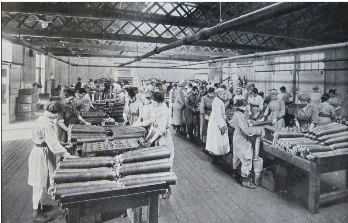
Fig. 4.21. NFF No. 1 Leeds (Barnbow). Interior view showing 18pdr assembly (undated). Note the single-storey wooden hut, Belfast Truss roof, and lack of blast protection (TNA MUN5/157).
