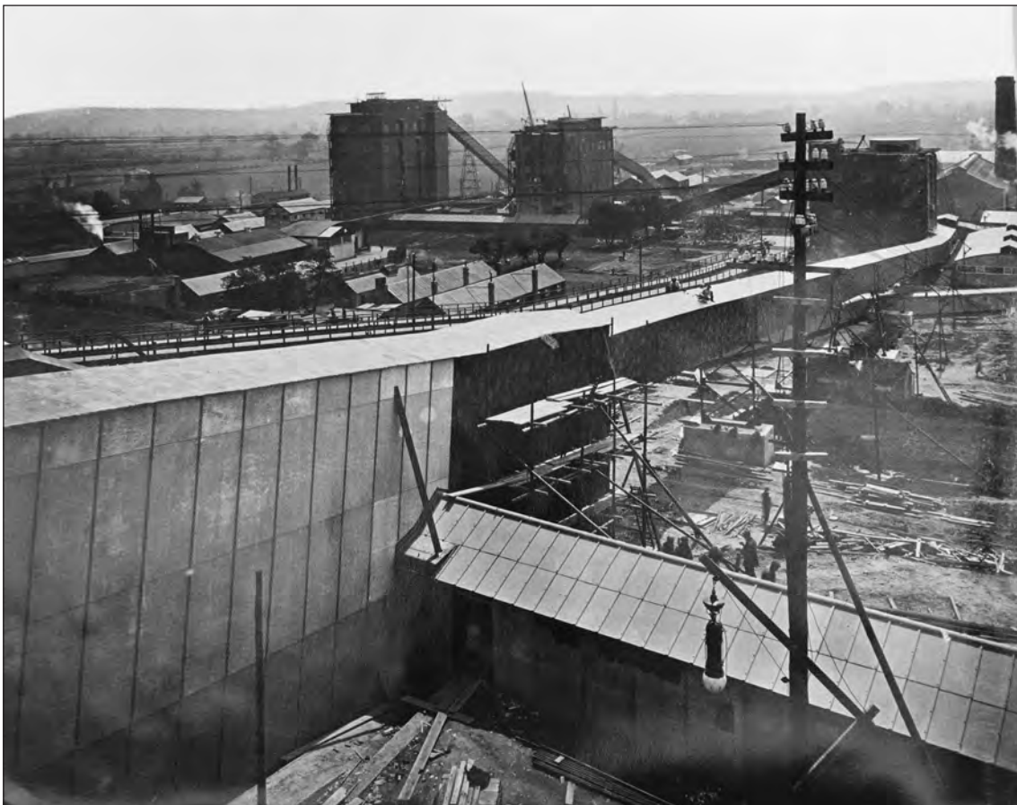
Fig. 4.26. NFF No. 6 Chilwell. View taken on 17 May 1916, looking south. The ammonium nitrate mill is on the centre left, with the TNT mill next right, then the mixing house. Covered conveyor belts carry the mixed amatol to the press houses located behind the camera position (© Historic England AA96/03602).
