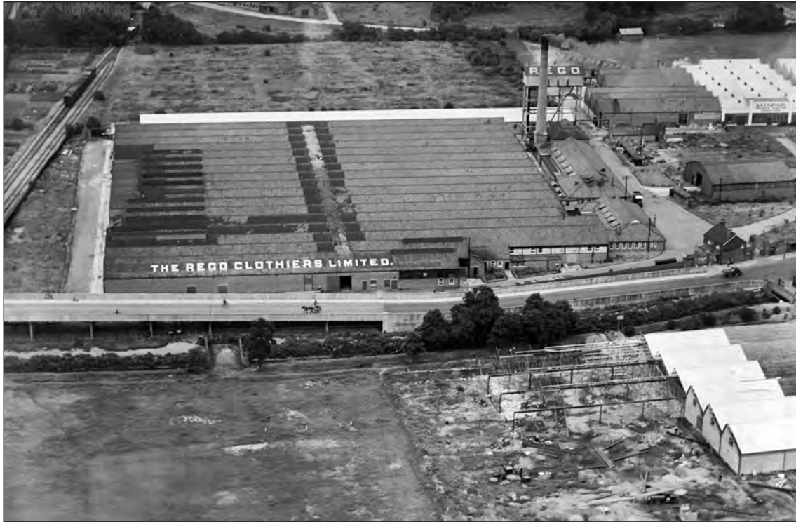
Fig. 4.33. GCF No.4 Edmonton, air photograph, 1933 (© Historic England EPW042088).
