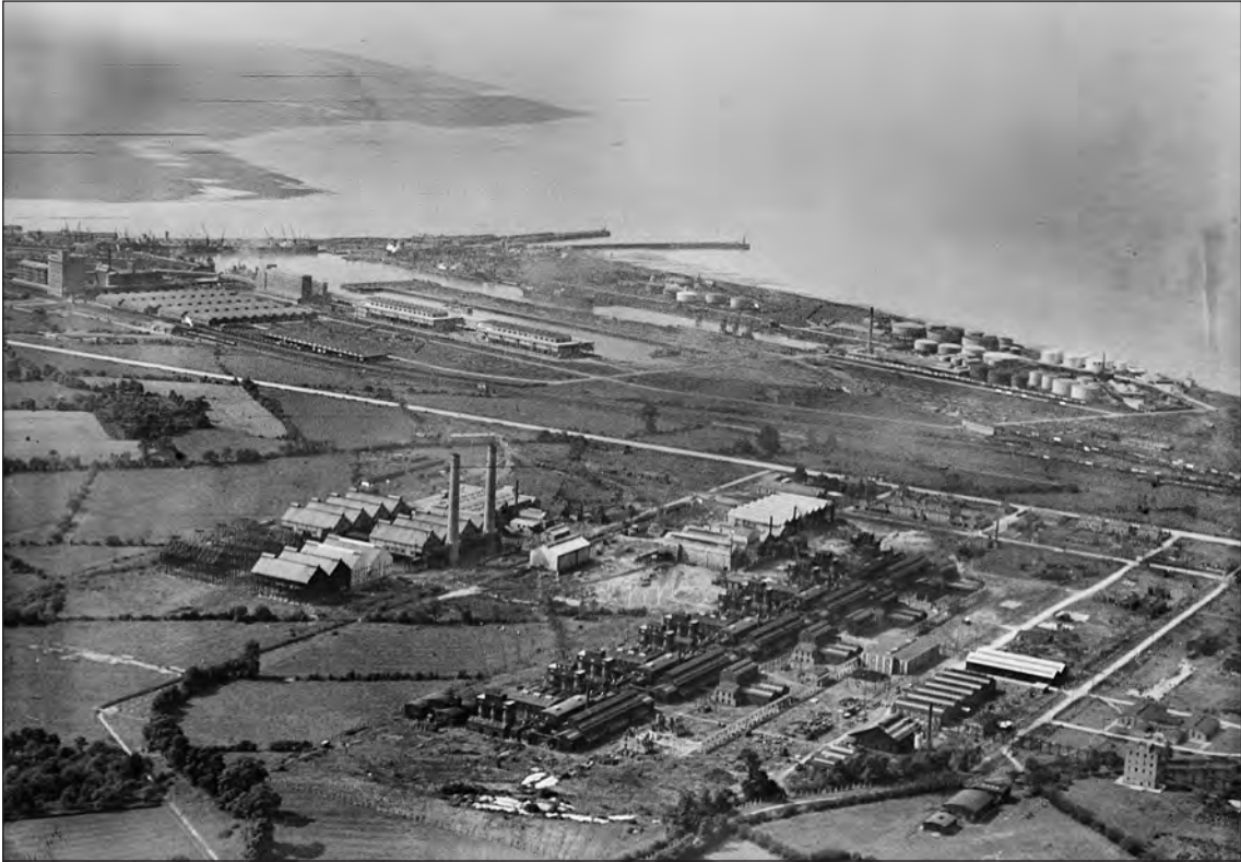
Fig. 4.10. HMEF Avonmouth, air photograph, 1927 (© Historic England EPW019264).
