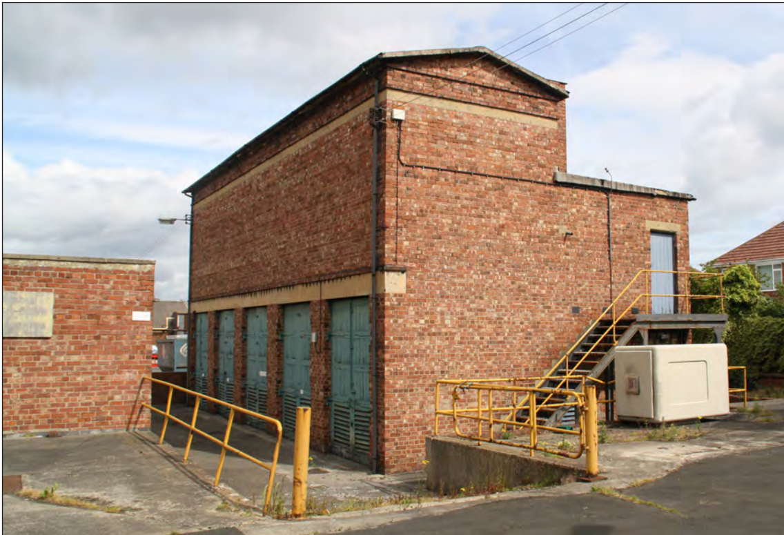
Fig 3.7. NPF Birtley, surviving electricity sub-station (W Cocroft).
