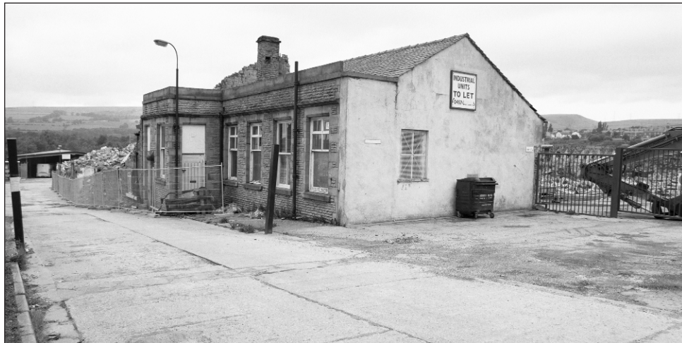
Part of mill, now demolished. (English Heritage BF055199) Other buildings may survive.
