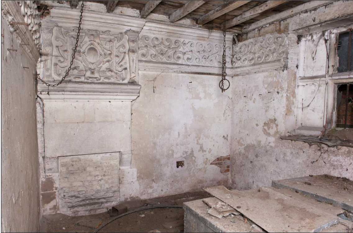
Figure 18: The north wall of the first-floor north-east room with its fireplace and overmantel and the partition to the left (DP220855)
