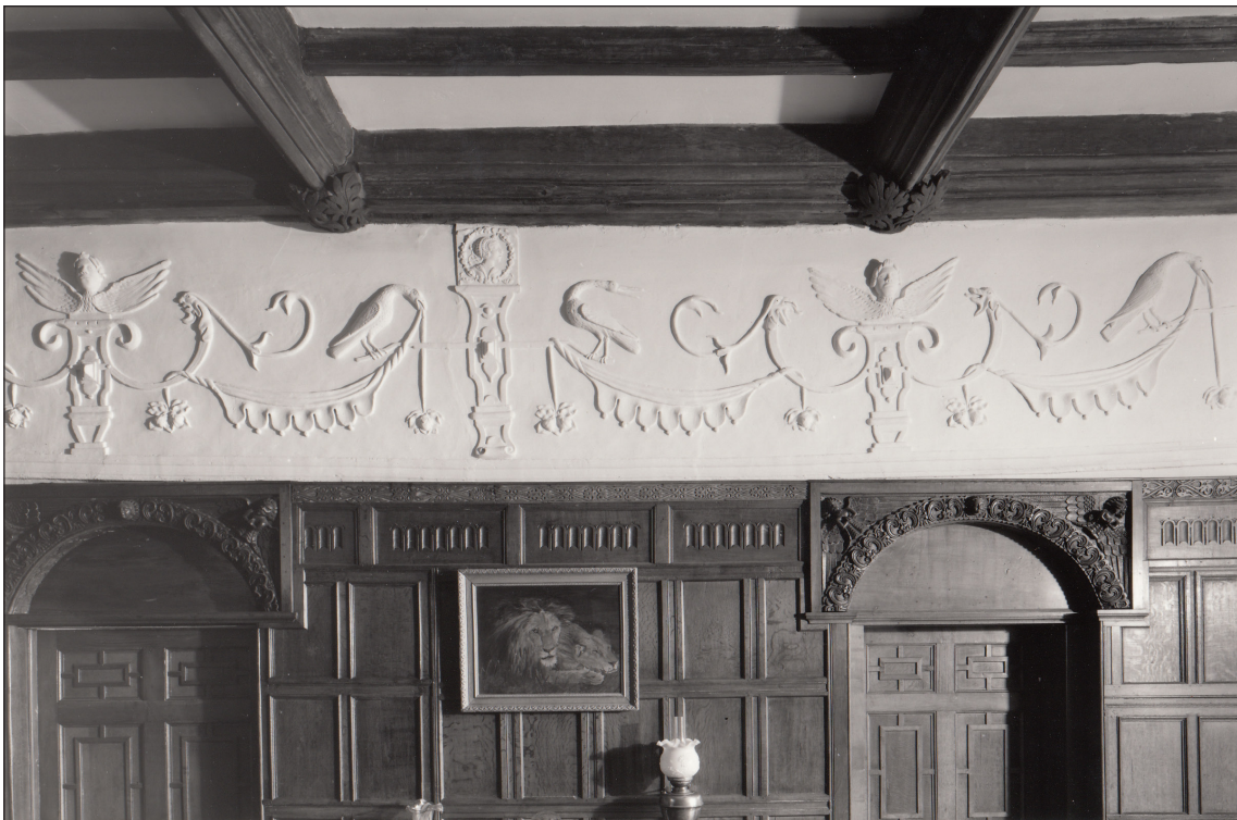
Figure 29: Central section of the plaster frieze in the hall of the Old Council House in Shrewsbury, photographed in 1985 (Historic England Archive, BF035801)
