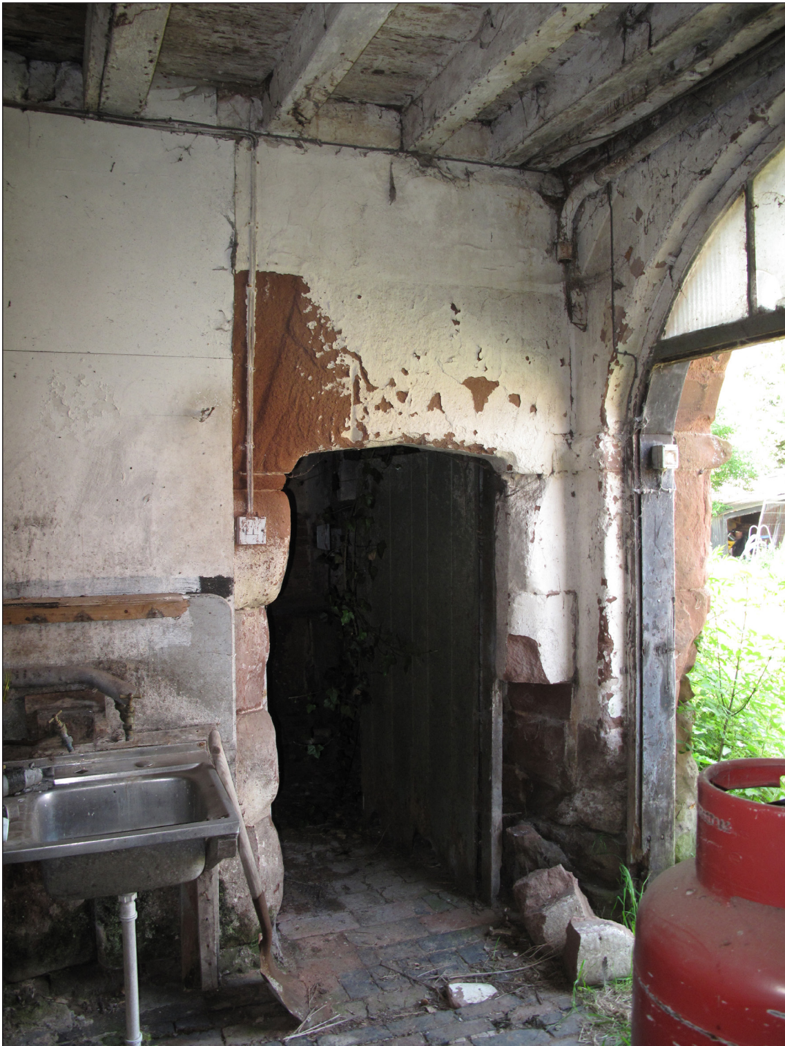
Figure 17: The archway into the ground-floor south room, looking southwest (Rebecca Lane)
