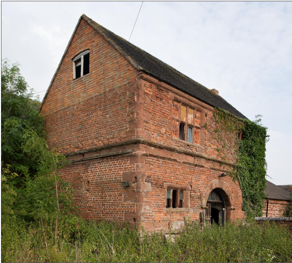
Figure 11: The gatehouse from the north-west (DP220883)
