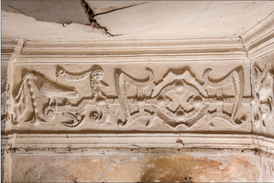
Figure 20: Detail of the plasterwork frieze on the south wall showing the repeating motifs of birds holding swags, S-shaped strapwork and a strapwork cartouche (DP220829)
