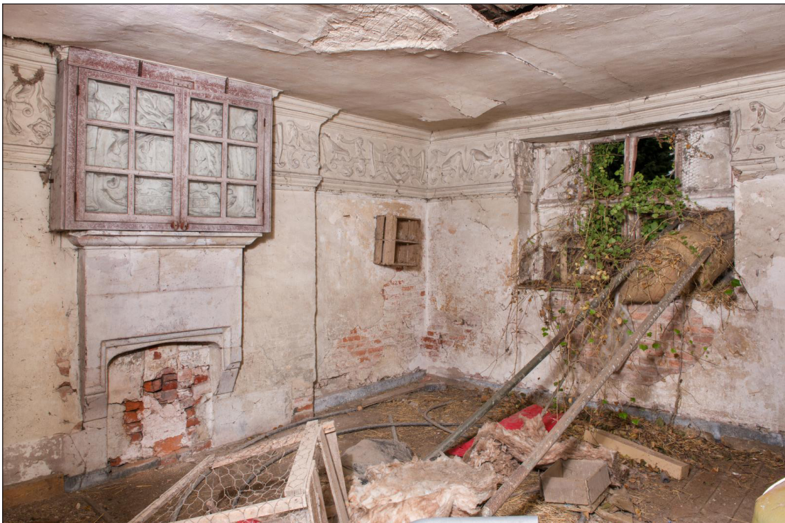
Figure 19: The first-floor south room, looking south-west (DP220850)
