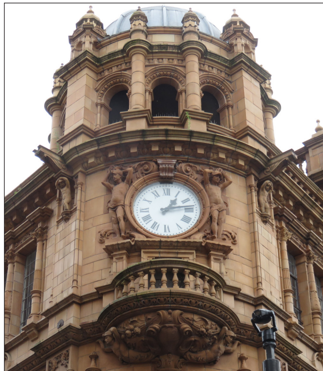
Fig 14. Decorative glazed terracotta around Boots' clock face on the corner of Pelham Street and High Street. (© Historic England, K. Morrison)
