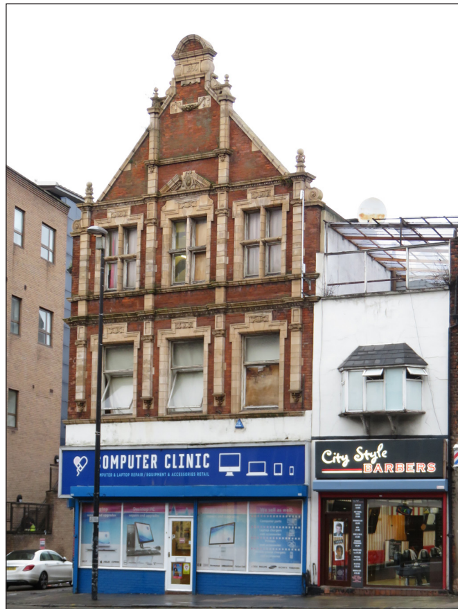
Fig 5. Former Boots, London Road, Liverpool, built in 1896 and photographed in 2017. (© K. Morrison)
