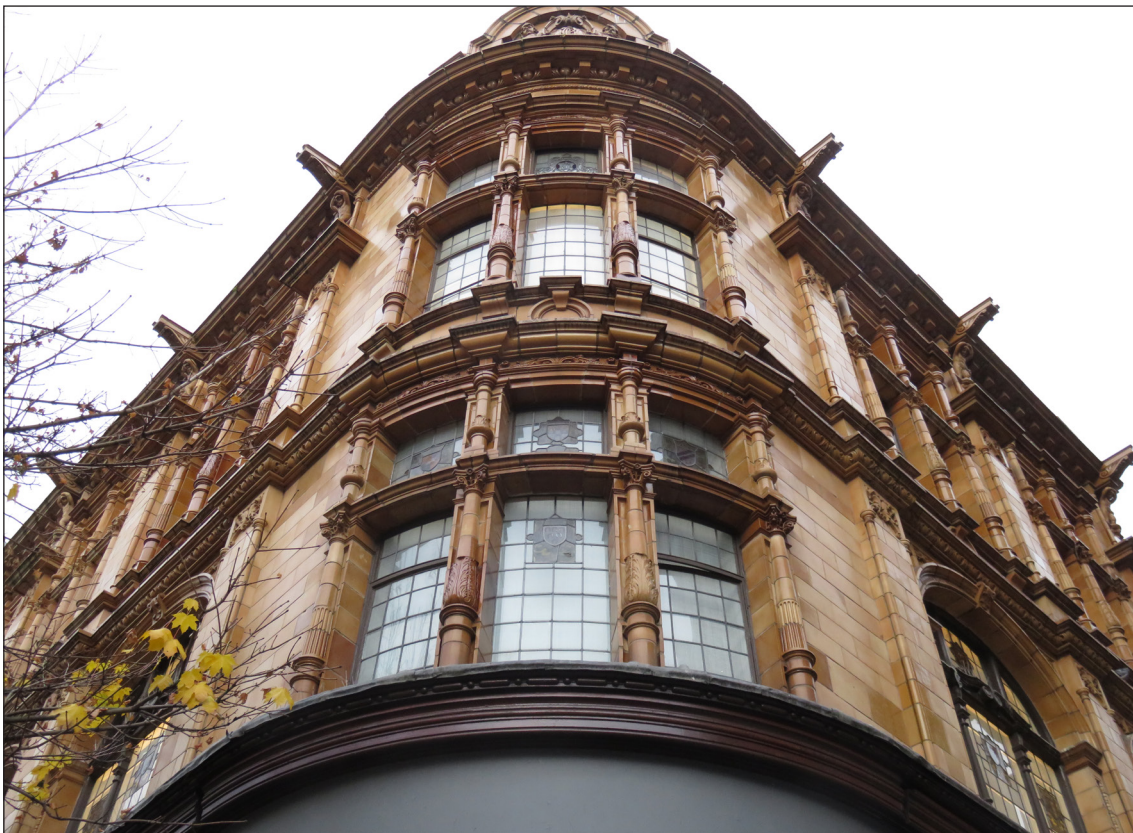
Fig 21. The south-west corner of Boots' building, which was added in the 1920s. (© Historic England, K. Morrison)
