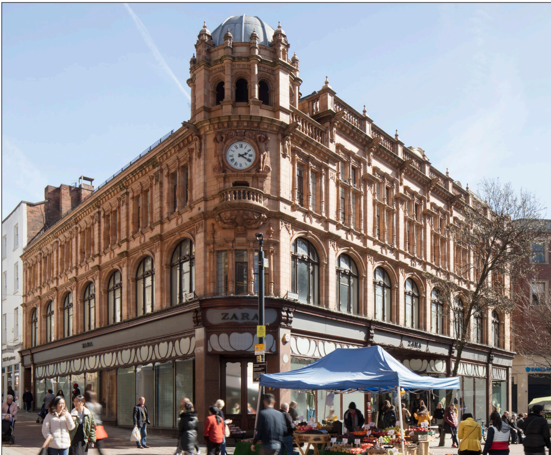
Fig 12 (below). General view of the Pelham Street store. (© Historic England, Pat Payne)
