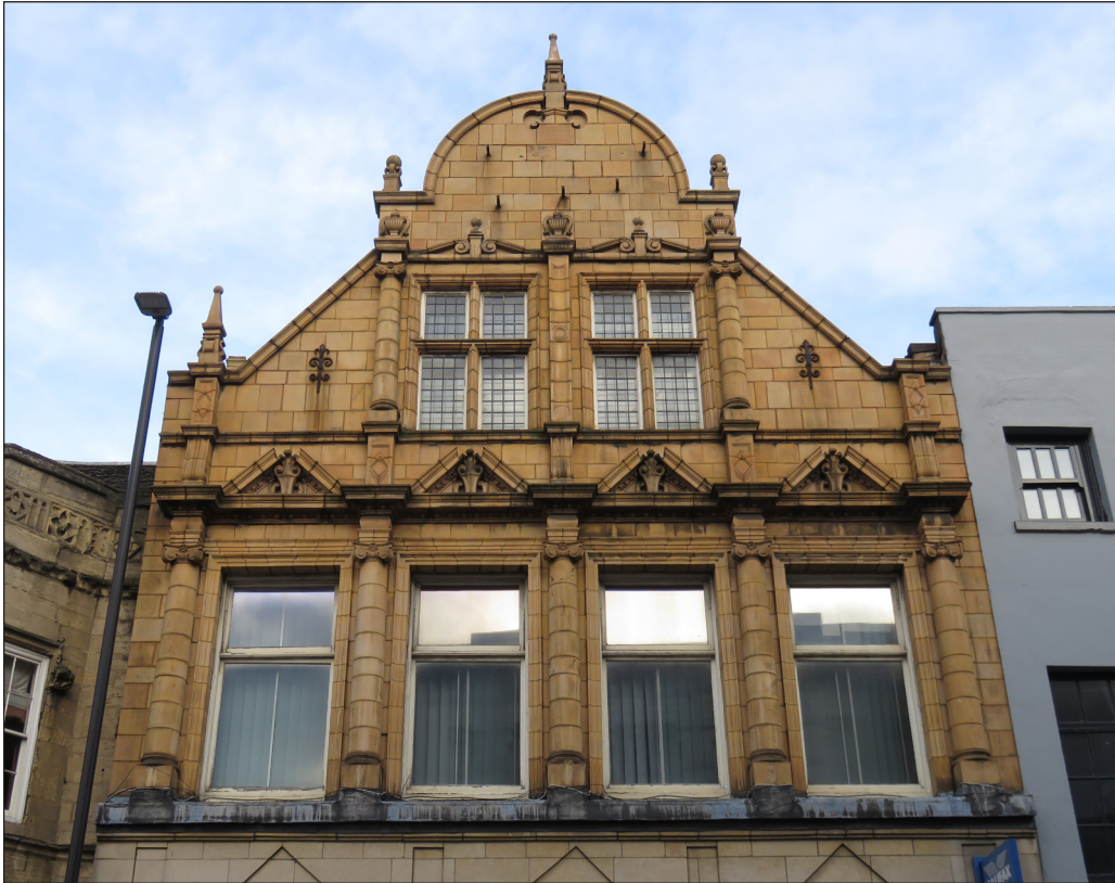
Fig 6. Former Boots, High Street, Grantham, built in 1899 and photographed in 2017. (© K. Morrison)
