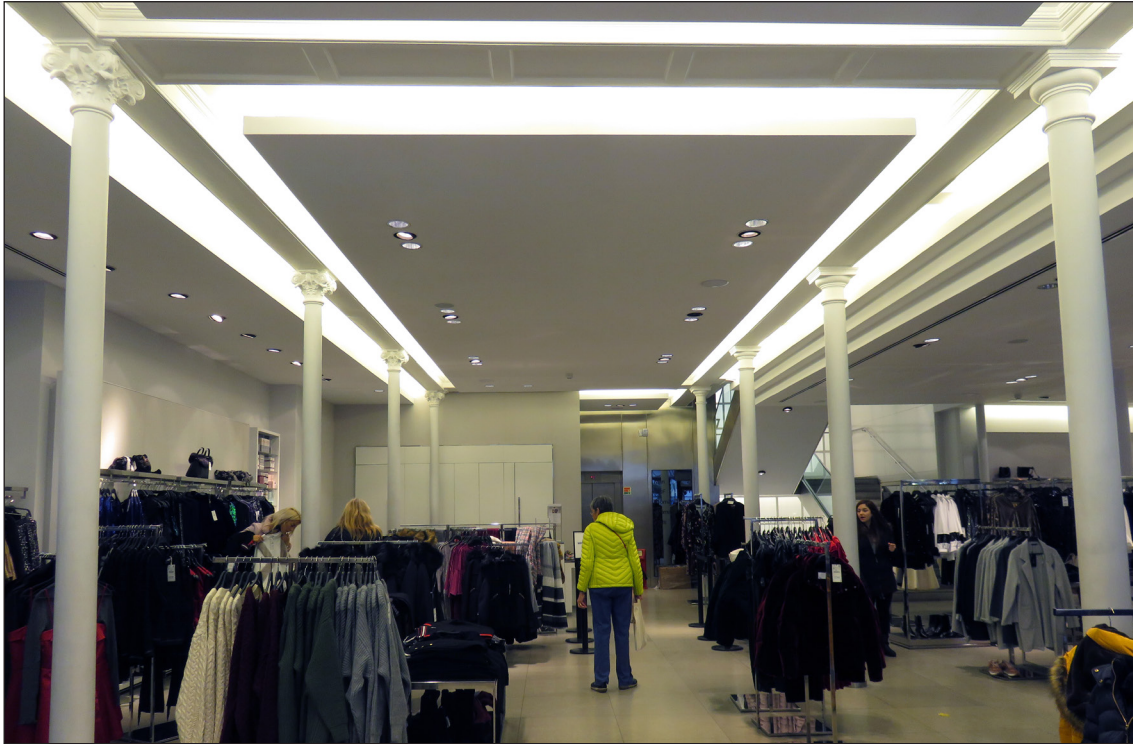
Fig 19. Interior of ground floor of Zara: the columns and capitals which once carried the 1892 gallery (see fig 2) are on the left; those on the right were added in 1902-05. (© Historic England, K. Morrison)
