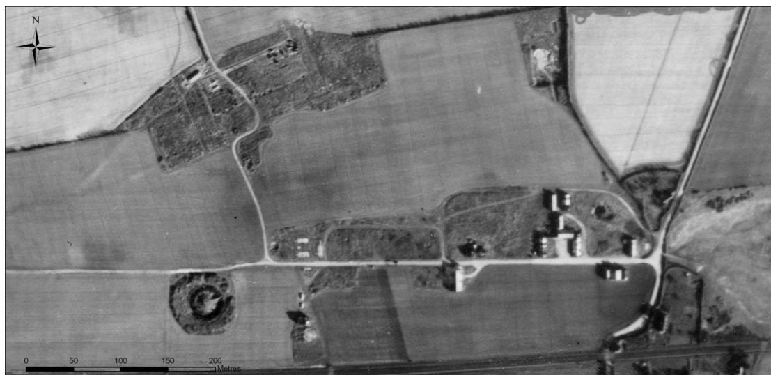
Figure 81. Possible site of First World War Airship Station, Crossways.
