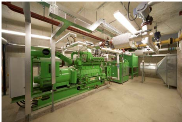
Figure 18: CHP engine at Grosvenor Waterside, SW1
