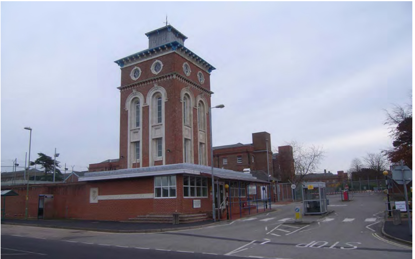
Plate 14: HUCA 14: Haslar Hospital entrance and water tower
