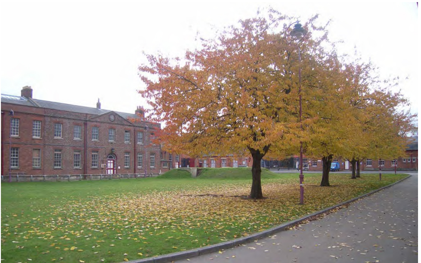
Plate 4: HUCA 4: General view of Buildings at Priddy's Hard
