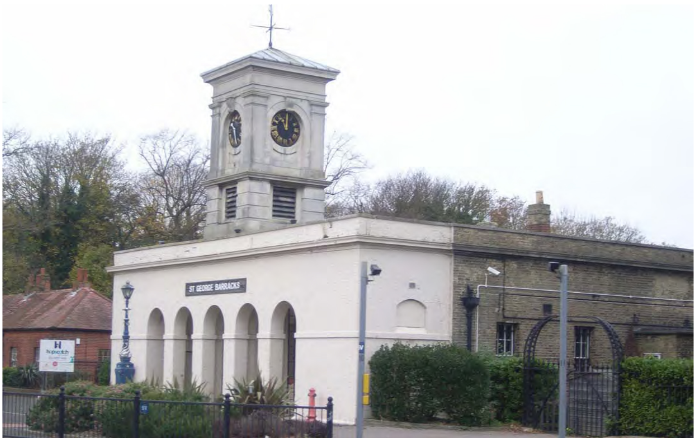
Plate 2: HUCA 2: Entrance to St George's Barracks
