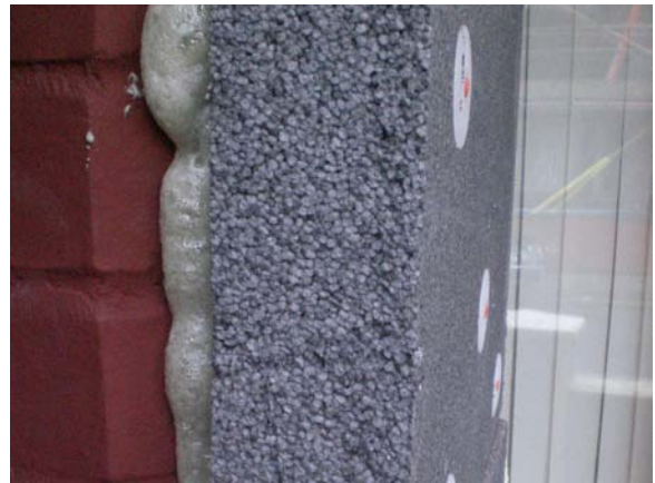
Figure 61 Use of expanding foam rather than cut EPS 68
