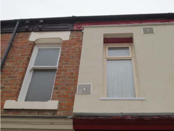
Figure 16 Untreated vs treated window, Note new sill
