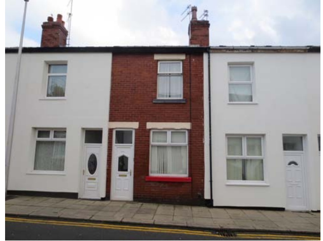
Figures 74 & 75 Note different approaches to lintels, i.e. leaving exposed or covering: leaving them exposed retains the feature but increases the thermal bridge, covering them creates a cleaner look and increases insulation coverage
