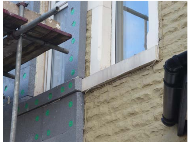
Figures 94 & 95 Conventional EWI window sill (left) vs recreated – and insulated – original stone sill (right)
