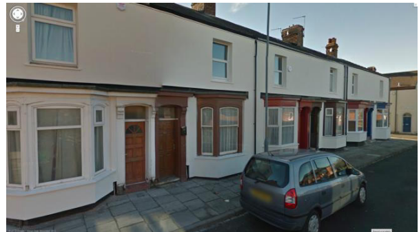
Figures 42 & 43 Properties with bay windows (some new, some not); also note lack of eaves brickwork detailing 56
