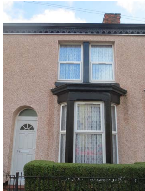
Figures 56 – 57 Note the challenges of insulating bay windows; also upper-right window surrounds untreated. The thermal benefit of the thin section of insulation below the left-hand ground-floor bay window is unclear
