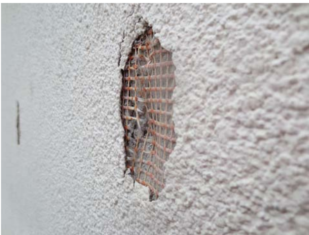
Figures 34 – 37 Several areas of failing render finish; reasons for this are unclear, possibly impact or unsuitable application
