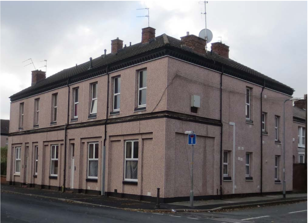
Figure 64 Note the high area of uninsulated wall area in this building; reasons for some of the untreated areas are not clear
