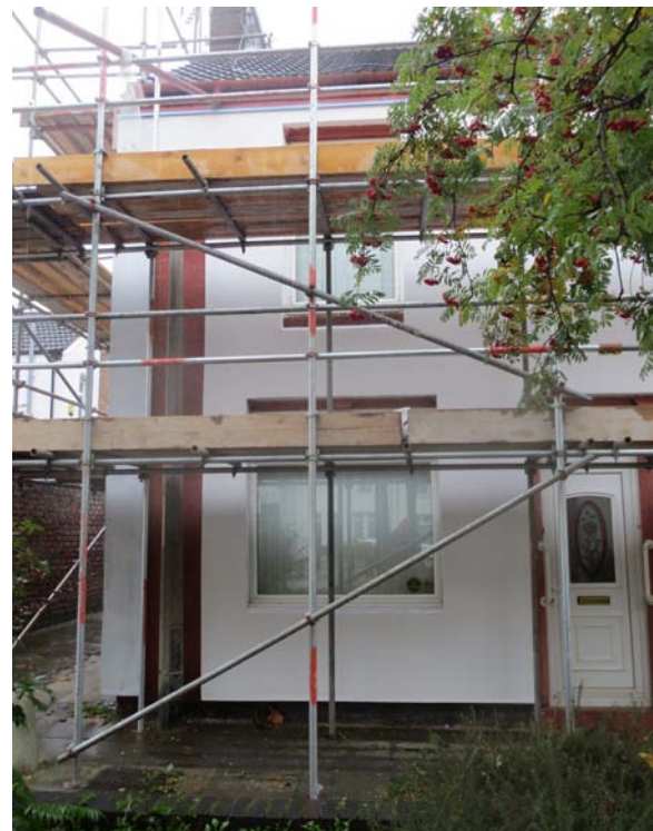
Figure 25 Large thermal bridge created by lamppost
