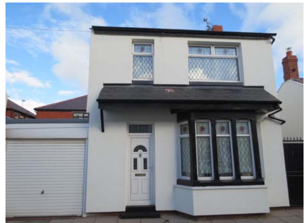
Figures 80 – 83 Note large uninsulated areas: vennels, gas pipes, porch roofs, window & door surrounds
