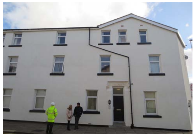
Figures 96 & 97 The property on the left is untreated; the property on the right is insulated but maintains the original aesthetic through detailing such as painted stone-effect window sills and soft corners at window reveals
