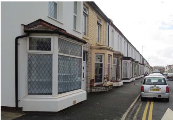
Figures 78 & 79 Bay windows leave large areas of untreated wall at ground floor level; gable ends are simpler
