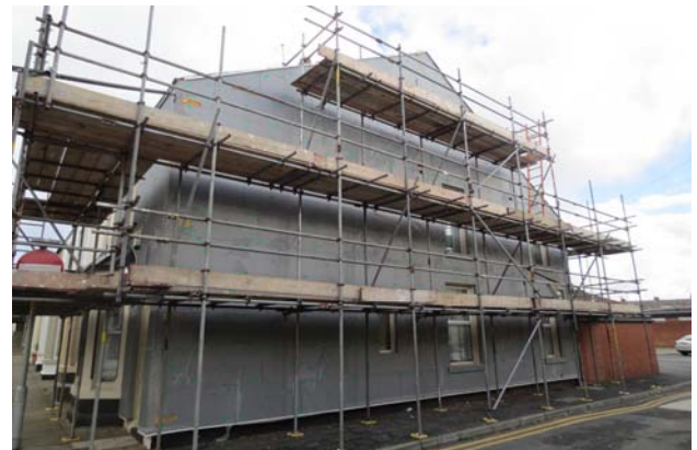
Figures 78 & 79 Bay windows leave large areas of untreated wall at ground floor level; gable ends are simpler
