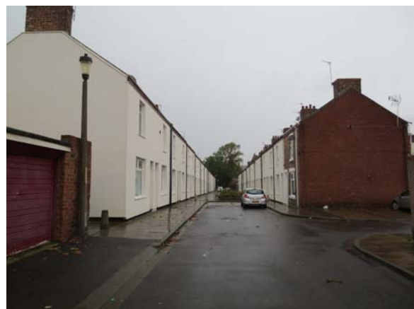
Figures 7 – 9 The visual impact; note the more uniform appearance where all properties are treated. Also note the thermal bridge at ground level
