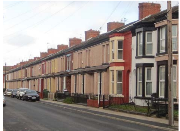
Figure 53 Porch roofs creating a thermal bridge
