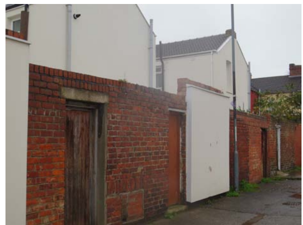
Figure 31 Insulation to end wall
