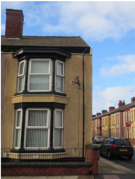
Figures 56 – 57 Note the challenges of insulating bay windows; also upper-right window surrounds untreated. The thermal benefit of the thin section of insulation below the left-hand ground-floor bay window is unclear
