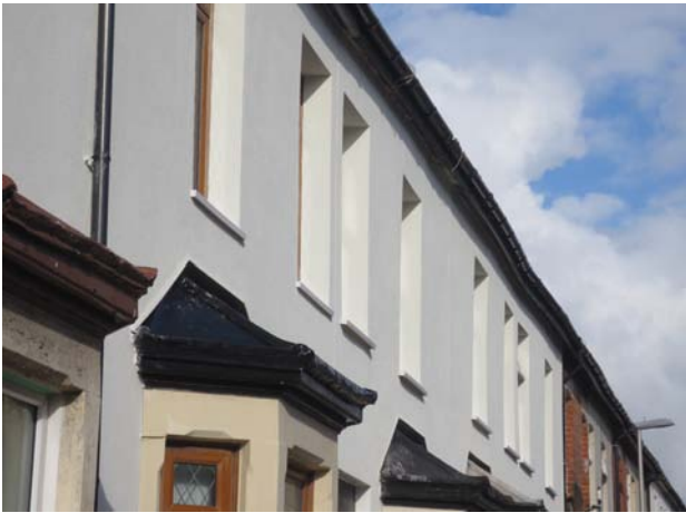
Figures 94 & 95 Conventional EWI window sill (left) vs recreated – and insulated – original stone sill (right)
