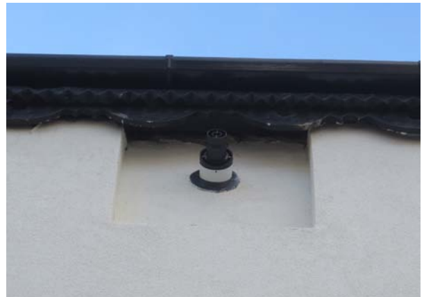
Figures 86 & 87 Uninsulated boiler flue surrounds (note flashing on left vs no flashing on right)
