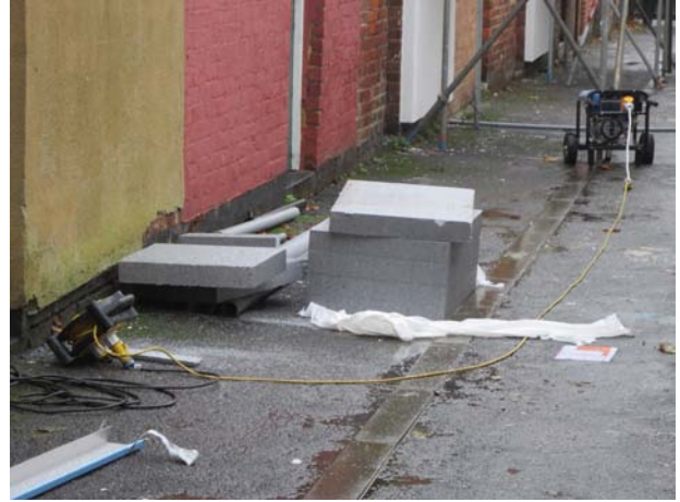
Figure 27 Wet EPS boards awaiting installation
