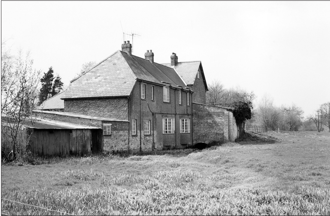
Figure 24 – Lewell Mill Farm, West Knighton, Dorset: the arch of the tailrace can be seen at the base of the wall of the wheelhouse to the right of the farm- (or rather mill-) house with the derelict channel of the former tailrace visible in the foreground; beyond, the embankment for the head race is visible (1960 Joseph Addison © Historic England aa042870)
