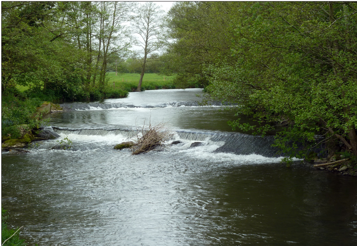
Figure 12 – Two angled weirs on the River Arrow, upstream from Penbridge, Herefordshire; the upper feeds a leat running off left to the Court of Noke water gardens and mill and the lower a leat to the right supplying a waterwheel at Leen Farm (© Alan Stoyel, with permission)
