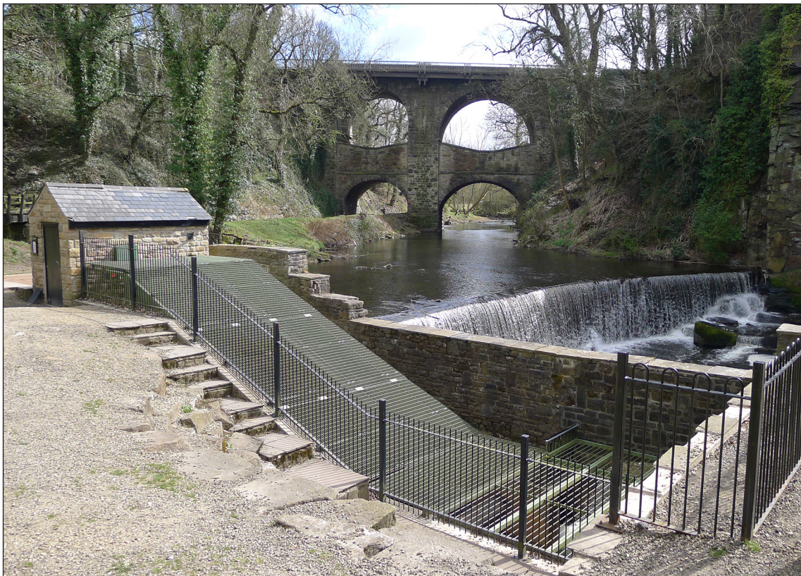
Figure 25 – A micro-hydro generation installation on a weir at Tor Mills, Derbyshire, with an Archimedes screw turbine within the protective cage behind the railings in the foreground (Matthew Edgeworth © Historic England)
