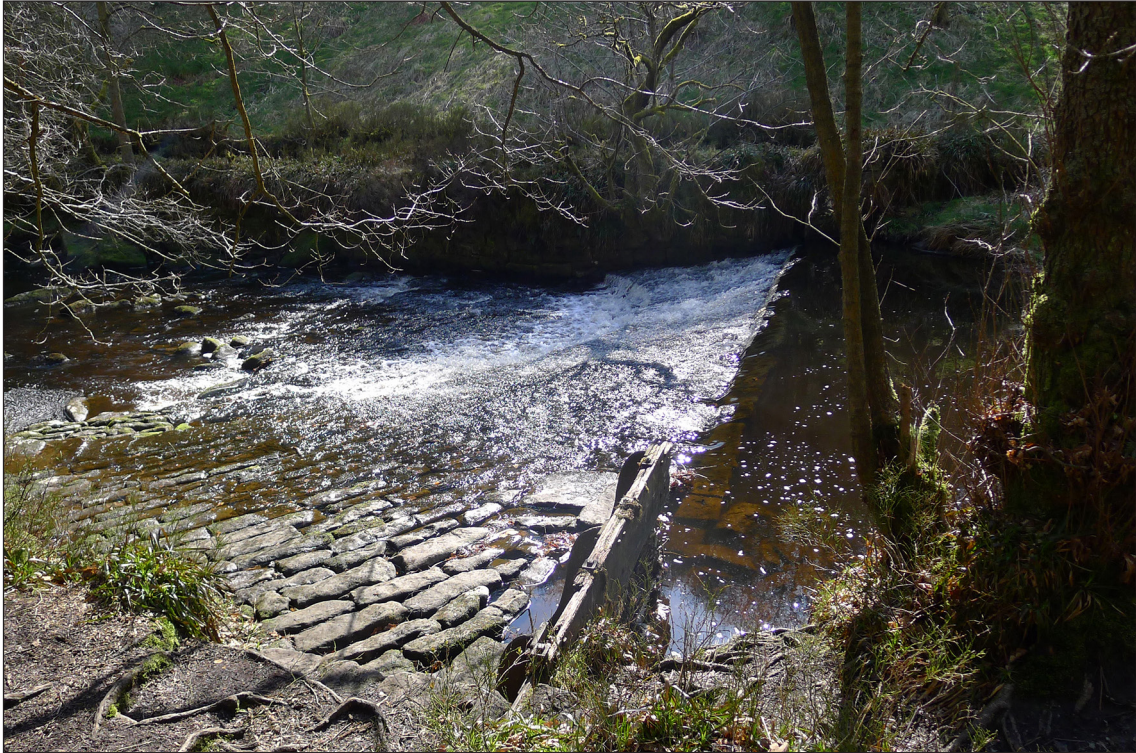
Figure 11 – A pitched stone weir on Hebden Brook, Yorkshire with a surviving section of 'washboard' visible in the foreground (Matt Edgeworth © Historic England)
