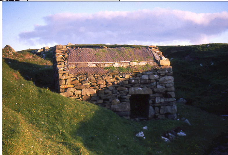
Figure 2 – A typical horizontal mill building in the landscape, the small stream that would have driven the mill can just be made out in the shadows to the right, Shetlands, Scotland (Wayne Cocroft, with permission)
