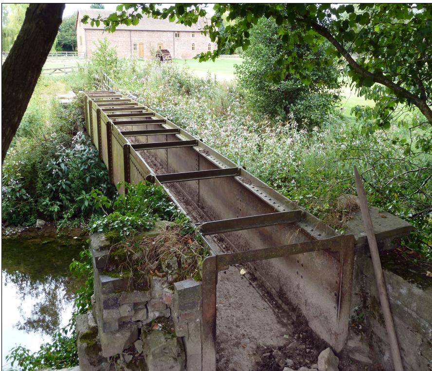
Figure 16 – A metal aqueduct across the River Lugg at Day House, Kingsland, Herefordshire, with the farm mill and waterwheel visible in the background (© Alan Stoyel, with permission)
