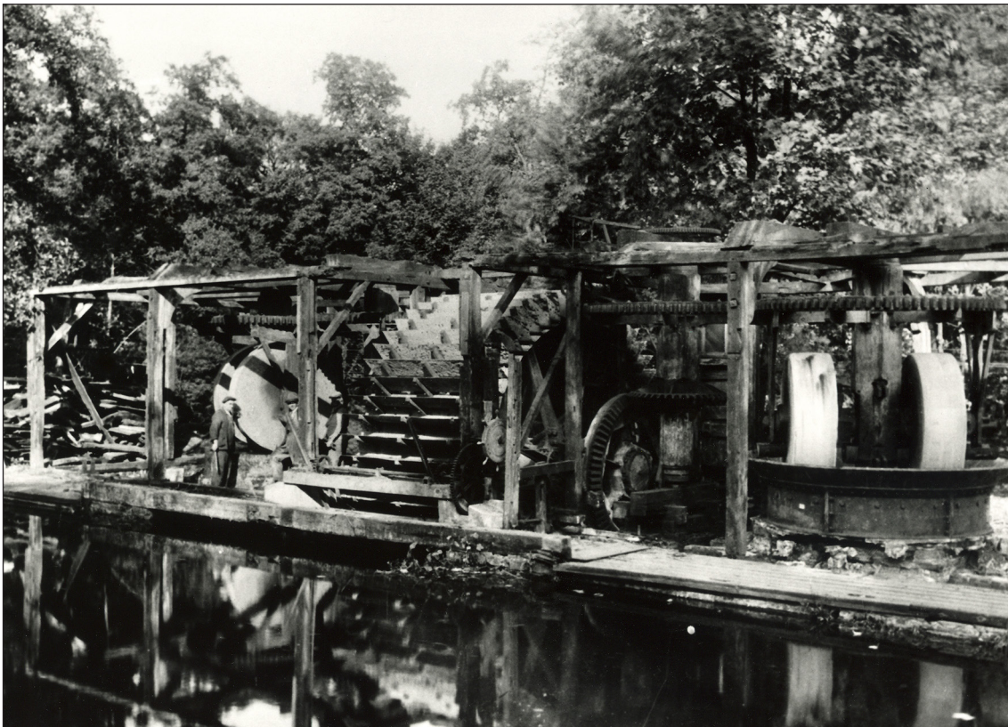
Figure 7 – In 1936, the demolition of No. 3 mill on Millhead Stream at the Royal Gunpowder Factory, Waltham Abbey, Essex, exposed the internal gearing and massive stones of this incorporating mill (BB94/8010 © WASC 139)
