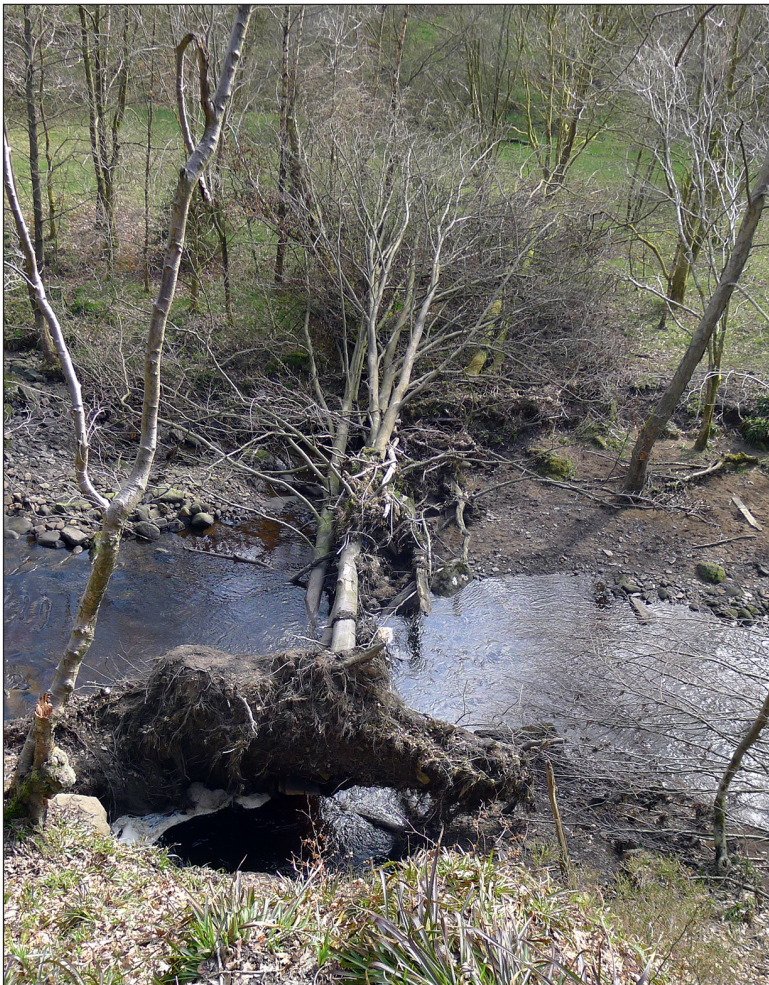
Figure 22 – Erosion has undermined the bank causing this tree to fall across Hebden Brook, Yorkshire, further damaging the bank. Within the channel meanwhile, debris has started to accumulate against the trunk holding up the flow – in flood conditions this could act as a weir forcing water out of the channel leading to further erosion and deposition altering the form of the channel (Matthew Edgeworth © Historic England)
