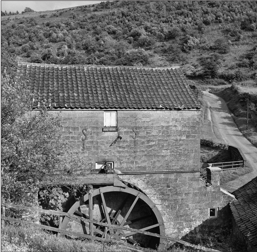
Figure 6 – Levisham Mill, Ryedale, North Yorkshire in the 1950s: a mill with a large overshoot wheel; note the pentrough supplying the water to the top of the wheel and the steep local topography which favours this type of mill (John Gay © Historic England aa083599)
