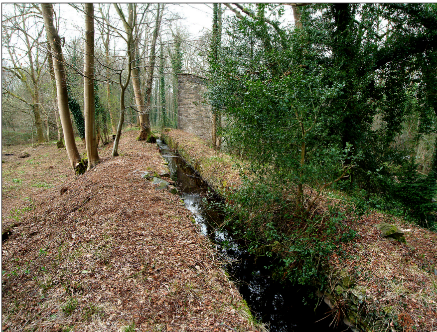
Figure 14 – View of the small, embanked leat running to the lower corning house on the Lowwood Gunpowder Works site, Haverthwaite, Cumbria (Bob Skingle © Historic England DP003477)
