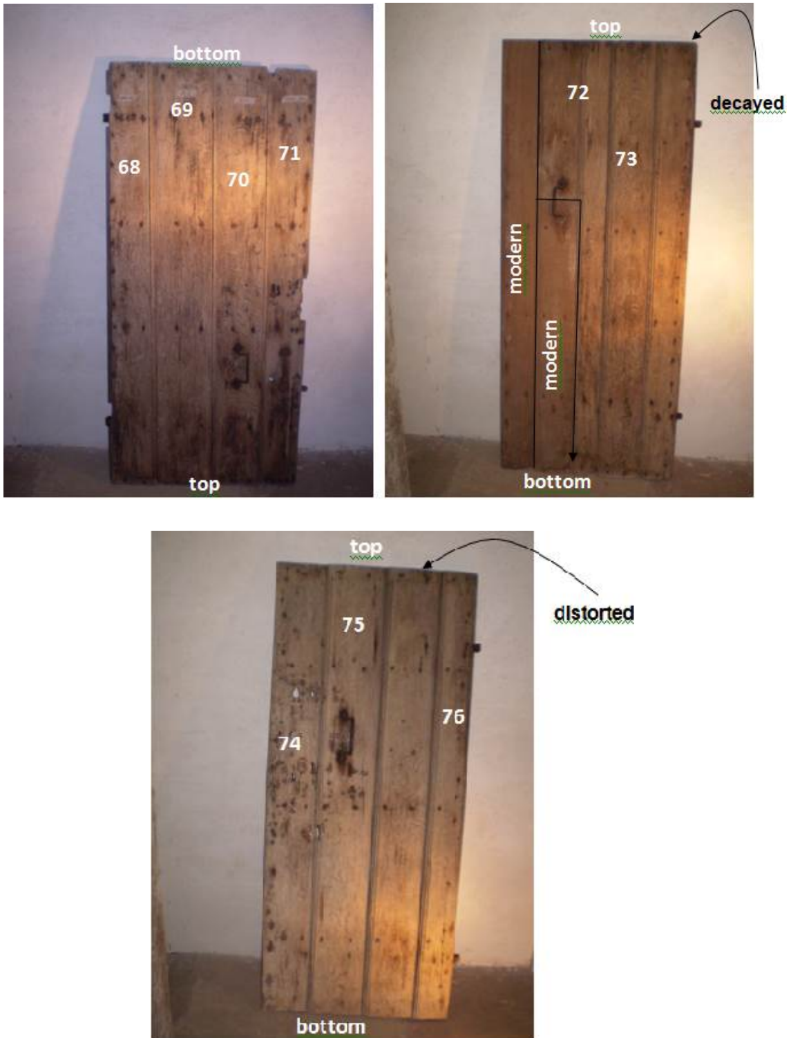
Figure 14a–c: Bedesman room doors to locate sampled timbers (photographs Robert Howard)
