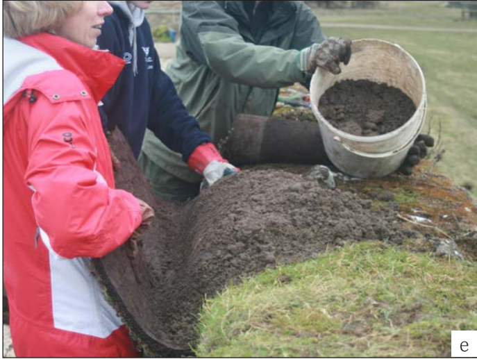
Figure 6.7 (e-h) (e) Sedum mat during installation – the heavy weight of the mat makes it difficult to manipulate. (f) Sedum mat after installation (g) Edges of Sedum mat after. (h) Sedum mat after 7 years showing loss of soil and Sedums at edges. (all ©Alan Cathersides)
