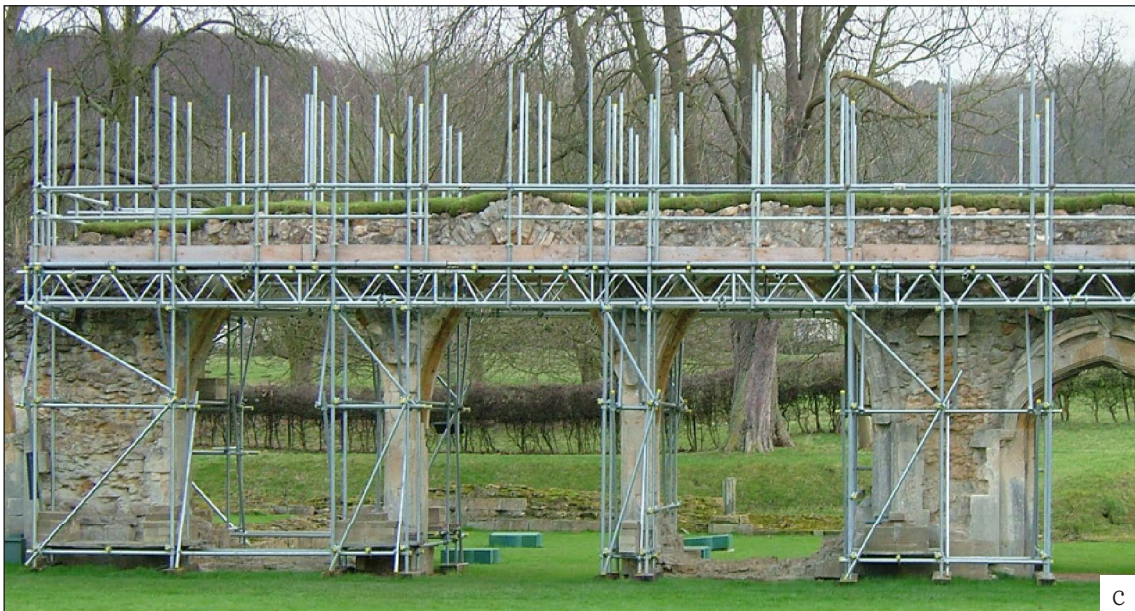
Figure 2.12c Soft capping was installed over the wall head in the east cloister at Hailes Abbey, where previous consolidation and lime mortar repairs had been carried out. ©Heather Viles, University of Oxford
