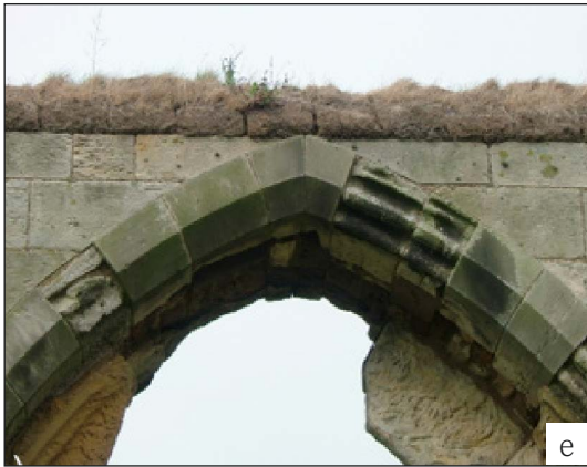
Figure 2.10 c,d,e (left) The soft capping installed at high elevation on the west Front wall at Whitby Abbey. (all ©Heather Viles, University of Oxford)
