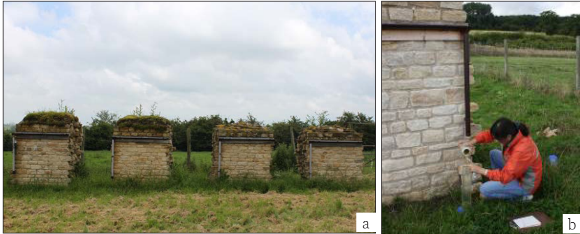
Figure 3.16 (a, b) The test walls with guttering installed, and the set up for collecting runoff in a container, which was then emptied and measured at regular intervals between August 2010 and September 2012. ©Heather Viles, University of Oxford
