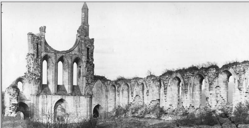
Figure 1.14 Byland in the early 20th century. Source: Historic England Archive (AL0581_009_01)
