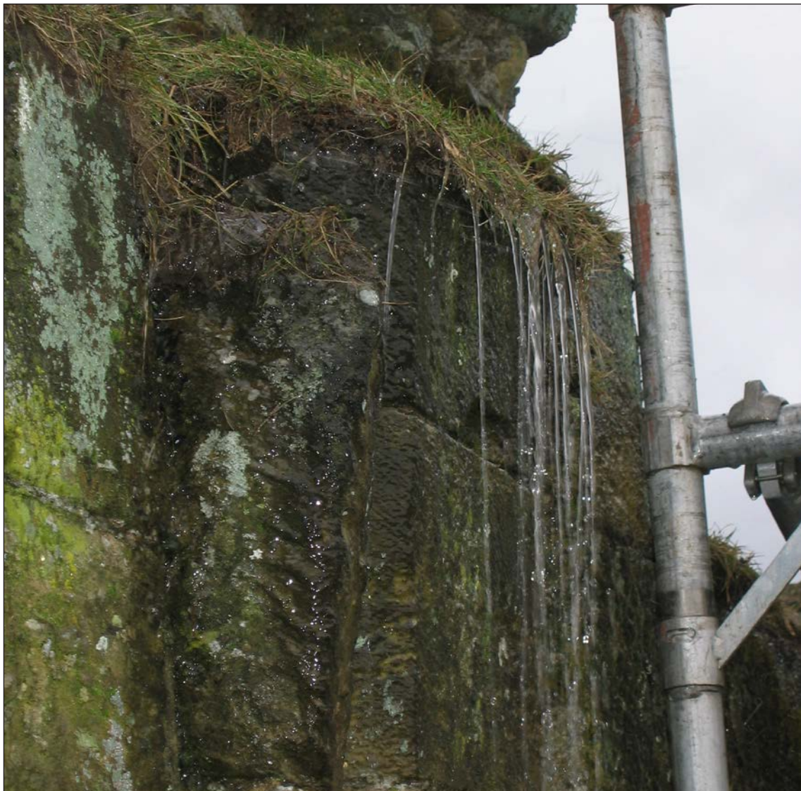
Figure 7.6 The effects of watering newly installed soft capping at Byland Abbey illustrated the water shedding role of even, short turf. ©Chris Wood, Historic England
