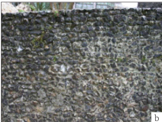
Figure 6.12 (a) An example of a 'natural' site where there has been no previous consolidation and (b) an example of a site where there has been extensive consolidation. (both ©Colin Burns)
