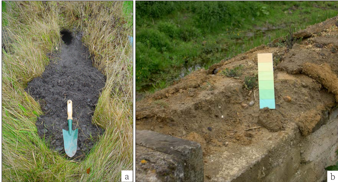
Figure 6.8. (a) A rabbit's trial burrow at Byland Abbey; and (b) damage to the newly installed soft cap at Howbury caused by a fox scrambling up the side of this low wall. (both ©Heather Viles, University of Oxford)
