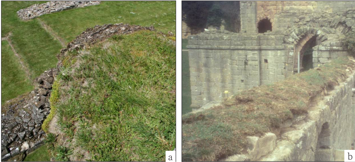
Figure 1.6 (a-b) Soft capping trialled at (a) Kirkham Priory, 1993 and (b) Fountains Abbey in the late 1980s. (a Chris Wood © Historic England ; b © Rory Ogilvie )
