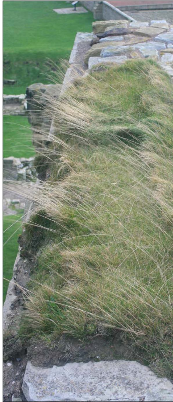
Figure 2.10 c,d,e (left) The soft capping installed at high elevation on the west Front wall at Whitby Abbey. (all ©Heather Viles, University of Oxford)
