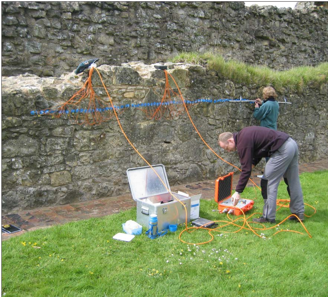
Figure 3.10 2D resistivity survey on the east face of the long test wall at Byland Abbey. The blue dots are adhesive ECG electrodes. The left-hand side is the hard-capped section. © Chris Wood, Historic England
