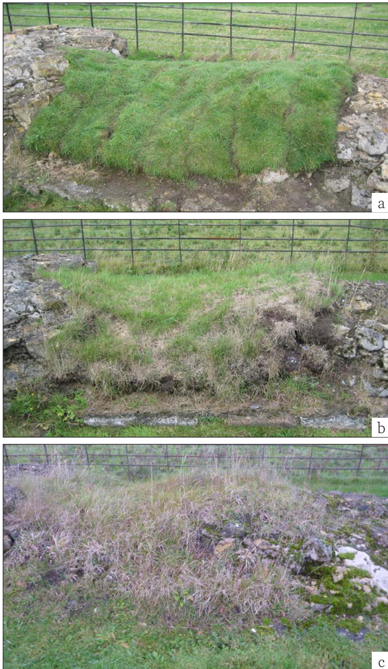
Figure 7.7 One of the soft capped areas at Thornton Abbey, (a) at the time of installation, (b) 18 months after installation, and (c) in November 2016. (all ©Chris Wood, Historic England)
