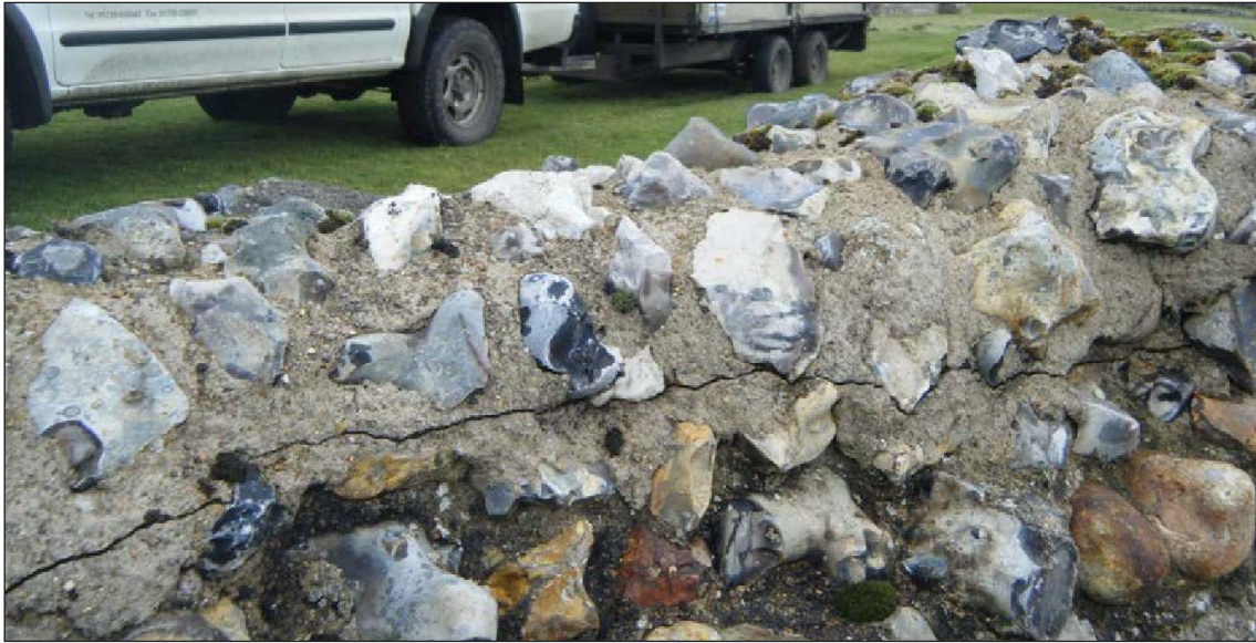
Figure 2.15c Detachment of hard capping from underlying low walls, at Castle Acre Priory in 2012. ©Heather Viles, University of Oxford
