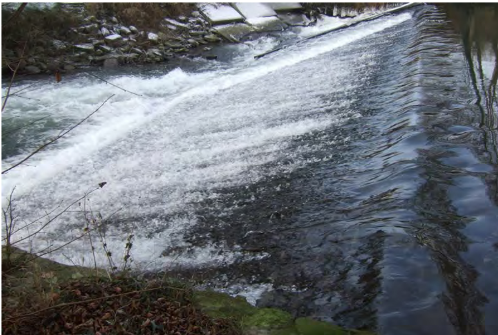
Fig. 3 Mortimer's Cross Mill, Lucton: a massive weir almost straight across the river.
