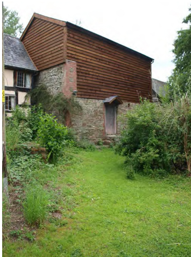
Fig. 11. Wegnall Mill, Rodd Nash & Little Brampton: the re-boarded timber-framed mill.
