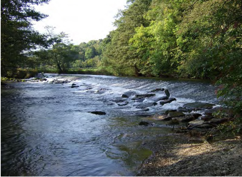
Fig. 2. Aymestrey Mill, Aymestrey; a very long oblique weir.
