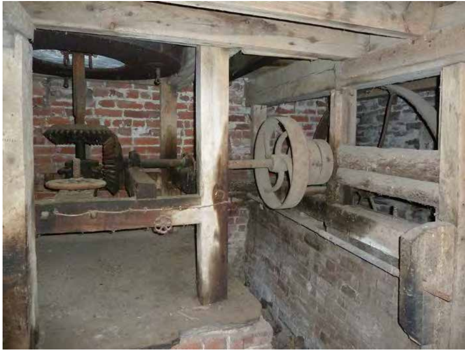
Fig. 14. Court of Noke Mill, Pembridge: mid 19 th cent. machinery - to chaff-cutter to right and drive to millstones at left.
