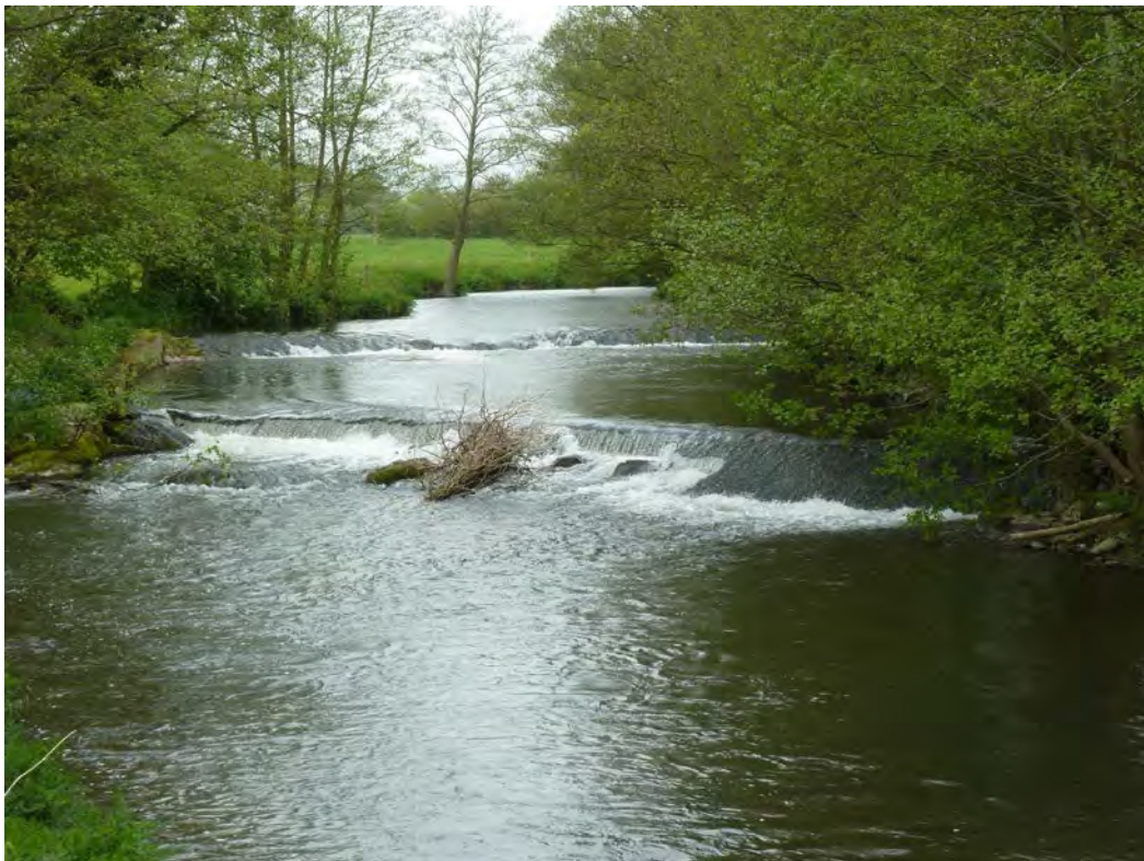
Fig. 19. Court of Noke, Pembrokeshire: pair of weirs. The upper one feeds Court of Noke water gardens & mill to the left of the photograph, and the lower weir fed a leat to the right for the waterwheel at Leen Farm, Pembrokeshire.
