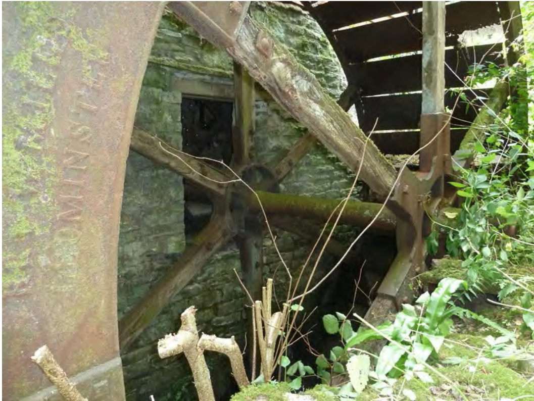
Fig. 12. Wegnall Mill, Rodd Nash & Little Brampton: the low breast-shot waterwheel.
