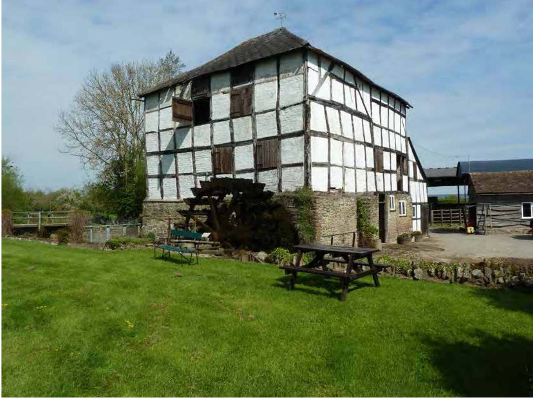
Fig. 32. Arrow Mill, Kingsland: the mill and waterwheel.
