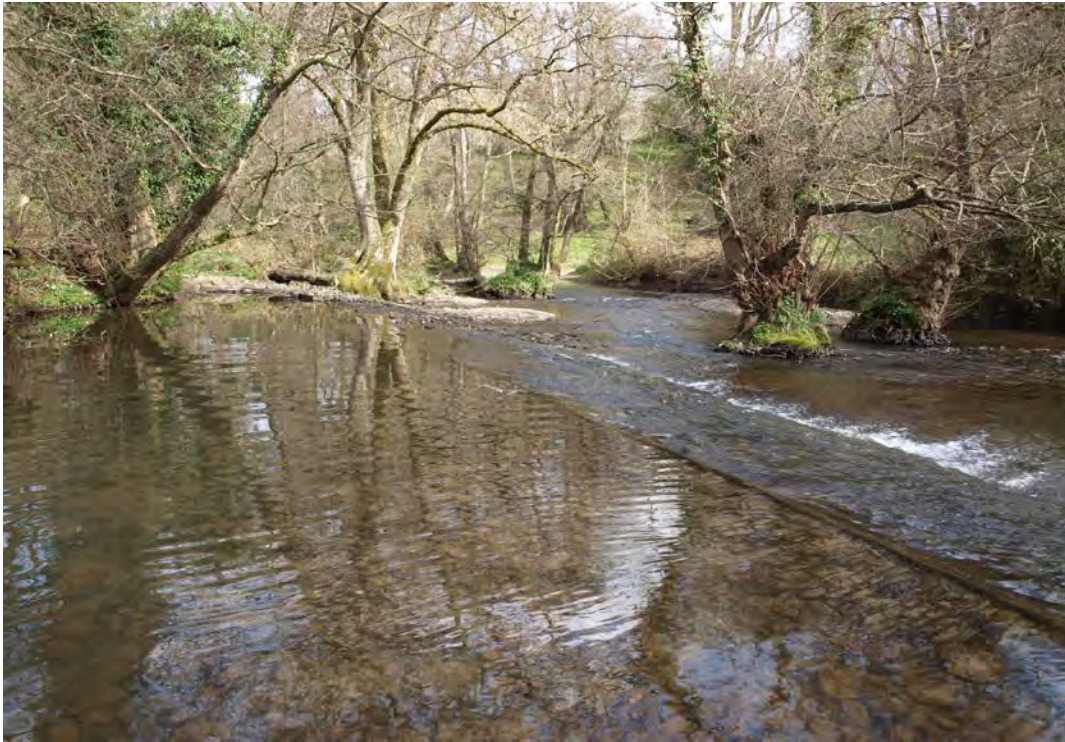
Fig. 4. Crabtree Mill, Kington: a beautifully constructed, ancient oblique weir.
