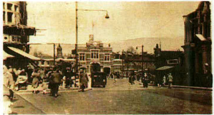
Figure 27 Beresford Square in the 1950s, viewed from Greens End.
