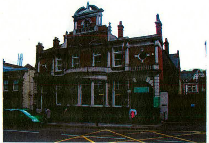
Figure 59 Public Library, 48 Calderwood Street, 1901 by Church, Quick & Whincop. (unlisted).
