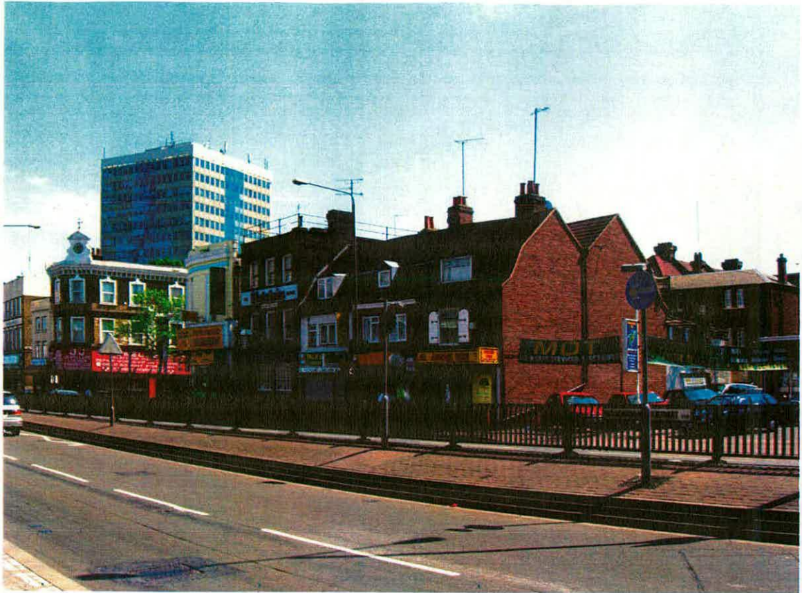
Figure 15 Nos 121-3 Woolwich High Street also survive as three of a group that was four houses, retaining the distinctive form of this 18th-century artisanal house-type, including M-shaped roofs and central-chimneystack layouts. Current uses of this characteristic grouping include an African-Caribbean restaurant (No. 121); an Off Licence (No. 122), and a Thai restaurant. The intimate scale of this survivor, and its eastward, 19th-century neighbours, is compromised both by the looming tower block in the distance and the dual carriageway in the foreground.
