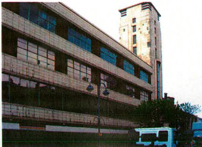
Figure 48 Opposite the original red brick and terracotta Headquarters Building is the streamlined extension of 1938, finished in cream faience and glass. It was designed by S.W. Ackroyd, the company architect, and is currently under consideration for Listing.
