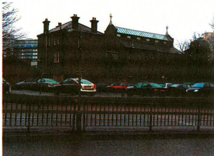
Figure 19 Callis Yard Stables, Brunton Street, as seen from Woolwich High Street. Despite being Not Listed, this urban stables complex built c.1890 makes an important contribution to the riverside townscape, its stock brick elevations complementing neighbouring buildings, and its Italianate detailing adding stylistic richness to the locale. Built by Greenwich Council to house horses and dustcarts, it reflects the early stages of municipal provision in Woolwich and is an attractive surviving example of a once-numerous building type.
