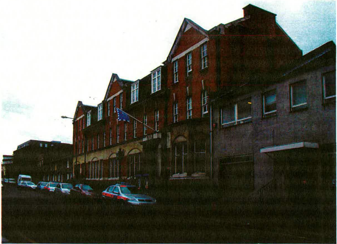
Figure 61 Police Station, 29-33 Market Street (unlisted). Erected in 1910, this Queen Anne style building was designed by John Dixon Butler, architect and surveyor to the police 1895-1920. During this period, Butler designed over 200 police stations and courts for the metropolis.
