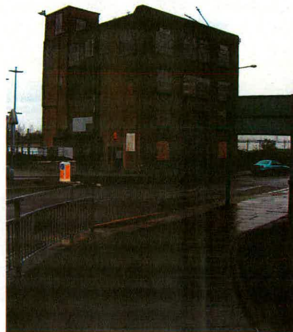
Figure 20 Gatehouse Building, Warren Lane. Erected in 1910 as a purpose-built extension to Furlongs furniture depository in nearby Nelson Street, this four-storeyed stock-brick building bears witness to the former scale of industrial buildings and activity on the riverside.
