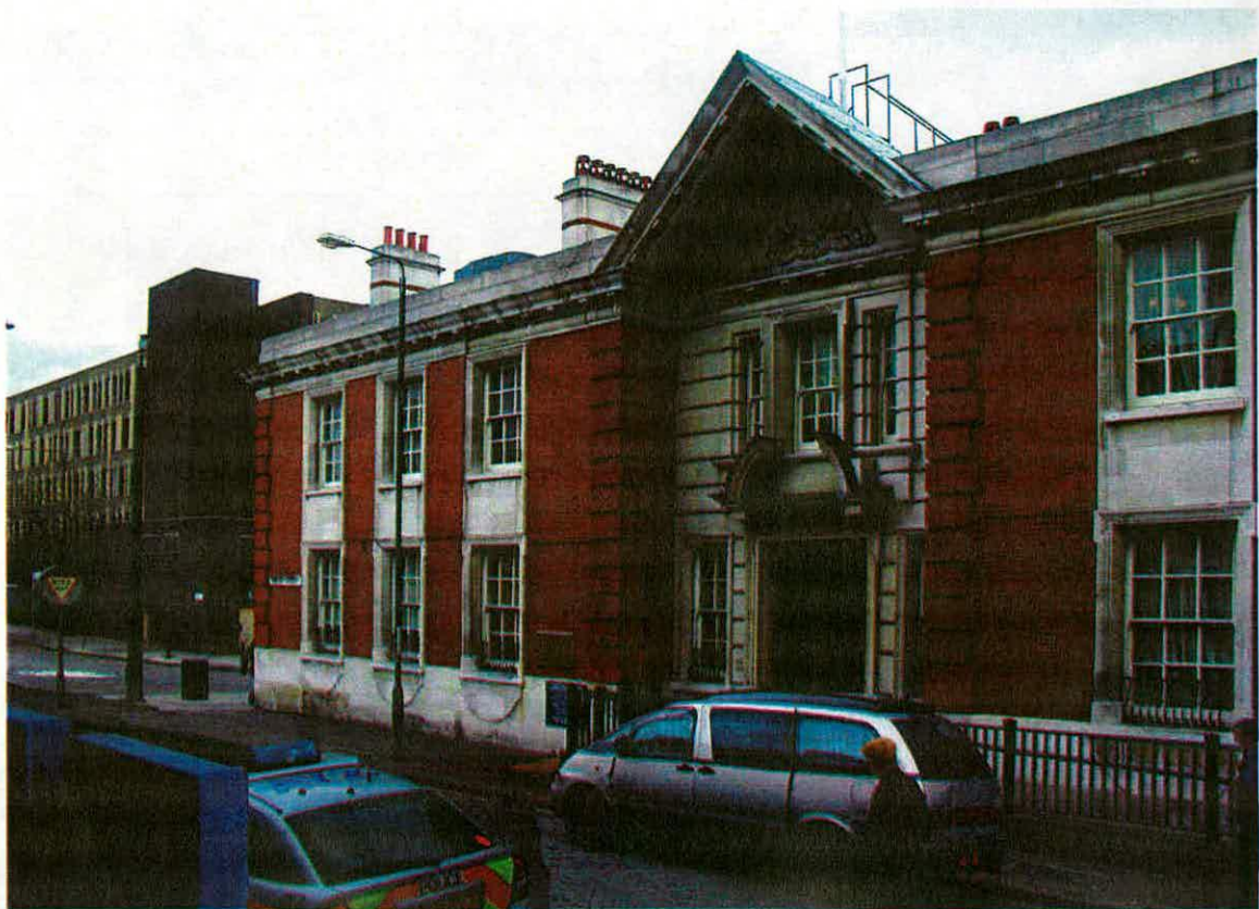
Figure 62 Magistrates' Court, 50 Market Street (unlisted). In the wake of a report produced in 1900 by a House of Commons Committee, which criticised courthouse provision and conditions, an ambitious programme of Edwardian building ensued. John Dixon Butler (1861-1921) developed a distinctive style for these new metropolitan police buildings, 'a crisp, austere version of the prevalent Free Classic or Anglo-Classic – the civic style doffing its regalia and donning a uniform' [Gray (1985), p. 132]. Erected in 1912, Woolwich Magistrates' Court is a fine example of his oeuvre: assured, eye-catching and redolent of Butler's admiration for the work of R. Norman Shaw and Philip Webb, with whom he had formerly collaborated.
