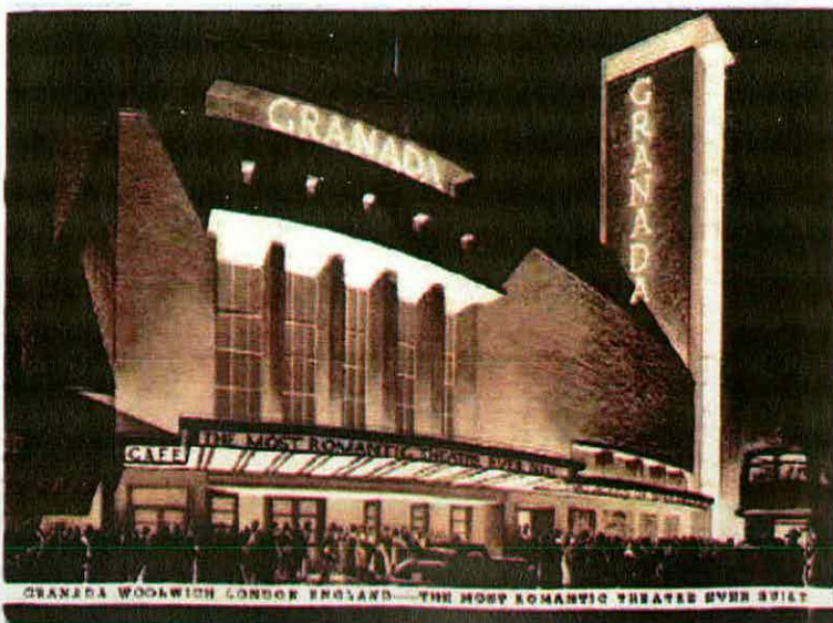
Figure 50 Touted as 'the most romantic theatre ever built' when opened in 1937, The Granada Woolwich survives as the most elaborate of the 19 purpose-built Granada cinemas apart from Tooting. Designed by C. Masey & R. H. Uren, it is the most 'modern' – and arguably most distinguished – of all the Granada cinemas. The thin advertising tower is reminiscent of Uren's contemporary work at Hornsey Town Hall. Listed II*
