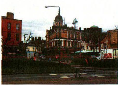
Figure 28 Beresford Square viewed from Plumstead Road, with the Ordnance Arms in the centre.
