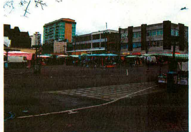
Figure 32 West side of Beresford Square: bar the narrow, two-storeyed Victorian survivor in the centre, the large buildings on this side are all products of mid-to-late 20 th -century redevelopment.
