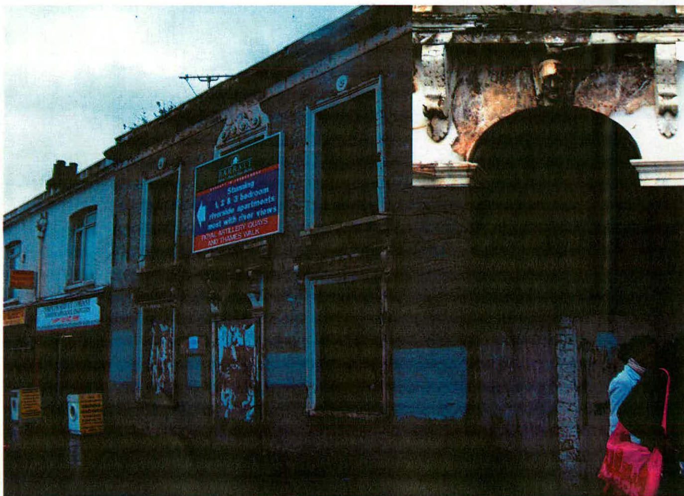
Figure 39 Until the 19 th century, Plumstead Road was essentially a country lane connecting Woolwich with Plumstead, a long-established and prosperous agricultural village further east. The great expansion of the Arsenal from the mid 19 th century saw the construction of properties along the south side to house both workers and military personnel. With frontages built hard up against the road, they stood directly opposite the high wall of the Arsenal. Survivors from this phase of intensive, ribbon development show that they catered for families across a relatively broad social spectrum, with some vaunting embellished façades, others far plainer. Despite recent shop conversions, and a generally run-down condition, much of this run of Victorian and Edwardian housing, shops and pubs survives. The Public Market, which replaced the Royal Arsenal Chapel (becoming the Royal Arsenal Reference Library) in the late 1930s (?) is of interest for its early 'Lamella' roof construction.
