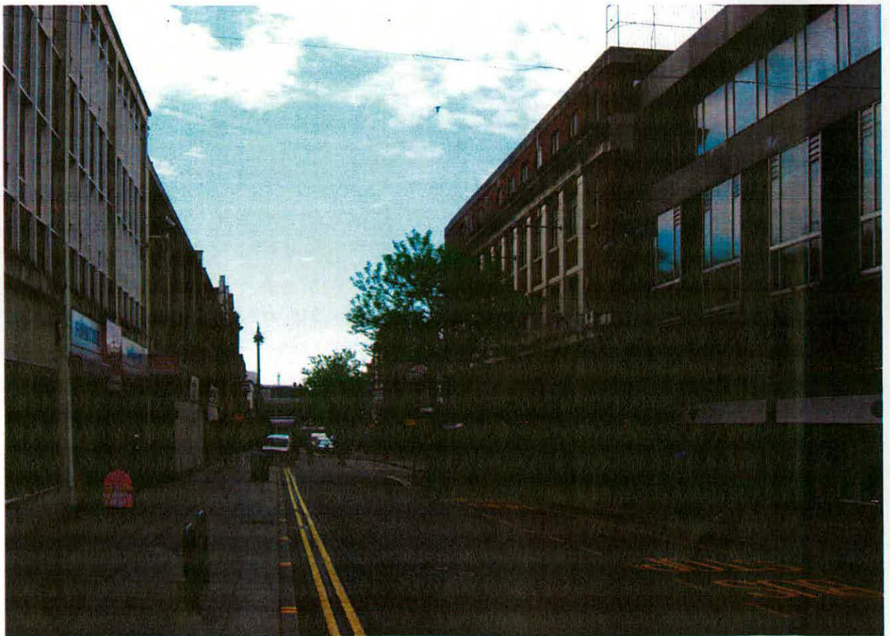
Figure 52 The north end of Hare Street, viewed from Powis Street. This end of the street has been redeveloped more extensively, and is home to second or third generation buildings largely erected in the inter-war or post-war years. The scale of these buildings is larger than those on the other end of the street, and modern materials such as concrete and aluminium impart a distinctly urban feel.
