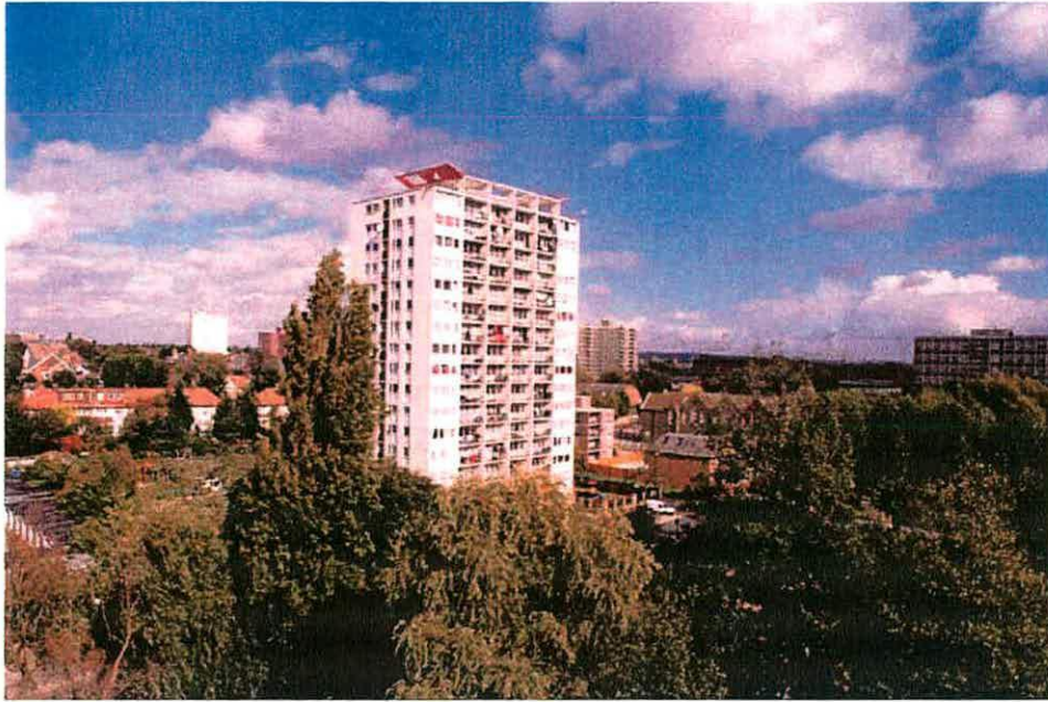
Fig. 56 - Jerome Tower from the southwest, 94 flats in 16 storeys, built 1962-3 as 34-220 Osborne Road (English Heritage, 2004, D. Kendall).
