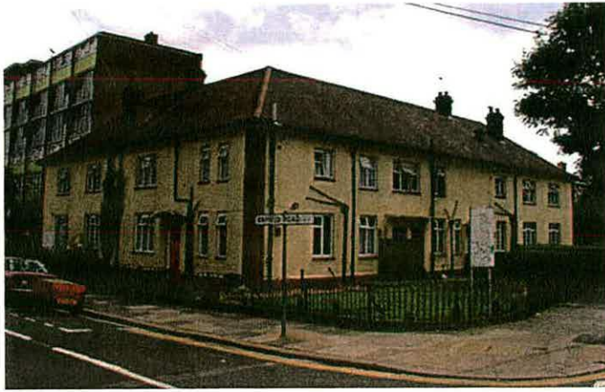
Fig. 22 - 363-371 Bollo Lane and 79-83 Enfield Road (formerly Enfield Road Flats), built in 1931 for Acton Borough Council (English Heritage, 2004), with contract drawing (Ealing Local History Centre).
