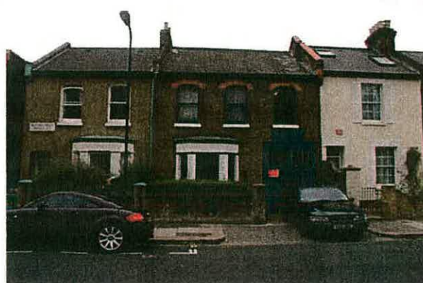
Fig. 9 - 67 Rothschild Road (to centre), house of the 1880s with workshop bay, occupied as William Everitt's laundry by 1887 (English Heritage, 2004).
