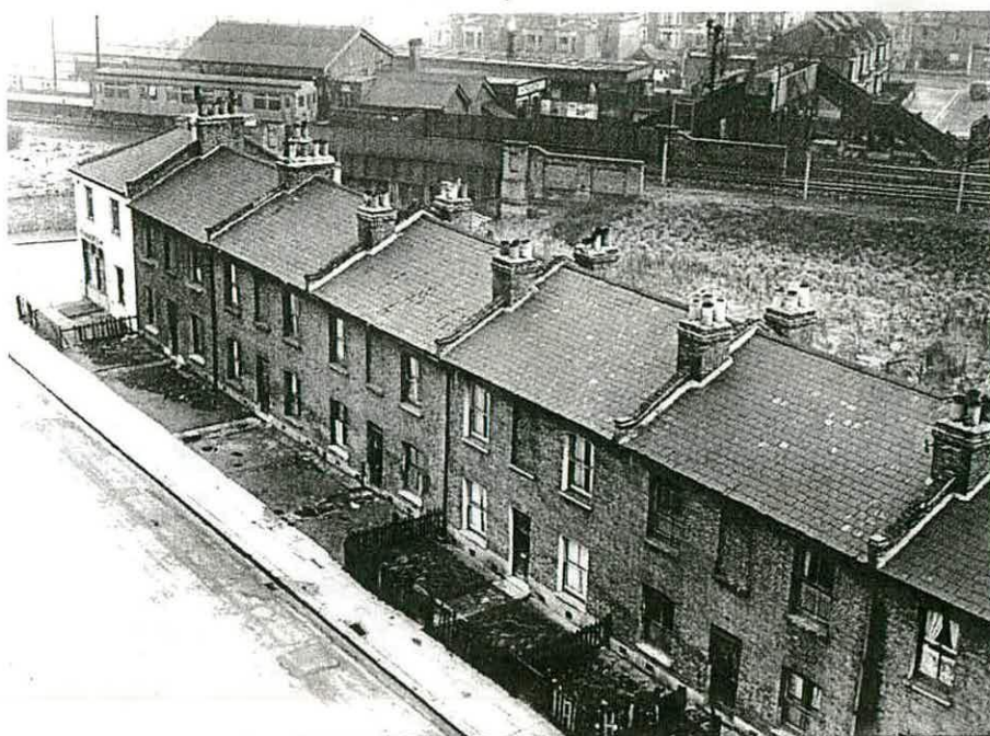
Fig. 6 - Junction Road (later Vincent Road), houses of c.1870 on the south side, photographed in 1954, just before their demolition. Note the 'ginny' shuttle train in the background at South Acton Station (Ealing Local History Centre).
