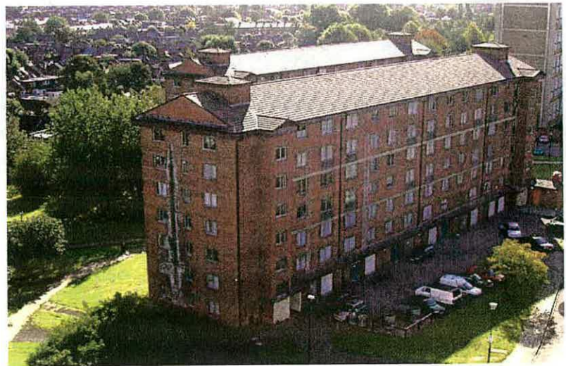
Fig. 68 - Ludlow Court (right), with Carisbrooke Court beyond, 54 flats each, built 1971-2 (English Heritage, 2004), with typical floor plan (below) (London Borough of Ealing).
