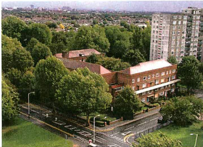
Fig. 29 - Bollo Court, 32 maisonettes in three ranges enclosing a courtyard, built by Acton Borough Council in 1949-50 incorporating an early application of central heating (English Heritage, 2004).
