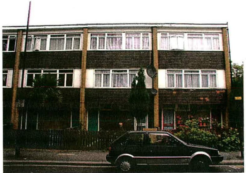
Fig. 47 - Three of a terrace of eight four-bedroom cross-wall-framed houses at 2-16 Enfield Road, built 1962-3 (English Heritage, 2004).
