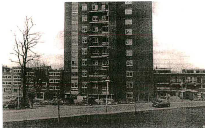
Fig. 69 - The building of 'Phase II' or the 'South Acton Extension' in 1978, showing Frampton Court (the tower block) and adjoining closes on the north side of Avenue Road (Ealing Local History Centre).
