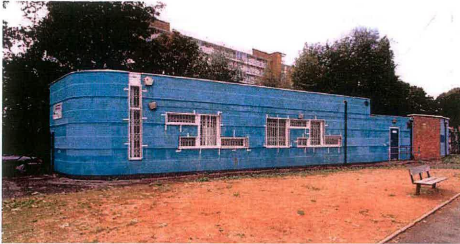
Fig. 52 - The Bollo Brook Play Centre (latterly Youth Centre), part of a garden and playground laid out in 1967-8 (English Heritage, 2004, D. Kendall).
