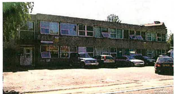
Fig. 51 - Avenue House, Avenue Road, health clinic built by Middlesex County Council in 1963-4, Douglas Stephen and Partners, architects (English Heritage, 2004).
