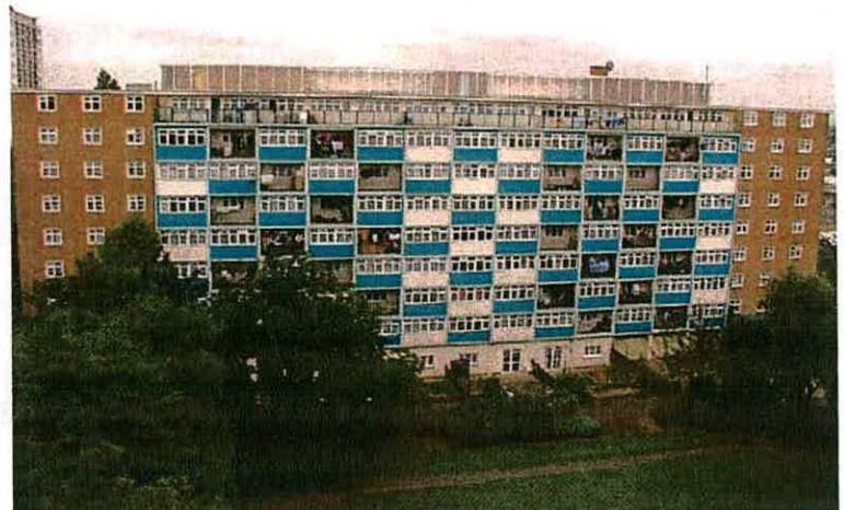
Fig. 39 - Meredith Tower from the west, originally 58 flats, showing the reinforced-concrete box-frame construction, with part of 'The Green' in the foreground (English Heritage, 2004)
