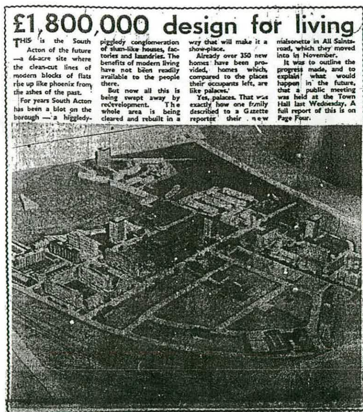
Fig. 45 - The scheme for the South Acton Comprehensive Development Area as revised in 1961 with an article from The Acton Gazette.
