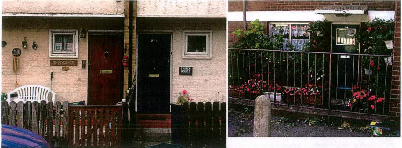
Fig. 78 - Outward personalisation of homes, through the naming of houses, on Osborne Road, and floral display, in the 'red-brick' area (English Heritage, 2004).
