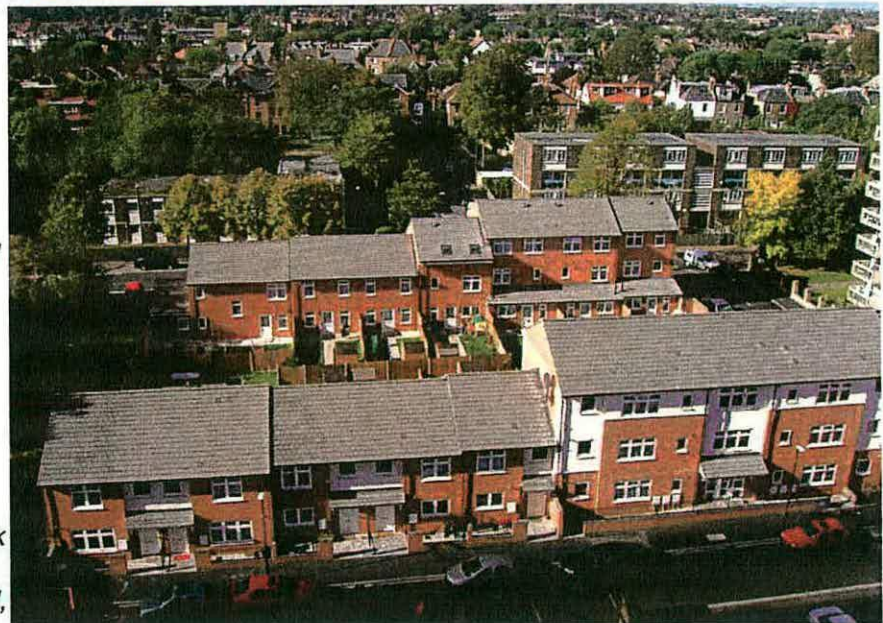
Fig. 85 - 'Phase I' of South Acton's regeneration (top to bottom): Newport Road with Appleby Court; 45-53 Brouncker Road; and looking down on Hope Gardens and Park Road North from the east, with Arundel Court, Glamis Court and the Mill Hill Park Estate beyond (English Heritage, 2004, D. Kendall, top and centre).
