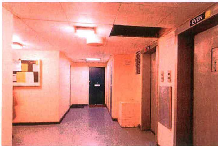
Fig. 74 - Shared indoor space in Harlech Tower, showing lifts serving alternate floors (English Heritage, 2004, D. Kendall).
