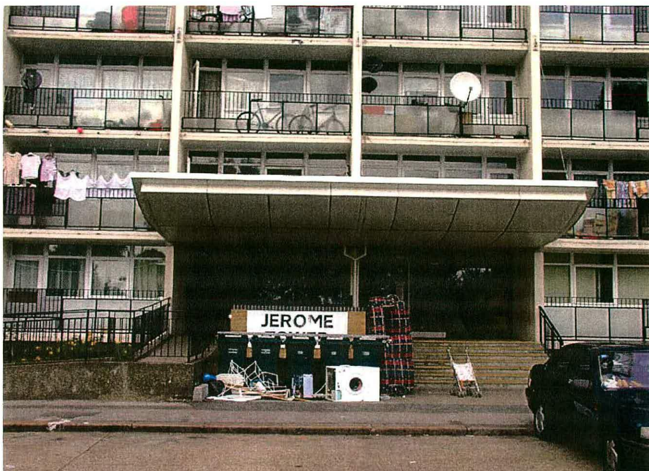
Fig. 82 - Entrance to Jerome Tower, built 1962-3, disabled ramp added 1972, canopy added 1991-2 and further altered c.2000 (English Heritage, 2004).
