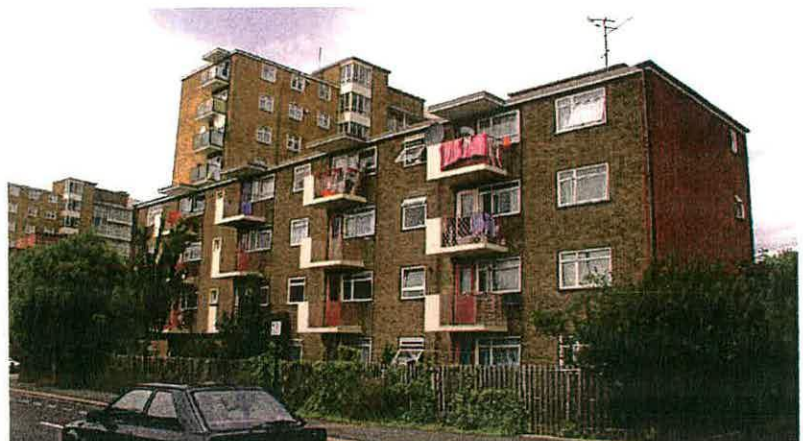
Fig. 40 - Chesterton Court from the south (English Heritage, 2004)
