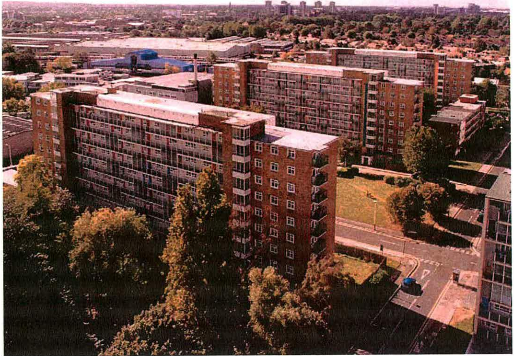
Fig. 38 - The former Hanbury Estate from the northeast, 'the Three Sisters' (Grahame, Meredith and Conrad towers) and their glazed access balconies being prominent, built 1955-9 (English Heritage, 2004, D. Kendall).
