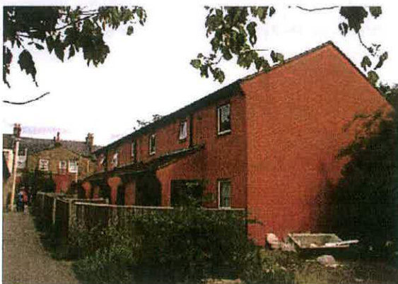
Fig. 79 - 1-6 Telfer Close, six houses for disabled tenants, built c. 1990 for the London Borough of Ealing (English Heritage, 2004).
