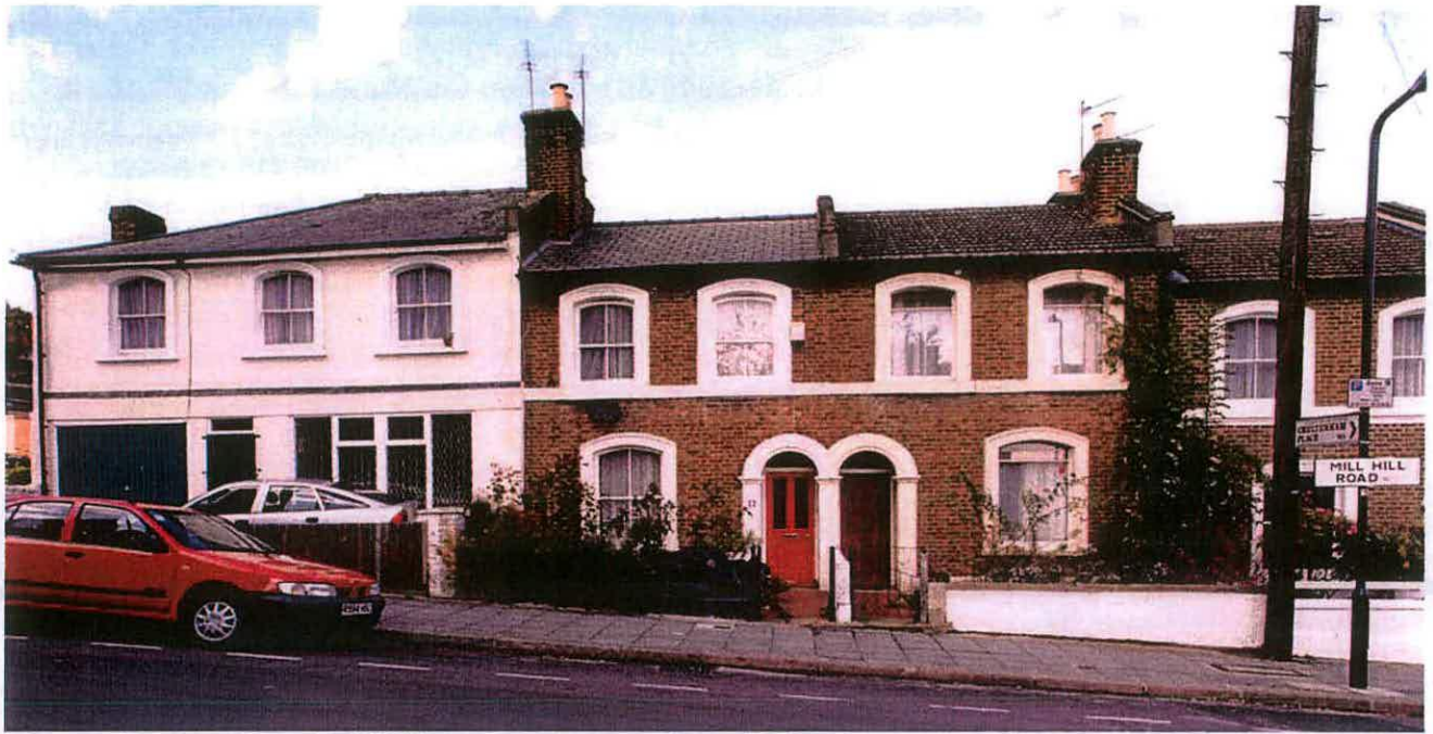
Fig. 3 - Nos 8-14 (even) Mill Hill Terrace, houses of c.1870 (English Heritage, 2004, D. Kendall).
