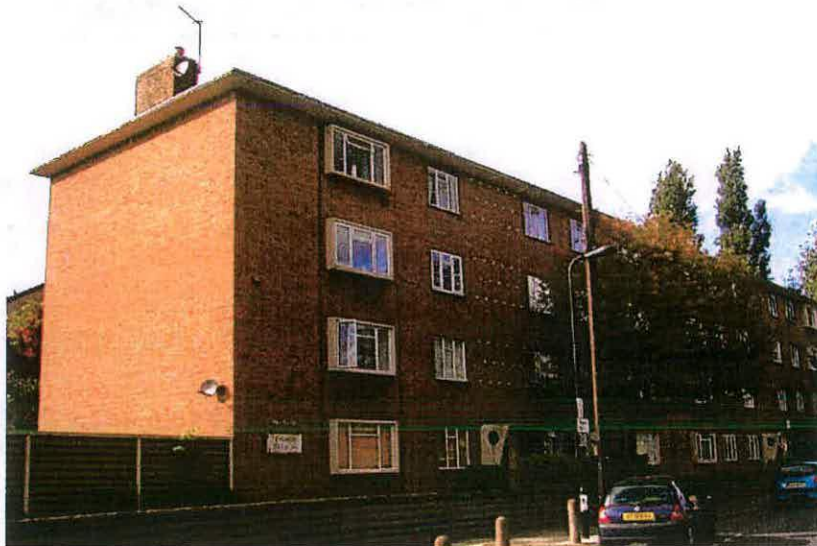
Fig. 37 - 1-15 Church Path, Acton Borough Council flats, 1952-4, one of eight blocks built in redevelopment of bomb sites south of the North London Line railway (English Heritage, 2004).
