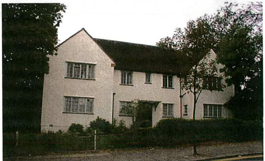
Fig. 19 - Helen House, Gunnersbury Lane, one of five blocks, each of eight flats, built for the United Women's Homes Association in 1927-8, Thomas Garrett and Son, architects (English Heritage, 2004).
