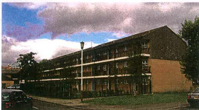
Fig. 72 - Neville Close, Acton Lane, built 1977-9 for the Borough of Ealing (English Heritage, 2004).
