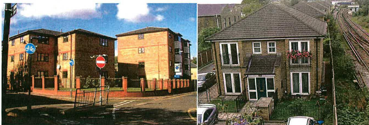
Fig. 83 - The Grange, 114 Avenue Road (left), 17 flats on what had been a laundry site, and Kingswood Terrace (right), 20 flats in five rail-side blocks, both private developments of the 1990s (English Heritage, 2004).
