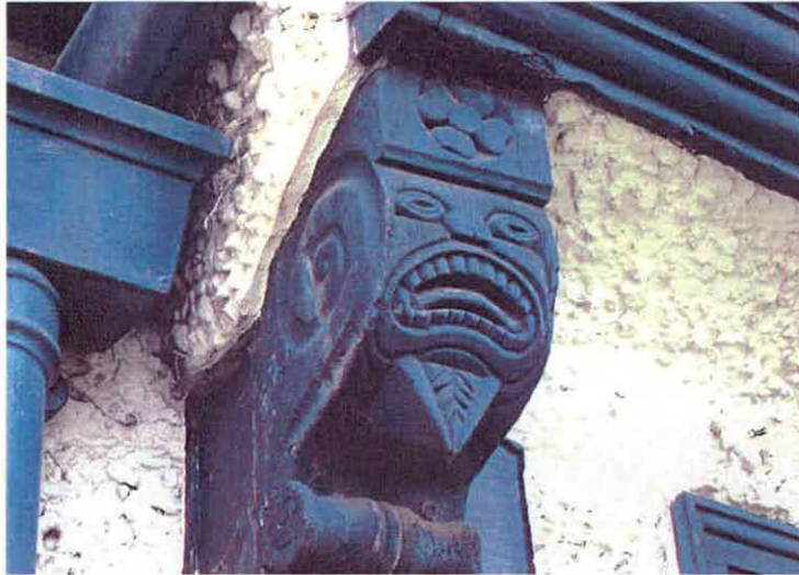
Figure 5 Carved timber bracket supporting first floor jetty of north cross wing of main house. The scroll ornament seen at the base of the bracket is also a feature of the brackets supporting the first floor ceiling over the west (original front) bay of the North Range.
