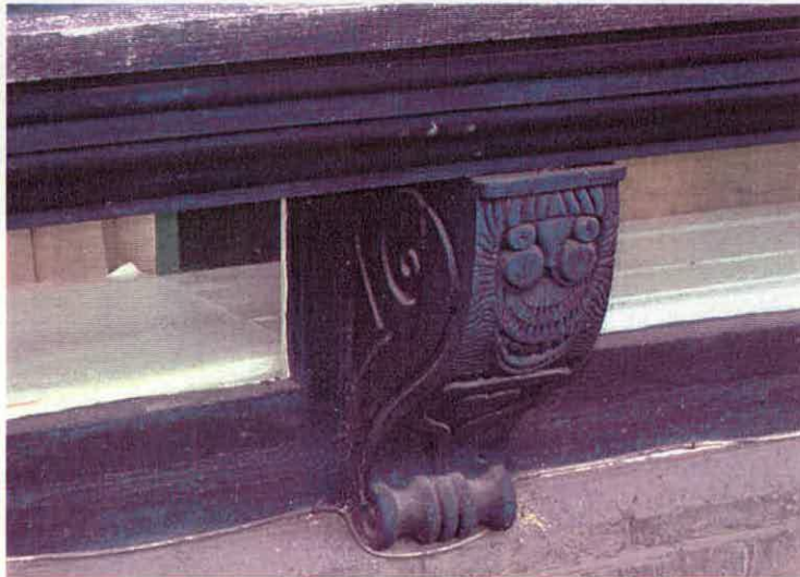
Figure 6 Carved timber bracket supporting projecting front ground floor window of north cross wing of main house.
