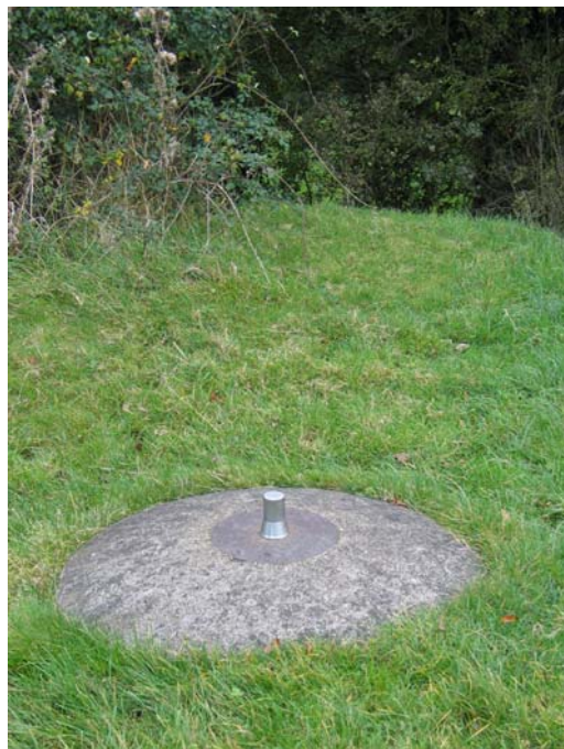
Figure 20 The mounting for the spigot mortar
