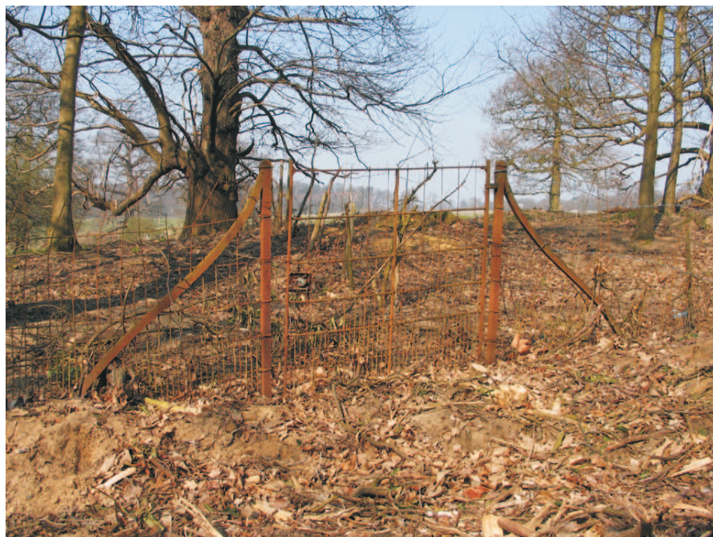
Figure 22 An original iron gate in Repton’s invisible fencing, on the western boundary of the North Pleasure Grounds, giving access into West Park (Paul Pattison)
