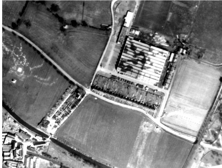
Figure 10 Extract from a RAF vertical photograph showing the Military camp on the left and the camouflaged ball-bearing factory in 1947
