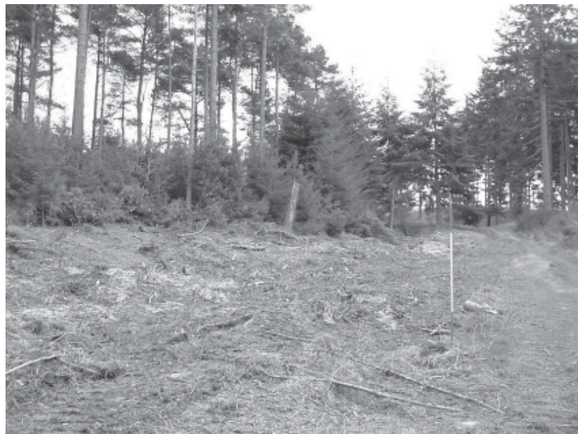
Recent shrub clearance showing damage to the agger
