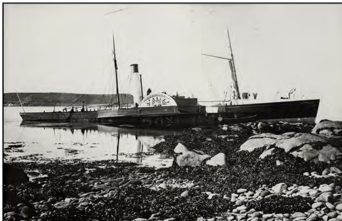
Fig 40 SS Earl of Arran , a steam packet which ran a service from Penzance to Scilly, grounded on Nornour in 1872. A small part of her boiler is still visible at low water (photo: © Gibson Collection)
