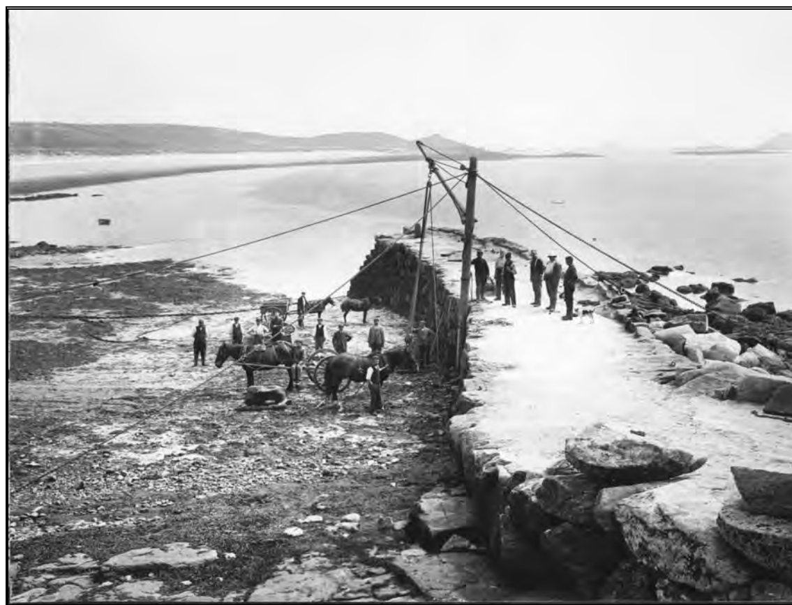
Fig 11 Higher Town quay under construction in c1888 (photo: © Gibson Collection)
