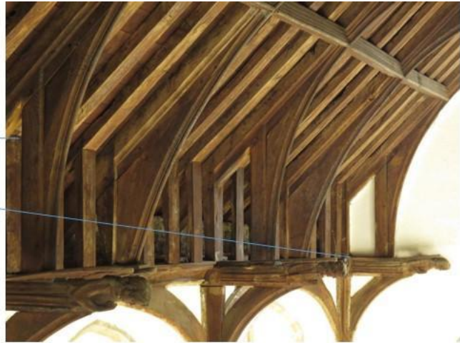
Left: nave eaves void areas to be boxed-in (north and south sides) circled in blue. View from the chancel.
