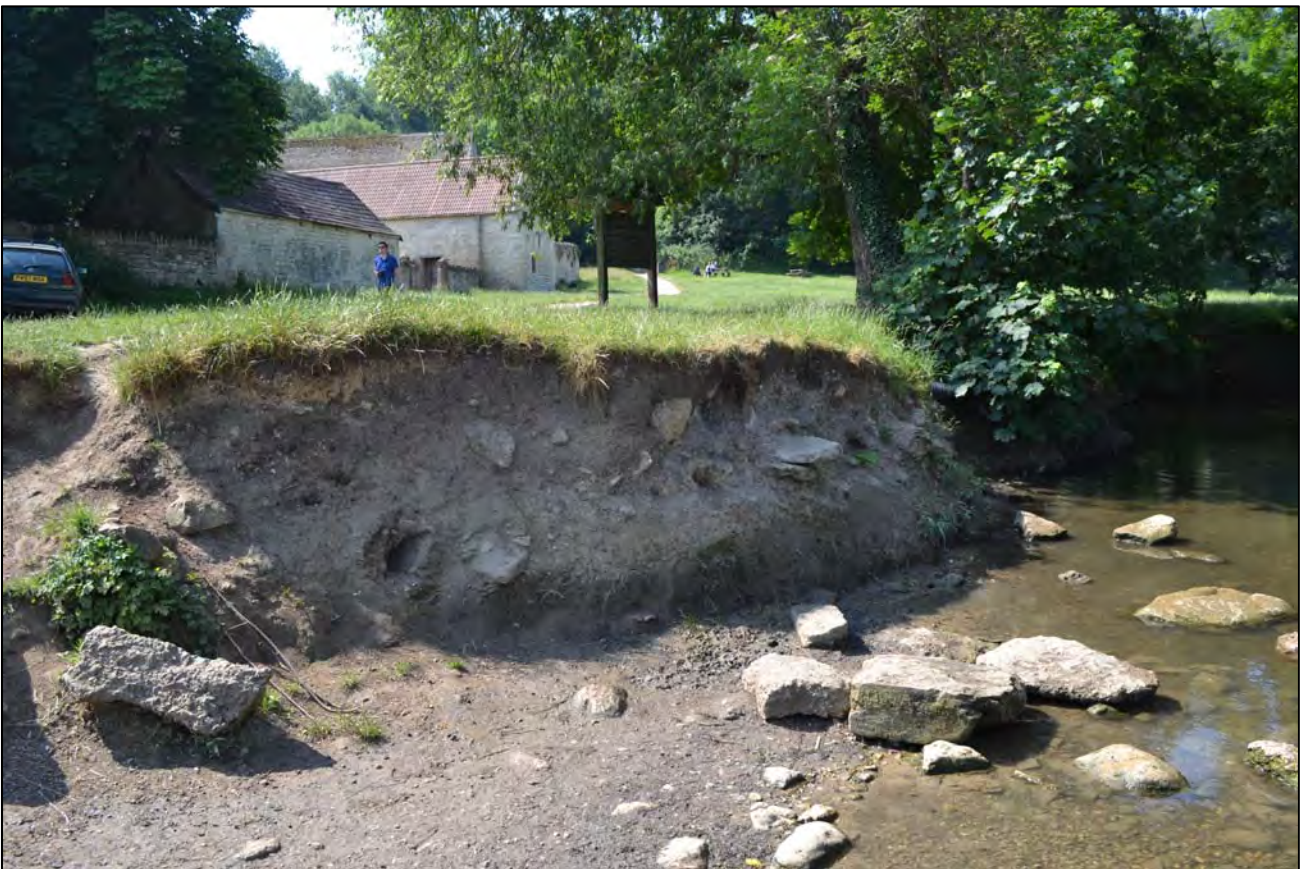
Plate 8: Eroding stonework at ford just outside scheduled area, Barton Bridge, Bradford-on-Avon (© Antony Firth/Fjodr)
