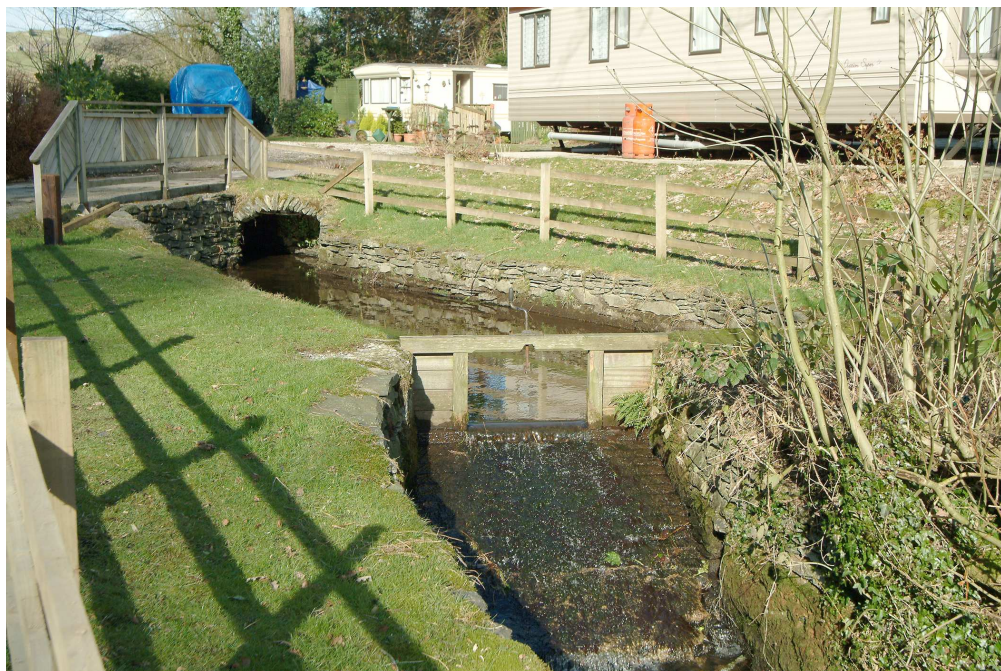
Figure 16. Widened beck channel and sluice to the north west of the former lower pond. (NMR: DP003418)
