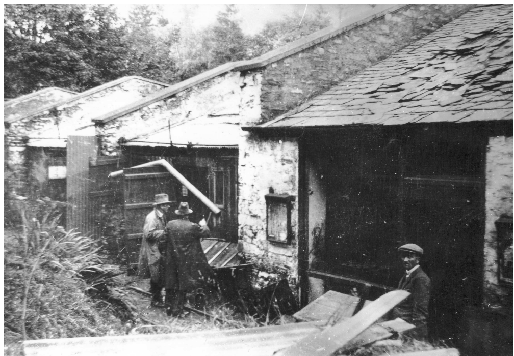
Figure 24. Incorporating mills 4-6 (left) and the main engine house (right) after the explosion in September 1928, looking north. (NMR: Patterson Collection)
