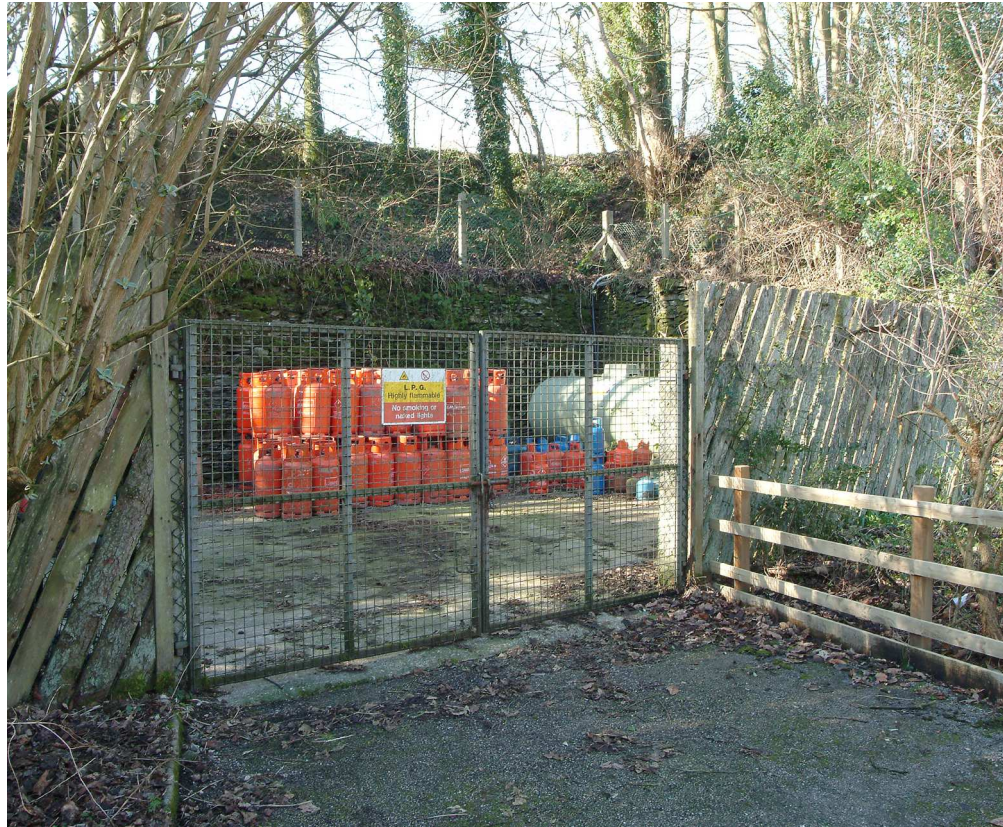
Figure 21. Site of the second mixing house looking west. (NMR: DP003394)
