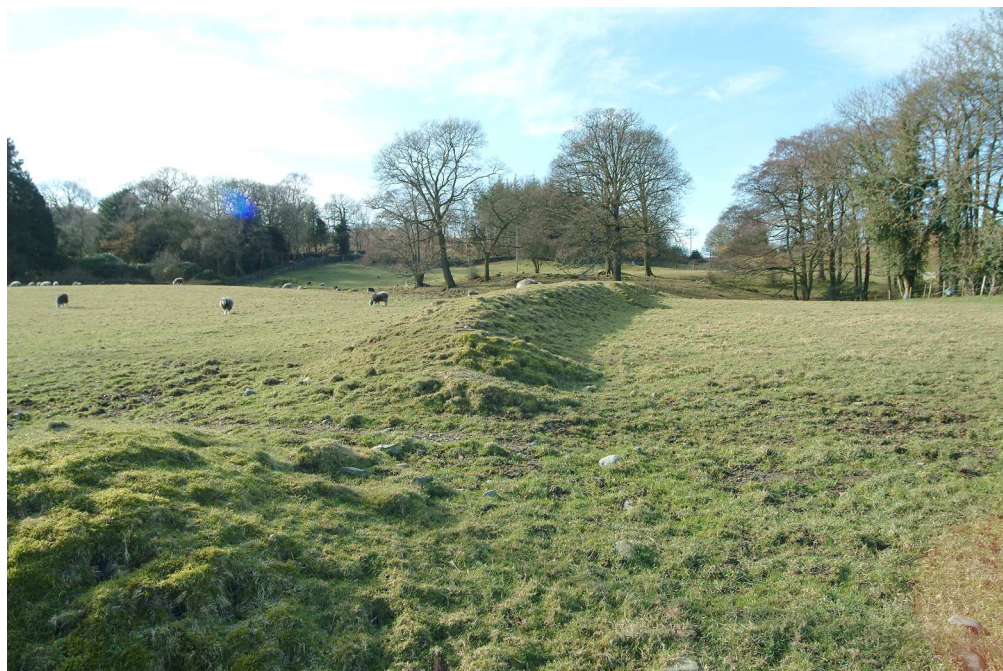
Figure 11. Upper part of flue (west of the farm track) from the boiler house. Looking west. (NMR: DP003389)
