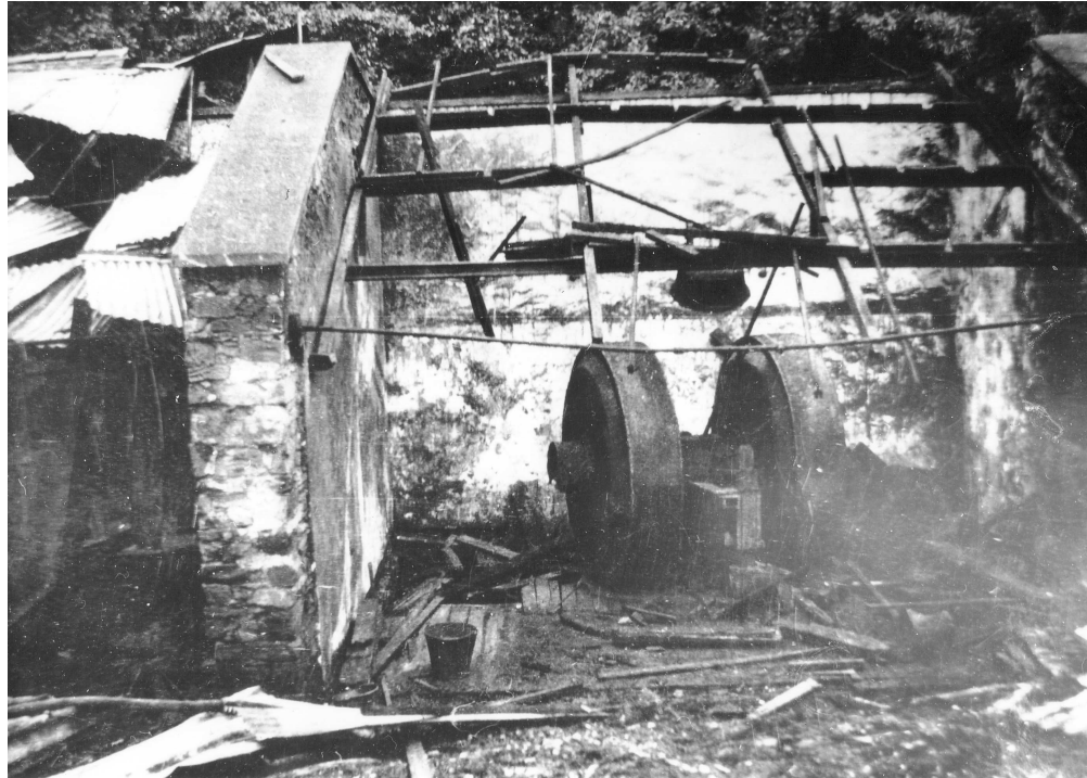
Figure 25. Mill chamber 2 and its edge runner mill after the explosion in September 1928, looking east. (NMR: Patterson Collection)
