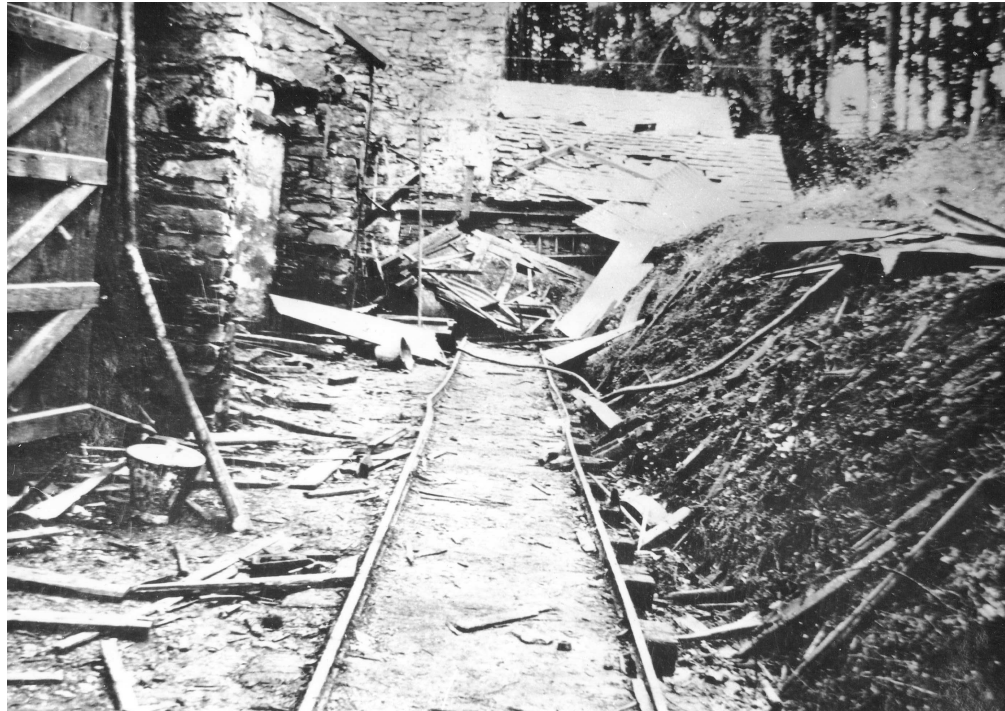
Figure 23. Incorporating mills 3-1 (left) and the north (blast) wall and roofs of the building range immediately to the south. Taken from the north after the explosion at the mills in September 1928. (NMR: Patterson Collection)
