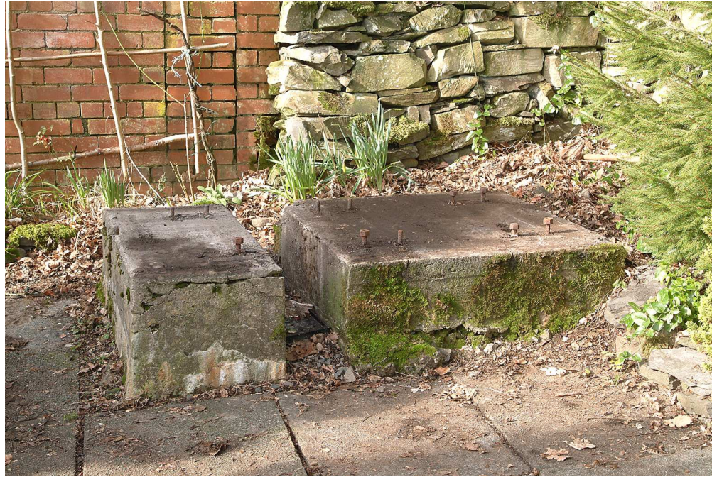
Figure 32. Machine beds on site of the probable reel house, from the east. Modern table top removed for photograph and blocked slot in end wall of electric motor house visible. (NMR: DP003375)
