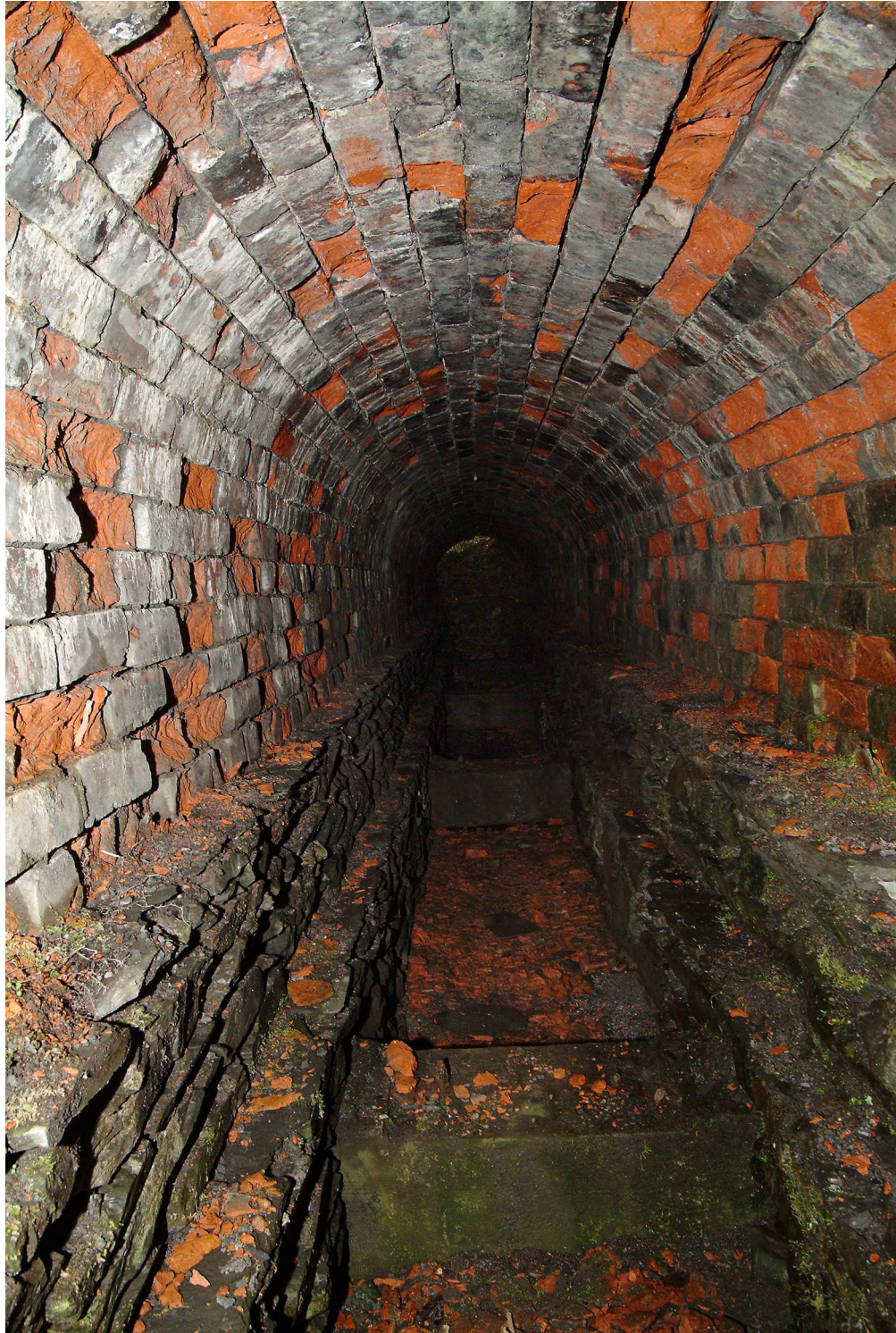
Figure 46. Drive shaft tunnel to second mixing house, looking south. (NMR:DP003534)
