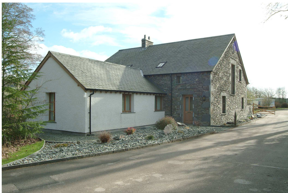
Figure 52. Caravan park manager's new house from the north west. Single storey part to left incorporates north end of weigh office and store. (NMR: DP003426)
