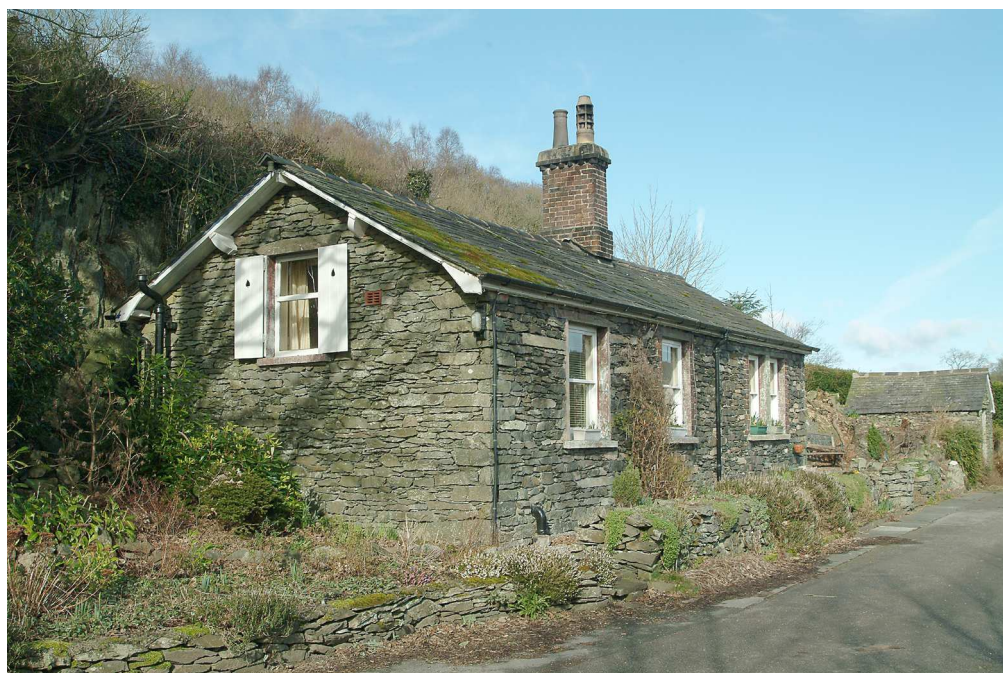
Figure 55. Small office at the southern entrance of the works (near Pool Bridge), from the south. (NMR: DP003377)
