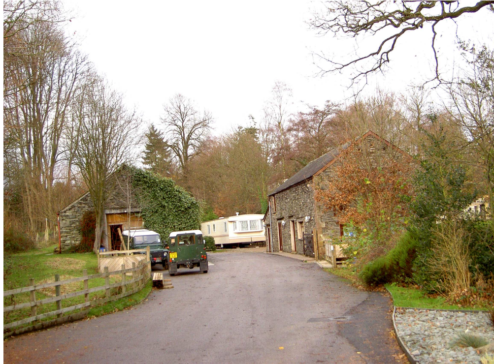
Figure 18. Saltpetre house (left) and store and stable (right) from the south. (Christopher Dunn, November 2003)
