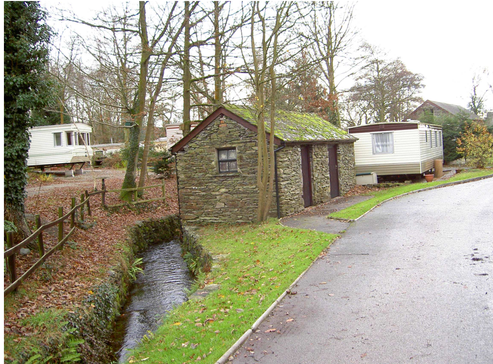
Figure 49. Oil store from the north west. The store and stable (right) is visible in the background. (Christopher Dunn, November 2003)
