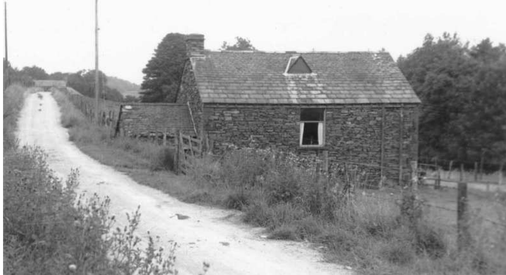
Figure 40. The watch house in 1958, from the south. (Ron Mein Collection, copyright reserved)
