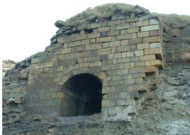
Figure 33. Photograph of the arch adjacent to the steps down to Hummersea Beach. This may be the remains of a kiln or boiler, possibly associated with the building shown in 19th century photographs.
