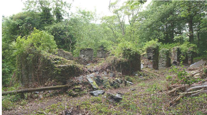
Fig 67. The ruins of the glazing house, viewed from the south following felling of standing trees. (NMR DP006445)
