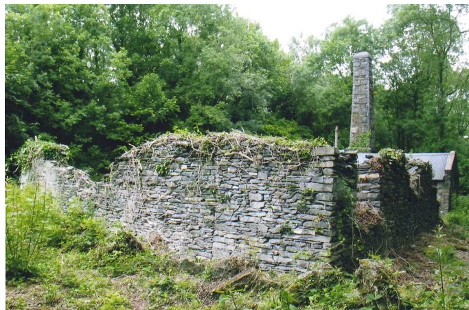
Fig 74. The lower stove, viewed from the south-west after vegetation clearance. (Ian Goodall, 2004)
