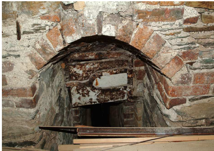
Fig 31. The stoking area and fire-box door to furnace no. 5. (NMR DP003508)
