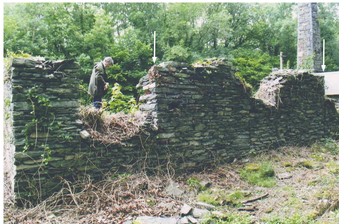
Fig 75. The south-east wall of the lower stove. The corners of the 1911 stove house are arrowed. (Ian Goodall, 2004)
