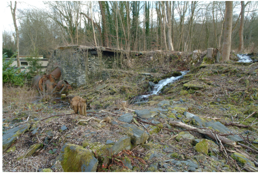
Fig 101. The sawmill and turbine header-tank at the end of the sawmill lead, viewed from the west. (NMR DP003445)
