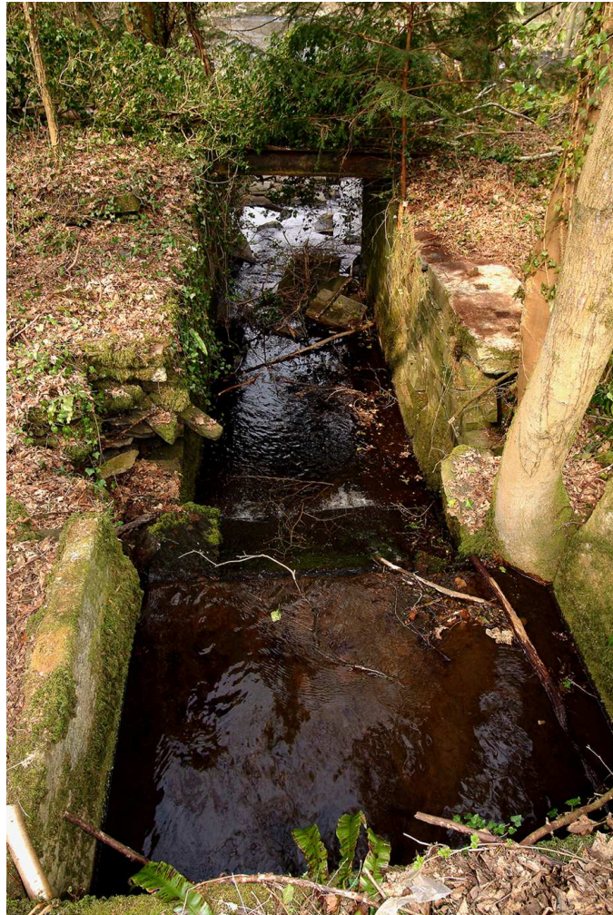
Fig 21. The reel-and-glaze- house leat and waterwheel-pit from the south-east. Note the steel girders (one obscured by the fallen tree) for the tramway bridge. (NMR DP003484)
