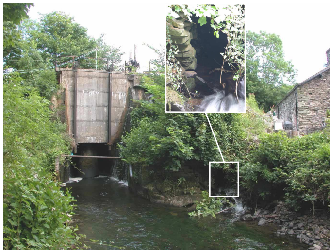
Fig 12. The outfall of the covered section of the ironworks headrace (shown in detail at inset) back into the main tailrace. The modern hydro-electricity station is visible at left of frame. (Christopher Dunn, July 2005)
