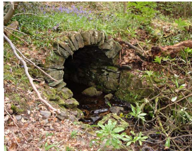
Fig 24. The outfall of the tailrace from the lower corning house. (NMR DP003524)
