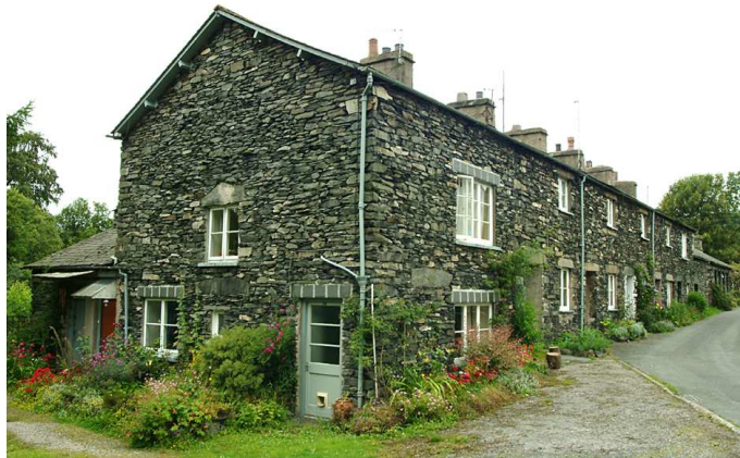
Fig 122. The front elevation of nos. 12-16 Low Wood. (NMR DP006429)
