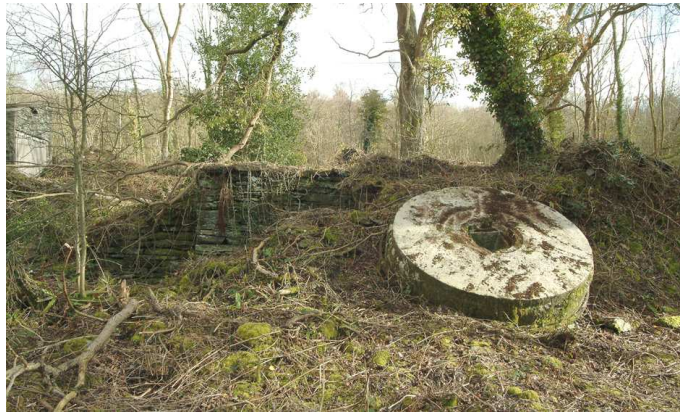
Fig 44. Incorporating mill 38 viewed from the north-west. The more ruinous wall at left of frame marks the rear edge of the waterwheel-pit, the stub wall next to it the division between wheel-pit and part-basement. (NMR DP003436)
