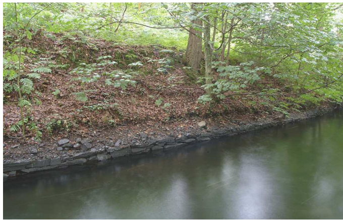
Fig 20. The original stone-lining to the east side of the headrace between the reel and glaze house and lower stove. The walling is now only visible when river levels are low; the modern winter water level in the headrace is shown by the scour mark in the leaf litter on the bank above the wall. (NMR DP006451)
