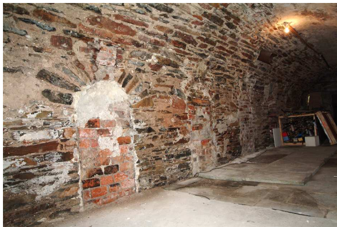
Fig 29. The boilerman's passage from the south-east, showing furnaces nos. 1-3 with no. 4 just visible behind the crates. (NMR DP003505)
