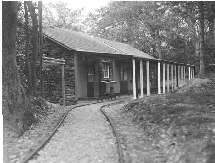
Fig 66. The glazing house as reconstructed in 1929, viewed from the south. (Patterson Collection, ©English Heritage.NMR)
