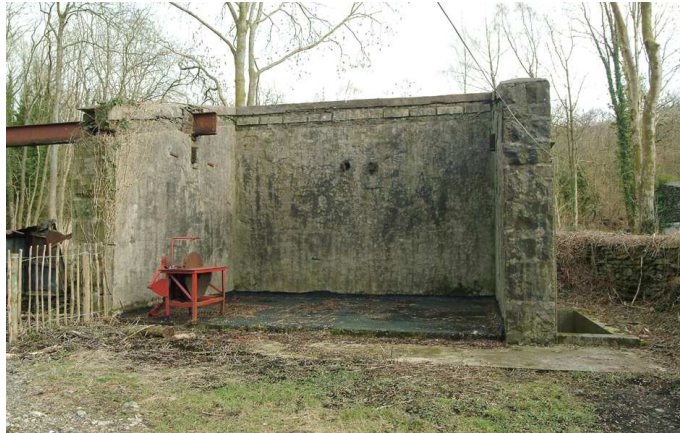
Fig 48. Incorporating mill 35 mark II, viewed from the north-west. (NMR DP003442)
