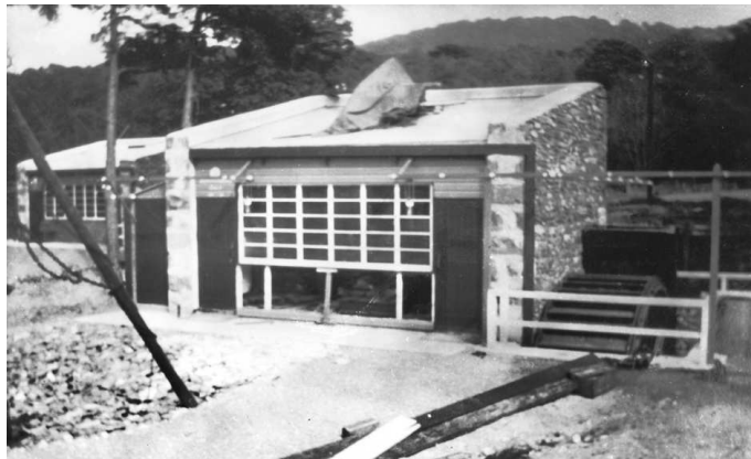
Fig 49. Incorporating mill 30 mark II, viewed from the west in 1929. (Patterson Collection, ©English Heritage.NMR)
