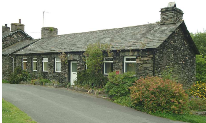
Fig 105. Cooperage no. 4 from the north-east, now a house called 'The Coopers'. (NMR DP006426)
