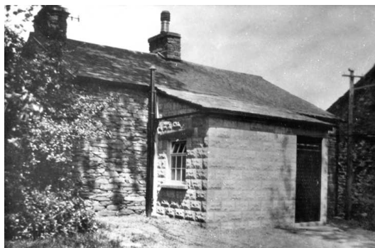
Fig 106. The addition to the north-east block of offices within the former iron-ore store, in 1929. (Patterson Collection, © English Heritage.NMR)
