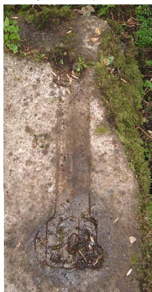
Fig 64. Imprint of one of the line-shaft supports in the floor of the belt-drive house attached to the lower corning house mark IV. (NMR DP006444)
