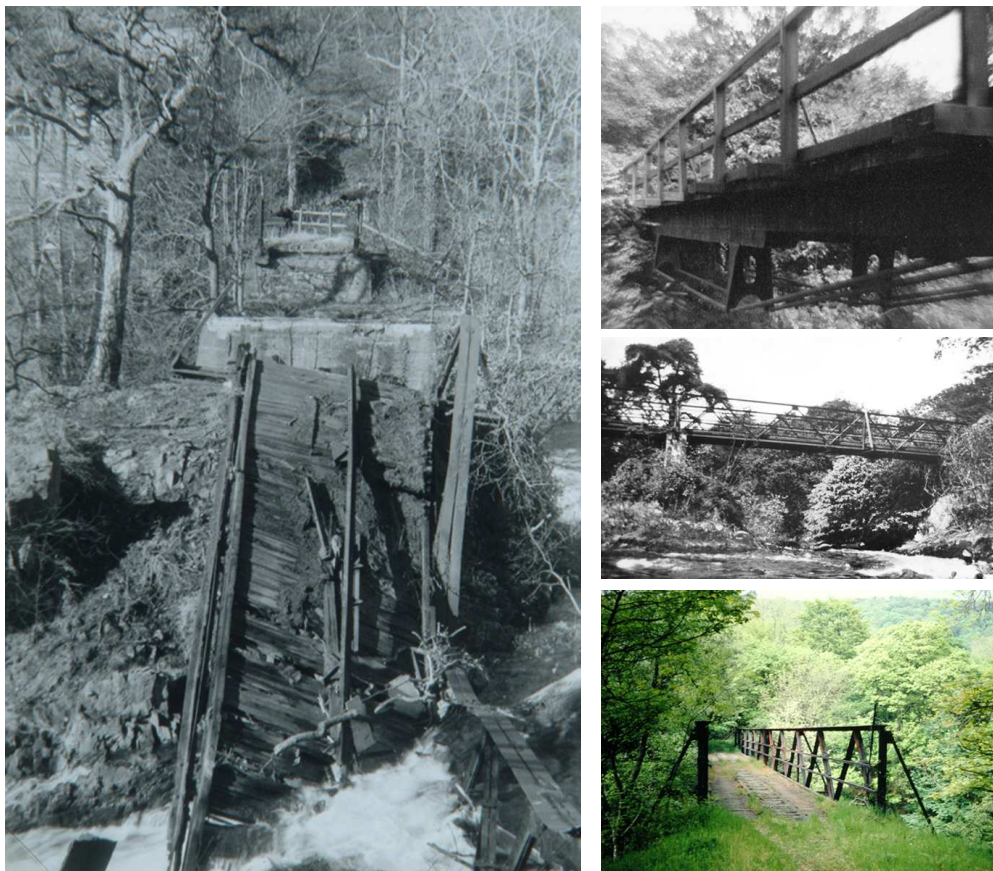
Fig 112. Four views of the tramway bridges at Bleaberry Holme. Clockwise from top right: a and b. The original timber bridge and the new girder bridge which replaced it in 1929. (Patterson Collection, © English Heritage.NMR). c. The southern end of the girder bridge in June 1966. (Davies-Shiel Collection, copyright reserved) d. The collapsed girder bridge viewed from the south in the 1970s. (Robert Harvey Collection, copyright reserved)
