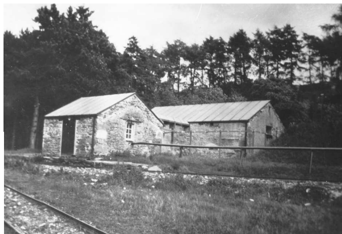
Fig 80. The rear of the higher stove house and heater house viewed from the west following reconstruction in 1929. (Patterson Collection, ©English Heritage.NMR)
