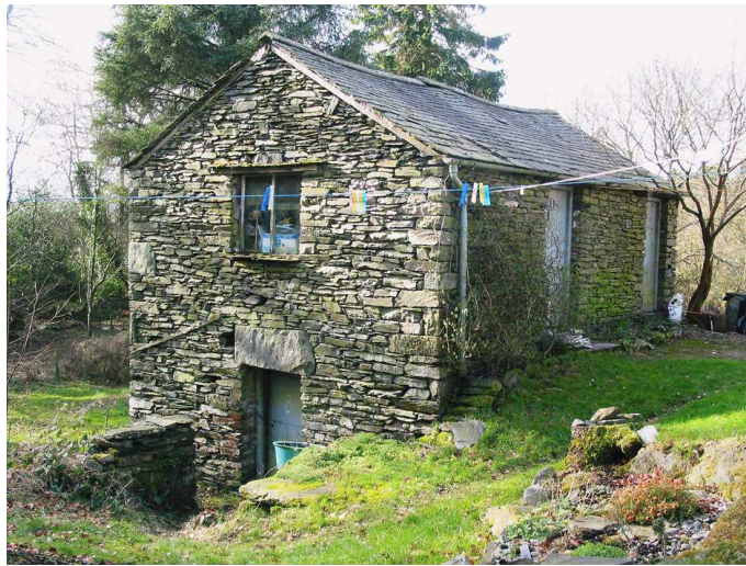
Fig 127. Peat houses serving nos. 7-10 Low Wood. (Simon Taylor, March 2004)
