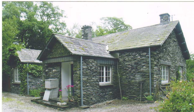
Fig 94. The former Busky magazine now converted into a private dwelling, 'Busca'. (Ian Goodall, 2005)
