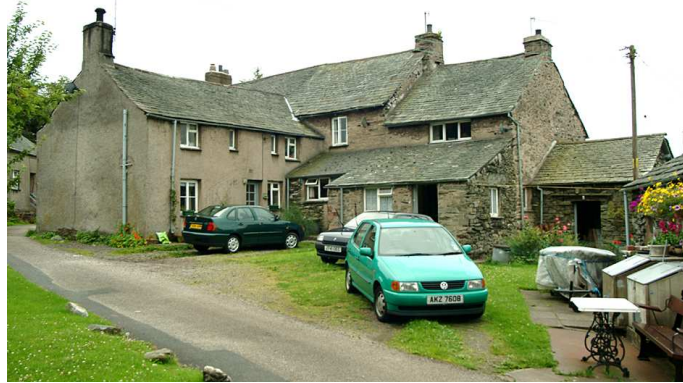
Fig 117. The north elevation of no. 4, and the rear elevation of nos. 1 and 2, Low Wood. (NMRDP006436)
