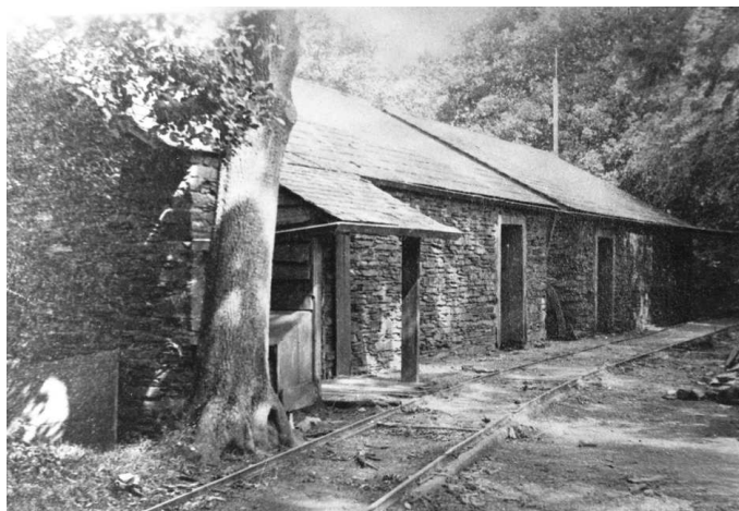
Fig 65. The front of the glazing house, photographed from the south in August 1928 prior to reconstruction by ICI. (Patterson Collection, ©English Heritage.NMR)
