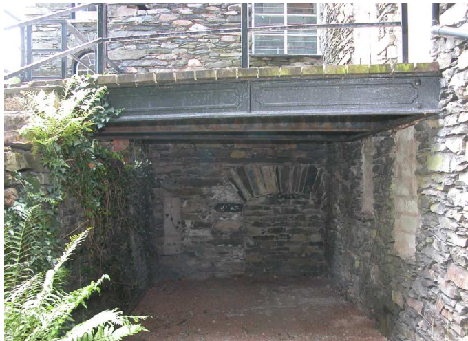
Fig 37. View beneath the raised path to the saltpetre refinery, showing the blocked doorway and window at the end of the boilerman's passage. (Christopher Dunn, July 2005)
