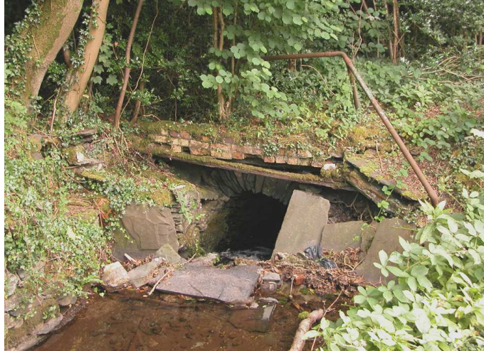
Fig 11. The entrance to the covered section of the ironworks headrace leading to the blast furnace. (Christopher Dunn, July 2005)
