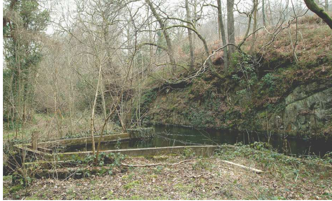
Fig 19. The rock-cut upper section of the gunpowder headrace at its junction with the subsidiary leat to the reel and glaze house. (NMR DP003489)
