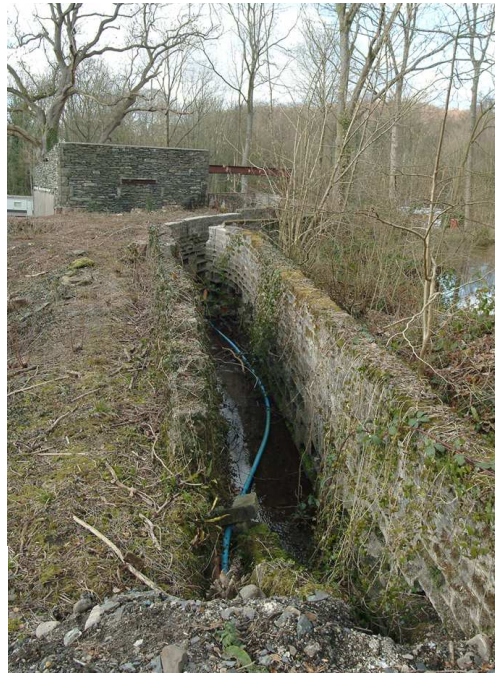
Fig 57. The relined leat to incorporating mill 35 mark II. (NMR DP003441)
