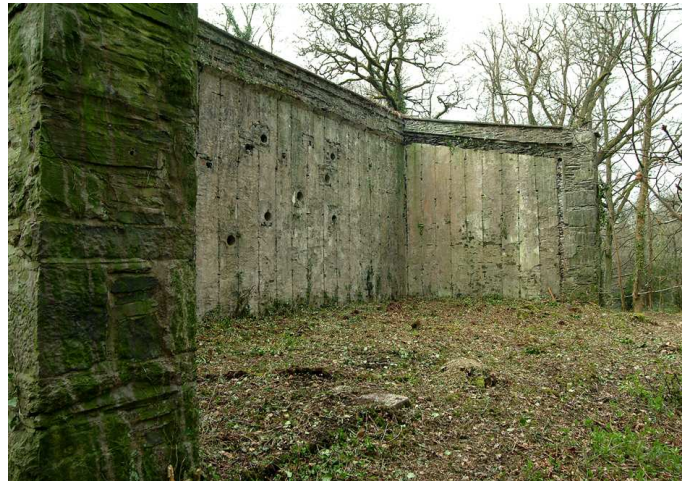
Fig 61. The interior of the lower corning house mark IV, viewed from the north-east. (NMR DP003475)
