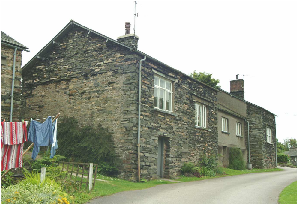
Fig 16. The iron-ore store from the north-east. (NMR DP006441)
