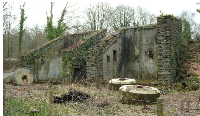
Fig 39. Incorporating mills 25/26 viewed from the north-west following clearance of vegetation from the fabric. Note the higher walling on the west side of mill 25. (NMR DP003470)
