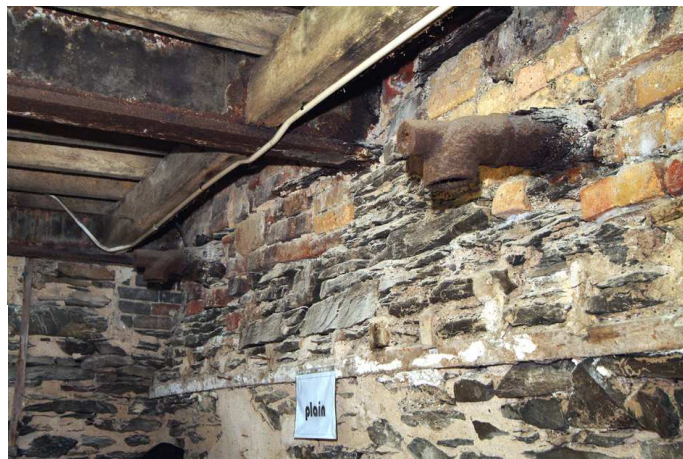
Fig 34. The taps for draining the boiling vats above furnaces nos. 5 and 6 into the filters. (NMR DP003504)
