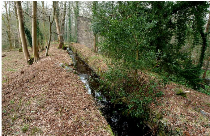
Fig 22. The final section of the leat to the lower corning house, looking south-west towards the corning house (visible at centre frame). (NMR DP003477)
