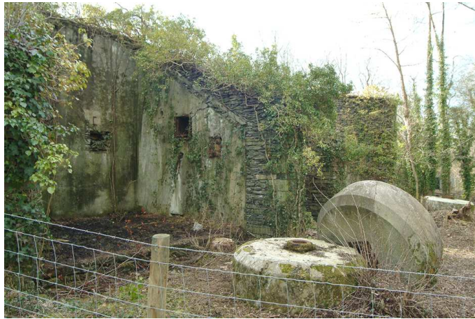
Fig 40. Incorporating mill 26 from the east before clearance of vegetation from the fabric. (NMR DP003433)
