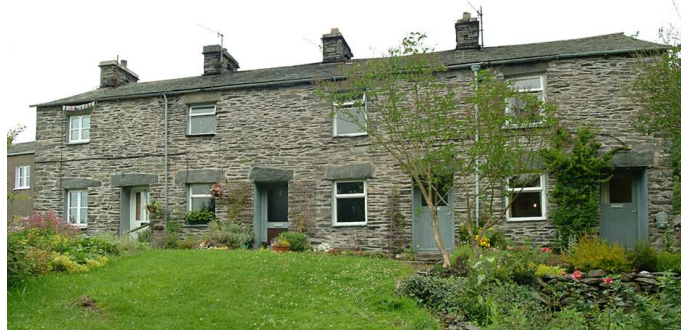
Fig 120. The front (south-west) elevation of nos. 7-10 Low Wood. (NMR DP006432)
