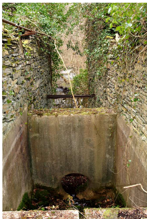
Fig 71. Two views of the glazing-house waterwheel-pit: a (left) looking north-west down the pit, showing the cross-wall for the turbine supply-pipe. (NMR DP003480) b (right) looking south up the pit, showing the joists for the turbine and the imprint of the discharge-pipe. (NMR DP006449)
