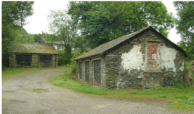
Fig 103. Cooperages nos. 1 (at right of frame) and 2 (left of frame), viewed from the north; both are now converted into garages. Cooperage no. 3 is just visible in the background. (NMR DP006425)
