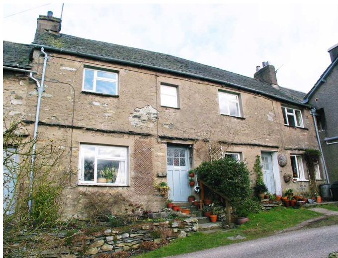
Fig 115. The front elevation of nos. 2 and 3 Low Wood. (Simon Taylor, March 2004)
