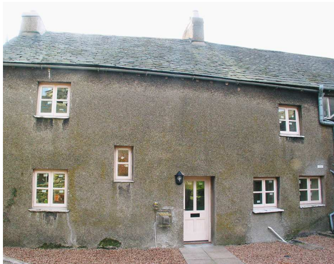
Fig 116. The rear elevation of no. 5 Low Wood. (NMR DP006436)
