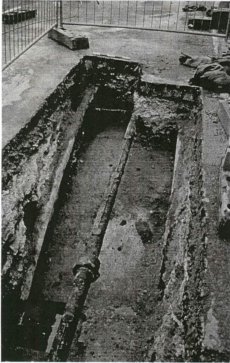
Side span, TP2 from SW
