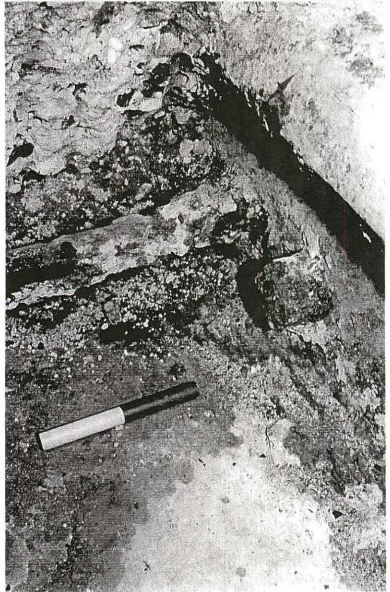
Main span tie bars SE side
