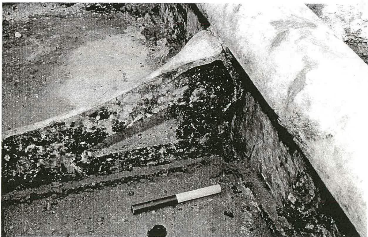
Main span crossbeam SE end
