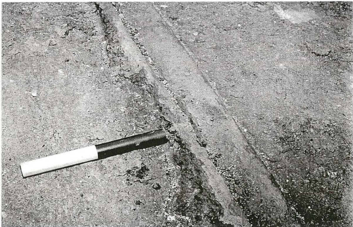
Main span, wedge in joint of soffit plates
