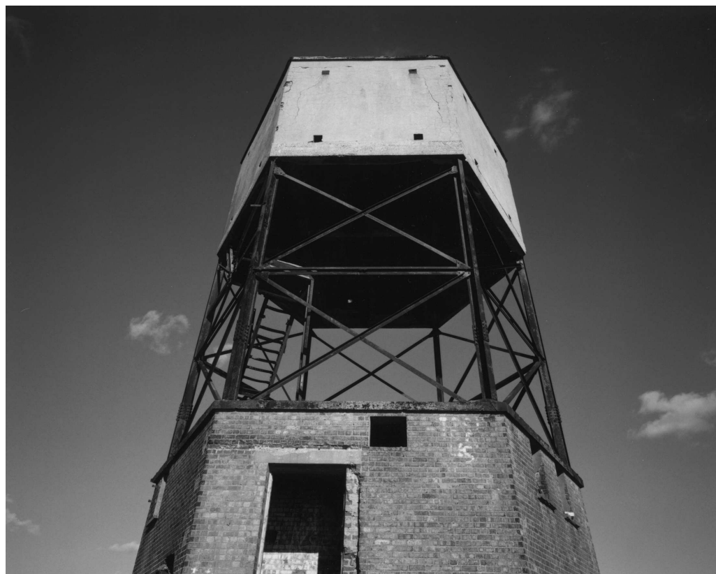
Figure 19 The Second World War radar tower at Coalhouse Point. Note the unusual raising of the upper level, probably necessitated by the low lying location on the mudflats (©Crown copyright NMR: AA/031291)
