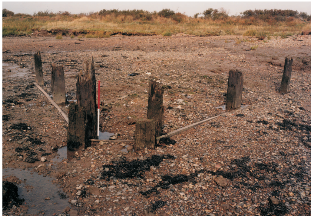
Figure 17 The probable remains of one of the sluices which during the 19th century controlled the flow of water between the river and the salt marsh (©Crown copyright NMR: AA/046708)
