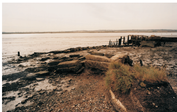
Figure 18 Remains of one of the two Defence Electric Lights at Coalhouse Point (©Crown copyright NMR: AA046711)
