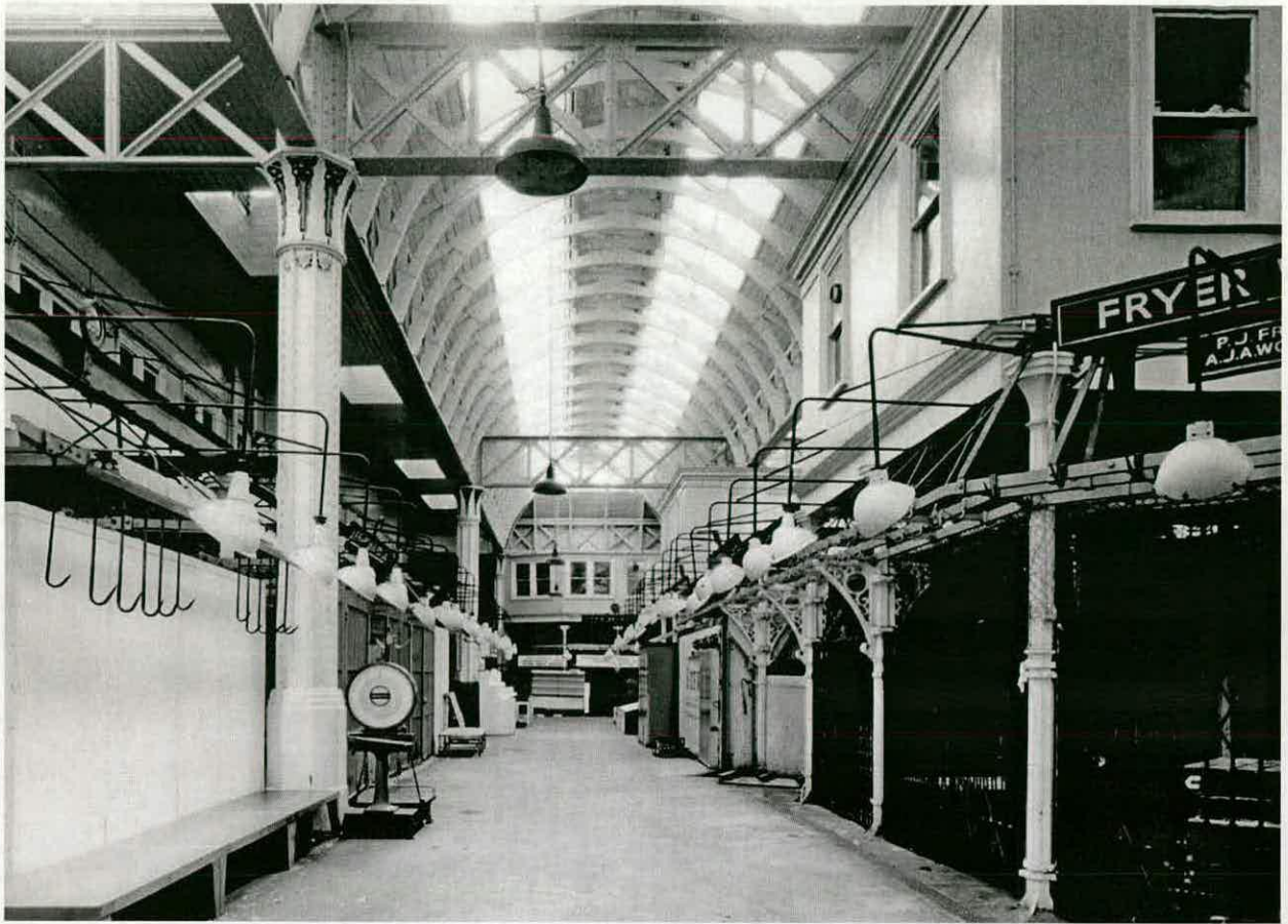
Fig. 9 – Interior of the General Market, view from west showing the Phoenix columns (BB87/7248, ©Crowncopyright.NMR).
