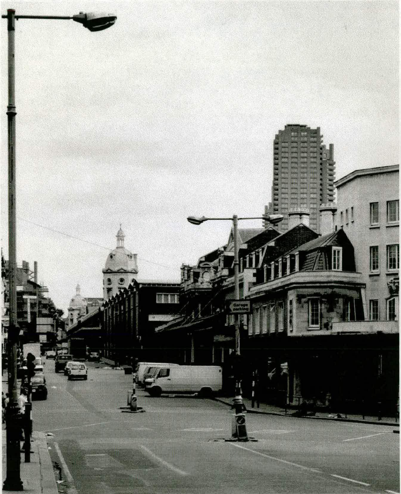
Fig. 5 London Central Markets, view along Charterhouse Street (BB87/7216, ©Crowncopyright.NMR)
