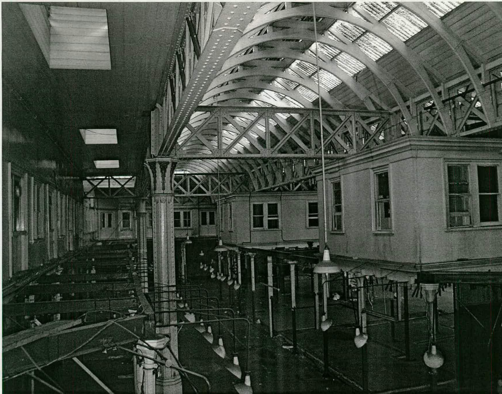
Fig. 16 – The modular two-way spanning framework of lattice girders and Phoenix columns, supporting laminated-timber roof trusses (DP001752, copyright ©English Heritage).
