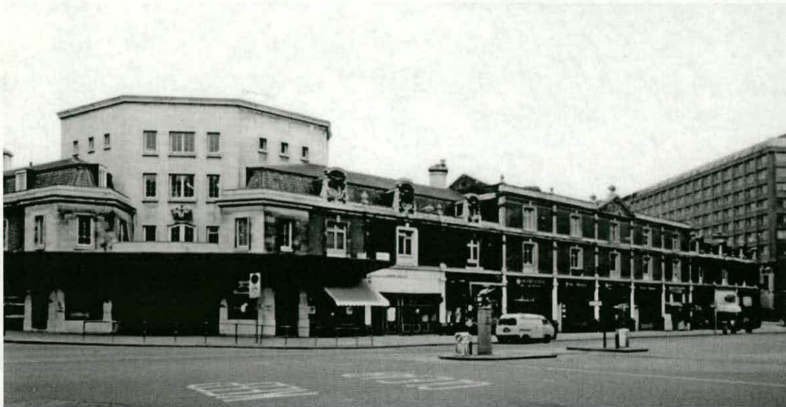
Fig. 7 – West elevation and corner tower of General Market (B880558, copyright © English Heritage).
