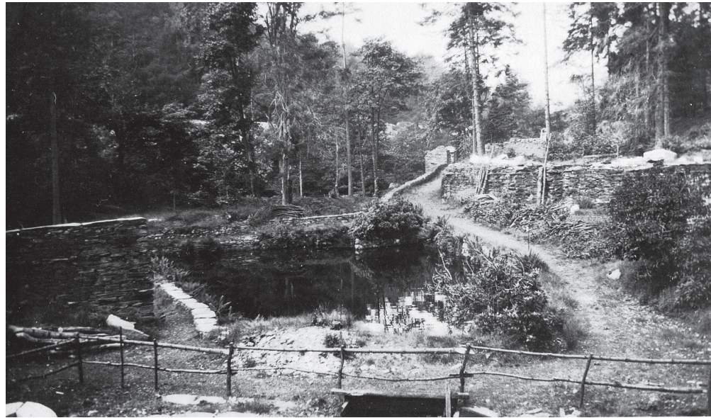
Figure 24. View west across the lower mill pond in the 1930s. The old lower charge house (building 4a) is in the middle distance; blast wall BW1 is at left of frame; while the edge of the wheel-pit to incorporating mills 1 and 2 is just visible at bottom of frame. (Barter collection, copyright reserved)
