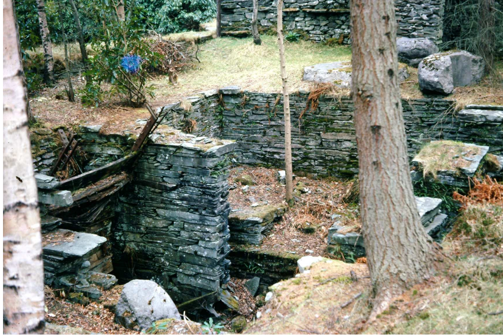
Figure 34. The Rennie's Hatch at mills 3 and 4, photographed in March 1967. Note the flywheel-pit and start of the longitudinal slot visible in the far gear chamber behind the stub wall. (Davies-Shiel collection, copyright reserved)
