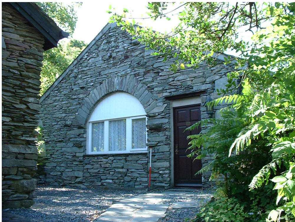
Figure 13. The southern gable of the saltpetre store (building 26), showing the blocked cart entrance
