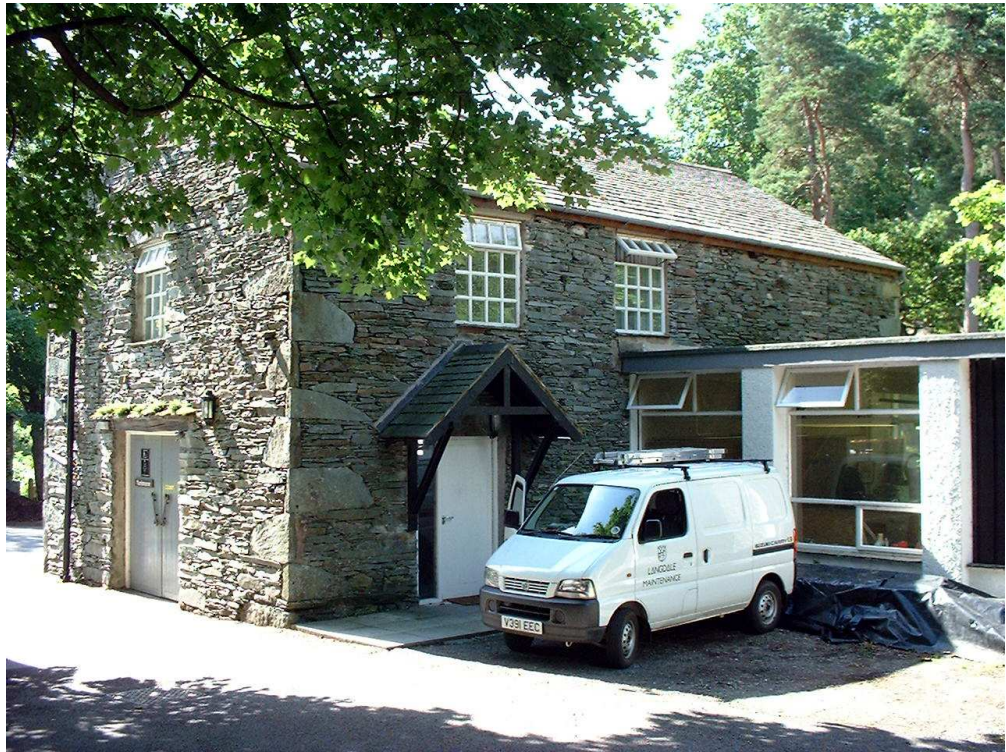
Figure 8. The corn mill/heading mill (building 47) from the north
