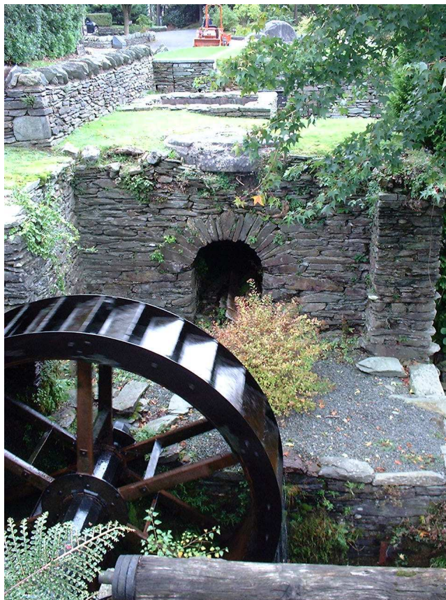
Figure 45. View north-east from above the wheel-pit in mills 9 and 10, showing the vaulted passage through the platform of mill 10
