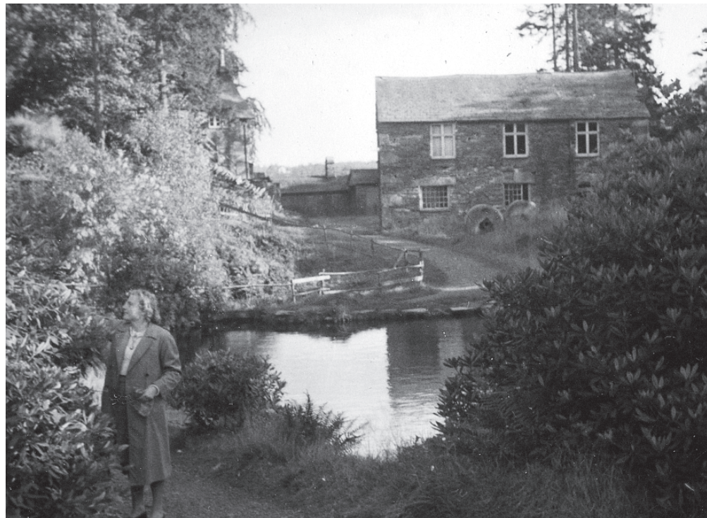
Figure 28. View east across the lower mill pond towards the heading mill (building 47) in the 1960s. The rock-cut gear chambers for the original pair of incorporating mills (nos. 1 and 2) are located behind the fence on the far side of the pond. (Barter collection, copyright reserved)
