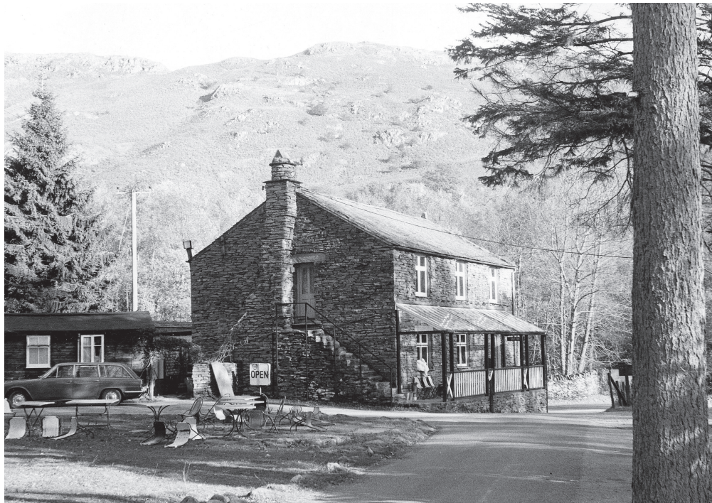
Figure 62. The saw pit (building 33) in use as the Gateway Cafe in the 1960s (Barter collection, copyright reserved)
