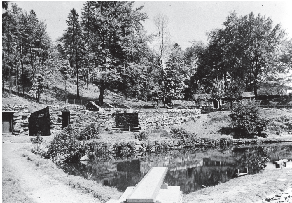
Figure 41. A 1960s photograph of the southern facade of mills 7 and 8 showing the blocked door openings. The unroofed walls of the old lower watch house (building 3) - with the three openings in its front wall - can be seen behind, whilst its replacement (building 2), by this time converted into a private residence called Brackens, lies to the right. (Barter collection, copyright reserved)
