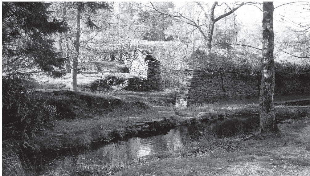
Figure 48. Blast walls BW4 and BW5 from the west in the 1960s (Barter collection, copyright reserved)
