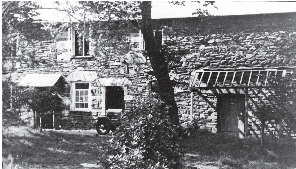
Figure 20. The charcoal store (building 31) during conversion in the 1930s into holiday cottages. The porch at left of frame is the entrance to the later upper watch and change house (building 30). (Barter collection, copyright reserved)
