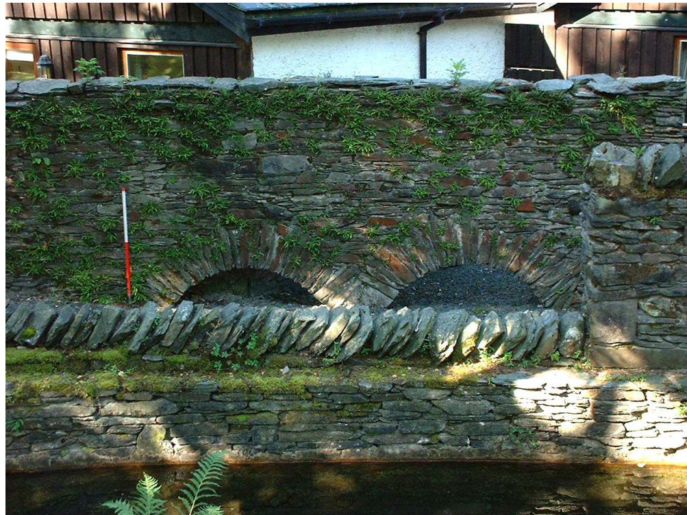
Figure 49. Arches through blast wall BW5, possibly marking the line of the former leat to the press house
