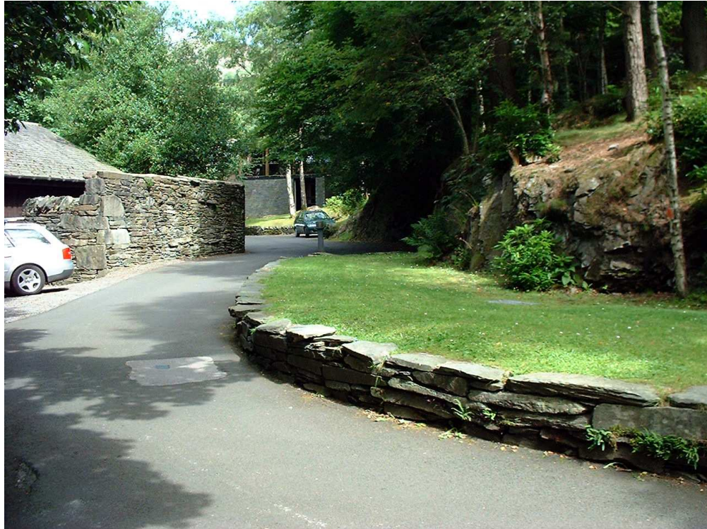
Figure 12. The leat supplying incorporating mills nos. 5-8 at the lower mill site, now infilled and grassed-over. The ruined walls of building 67 are visible at left of frame
