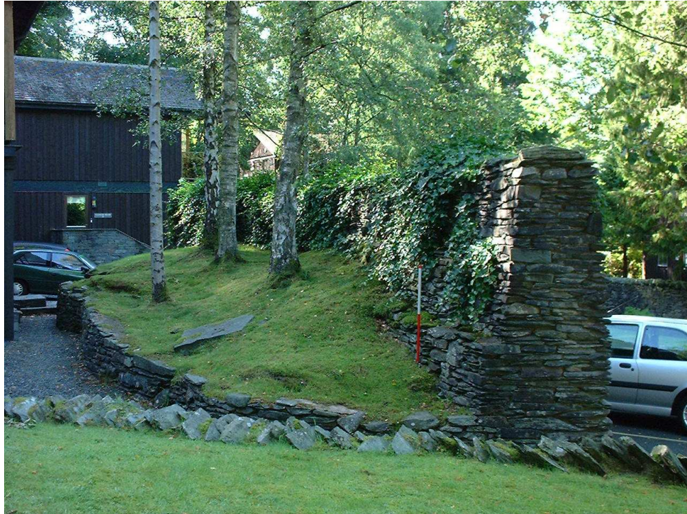
Figure 53. Blast wall BW3 to the south of glazing house no. 3
