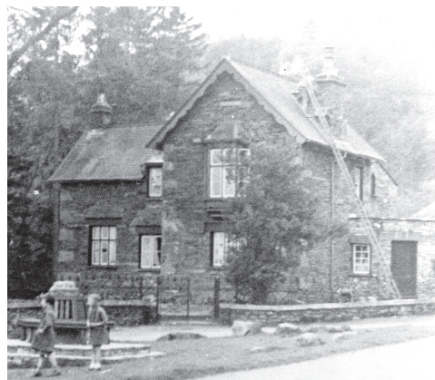
Figure 69. The works' office in the 1930s following conversion (Barter collection, copyright reserved)
