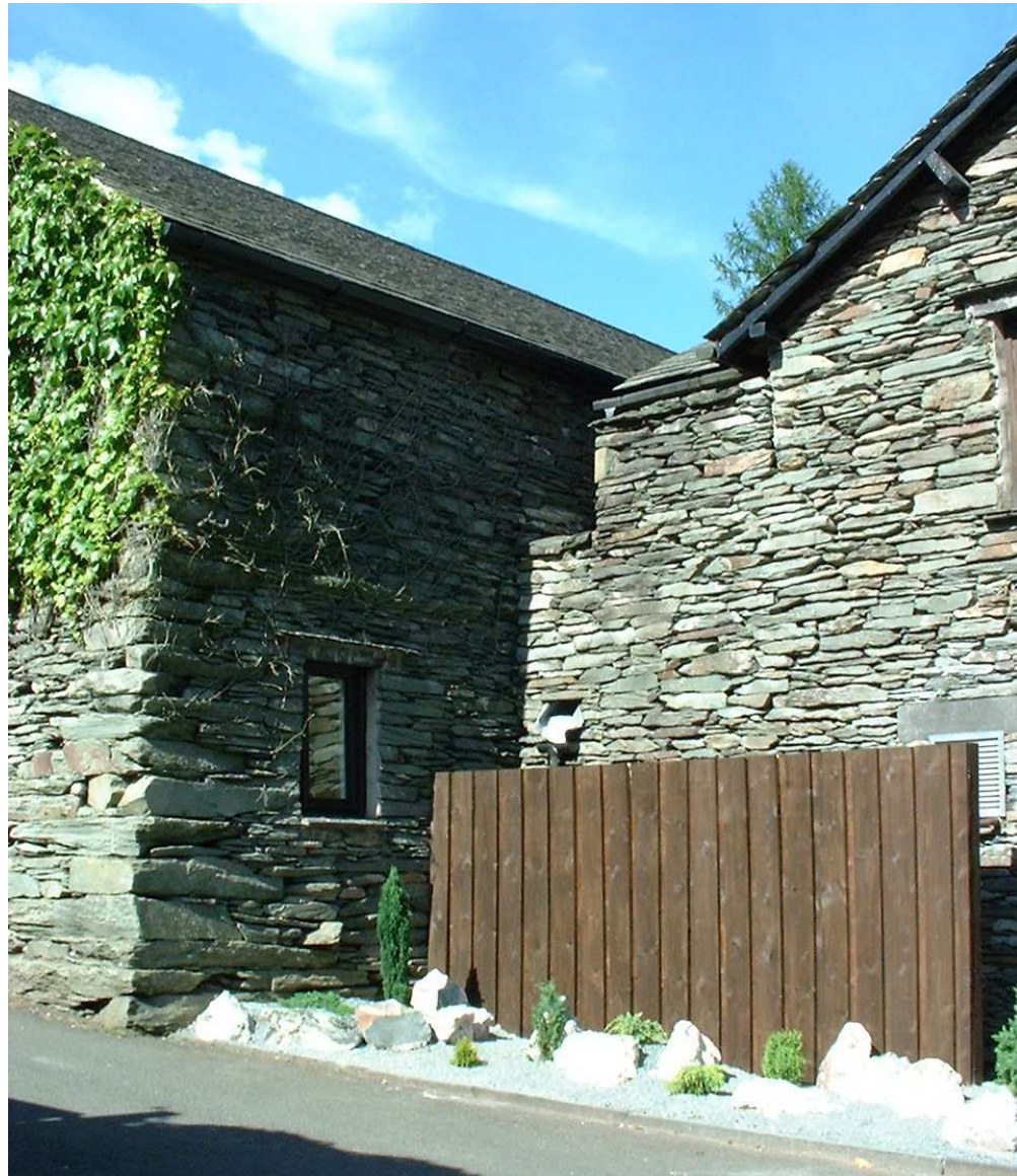
Figure 23. The blocked wheel-pit between the preparing house (building 20) and the saw mill (building 19)
