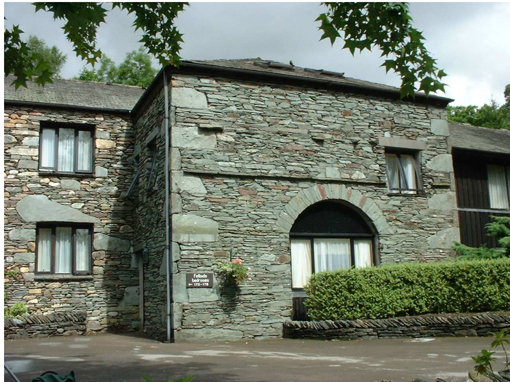
Figure 67. The blocked entrance to the original cart house (building 68), later part of the charcoal store (building 31)
