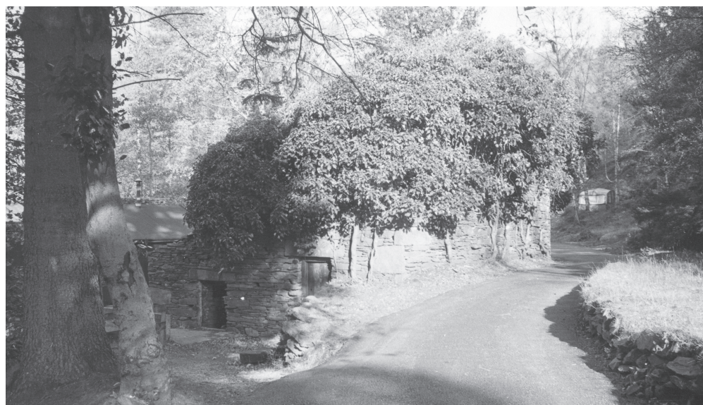
Figure 71. The south-east gable and south- west wall of building 67, photographed in the 1960s. (Barter collection, copyright reserved)
