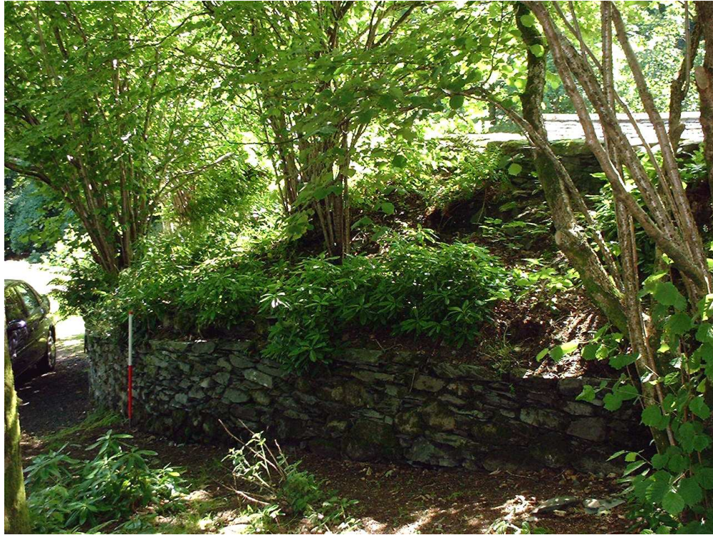
Figure 57. Blast wall BW7 shielding cartridge house no. 1 (building 27)
