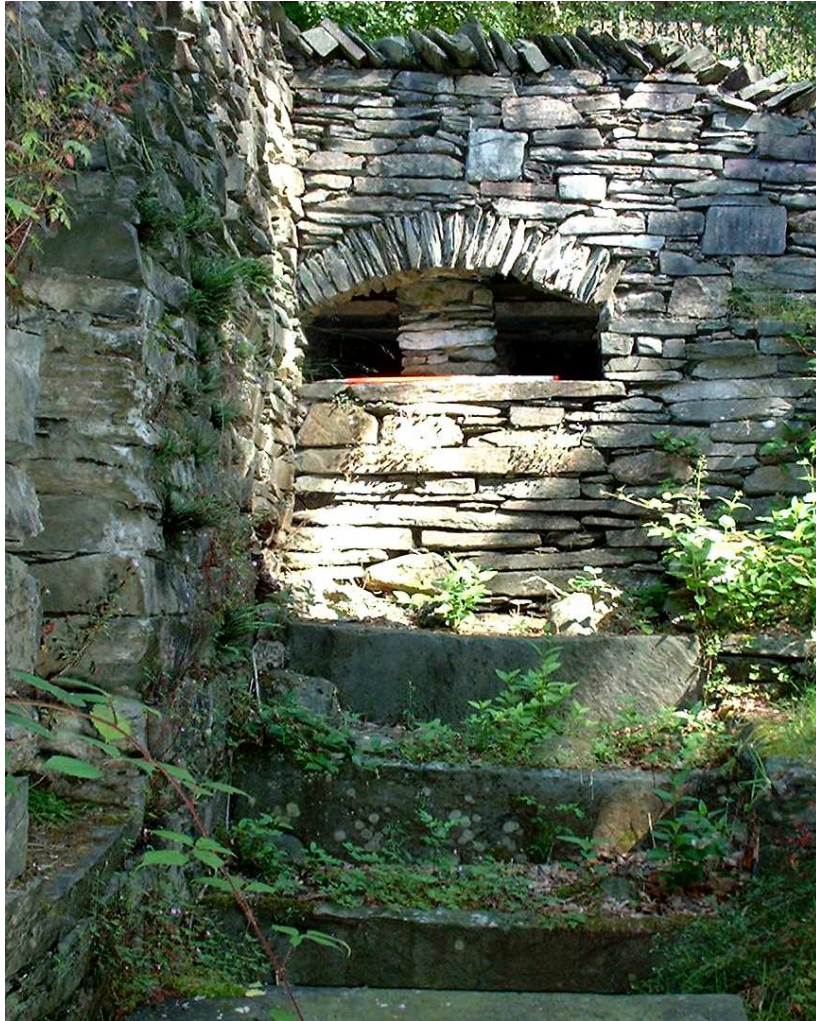
Figure 39. The landscaped wheel-pit between mills 6 and 7
