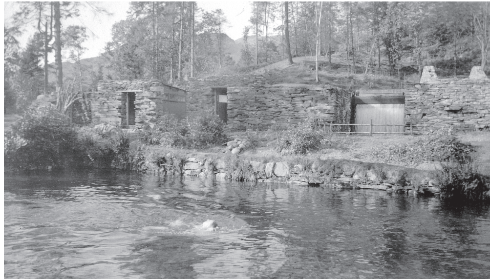
Figure 36. A 1960s photograph of the southern facade of mills 5 and 6. The start of the facade to mill 7 is visible at right of frame. Note the width of the wheel-pit between mills 6 and 7; this housed a wheel powerful enough to drive four mills. (Barter collection, copyright reserved)
