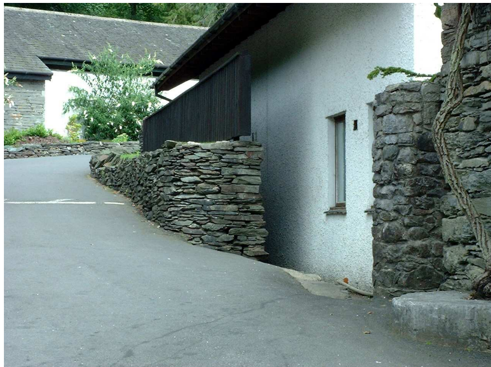
Figure 10. The stone base (now surmounted by a modern fence) for the elevated launder to the preparing house and saw mill
