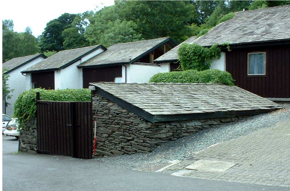
Figure 19. Part of the east end of the saltpetre refinery (building 24), re- used as a garbage enclosure
