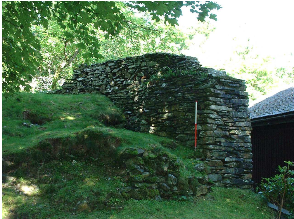
Figure 47. The northern end of blast wall BW4 shielding the press house (building 10)
