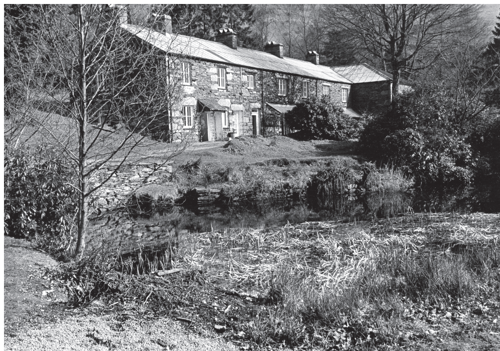
Figure 21. The charcoal store in the 1960s after conversion into holiday cottages. (Barter collection, copyright reserved)
