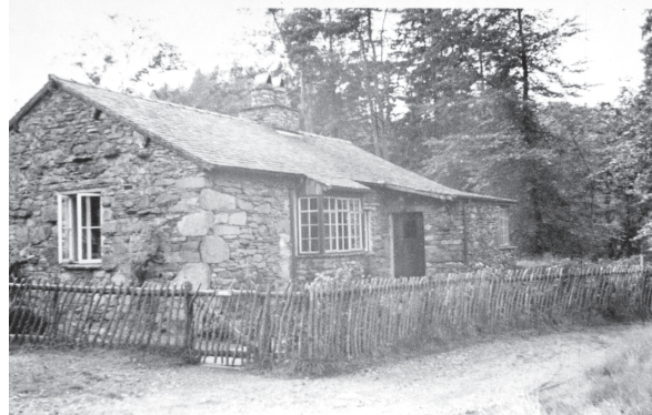
Figure 14. Two views of the sulphur store (building 11) in the 1930s: (top) before and (bottom) after conversion to a private residence, 'Cobblestones'. (Barter collection, copyright reserved)
