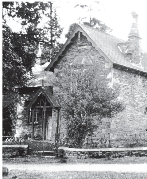
Figure 68. The works' office (building 49) in the 1930s before conversion to holiday accommodation. (Barter collection, copyright reserved)
