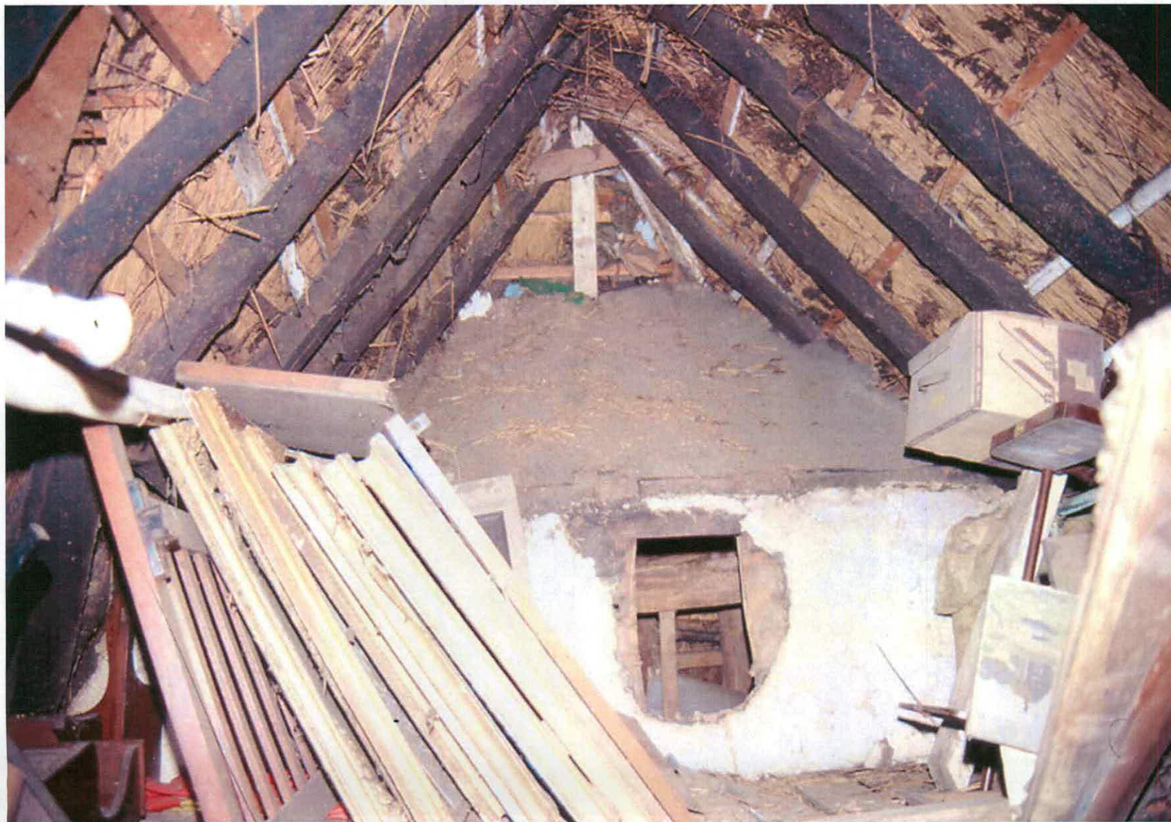
Figure 17 Interior of roof space looking west, showing smoke-blackened roof timbers and sloping ceiling over solar chamber. Photo taken in 1995
