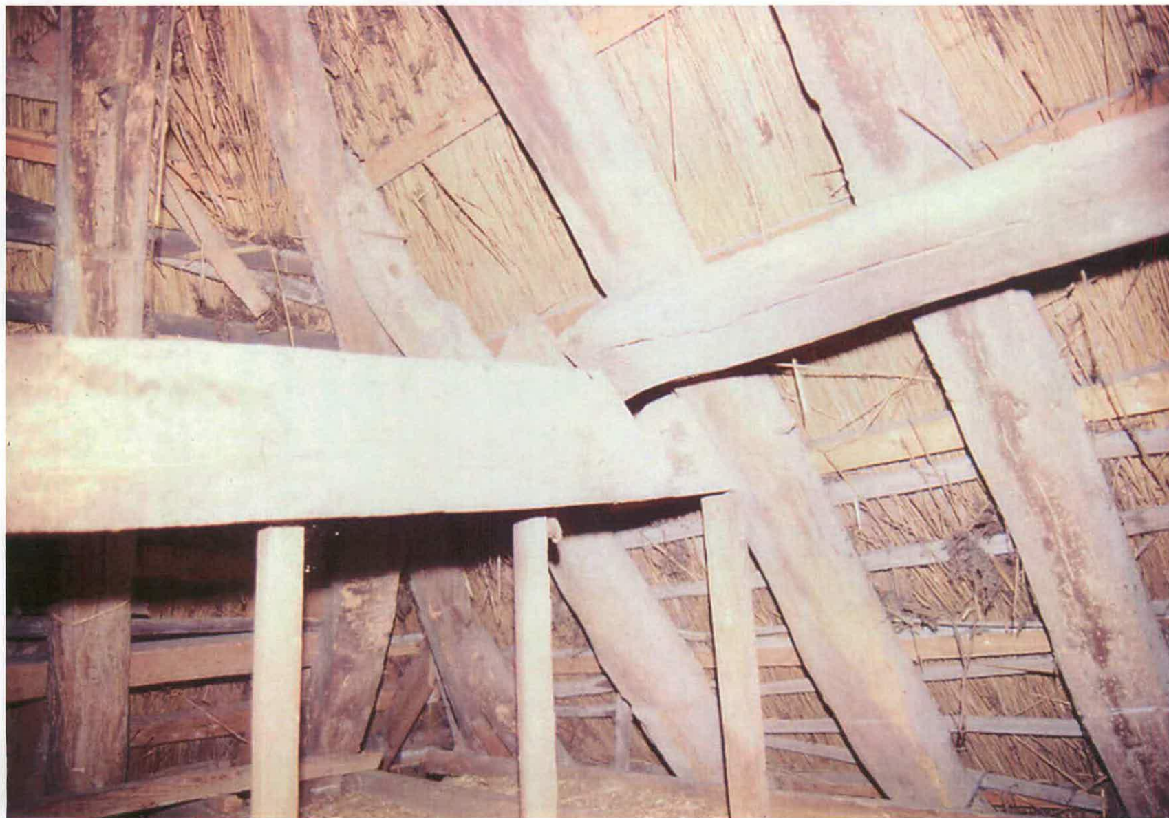
Figure 18 Interior of roof space over west (solar) chamber. Note the absence of smoke-blackening on the original roof timbers. Photo taken in 1995
