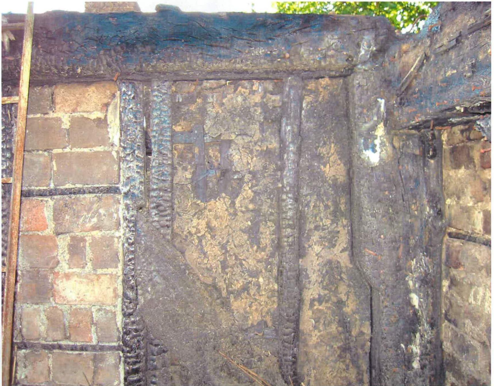
Figure 26 Original late-medieval infilling of timber frame at north end of east intermediate cross frame
