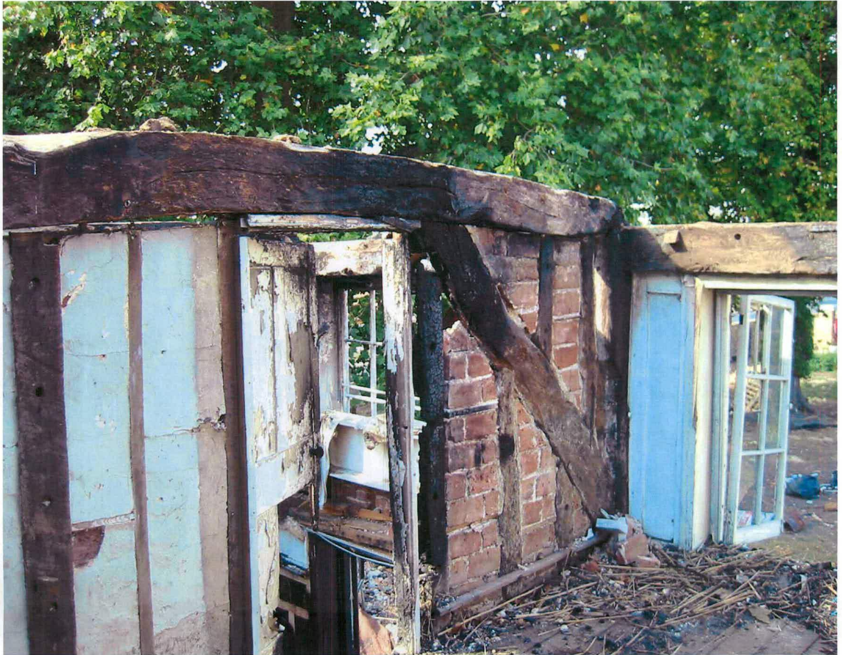
Figure 24 Framing of upper part of west intermediate cross frame following the fire in June 2003
