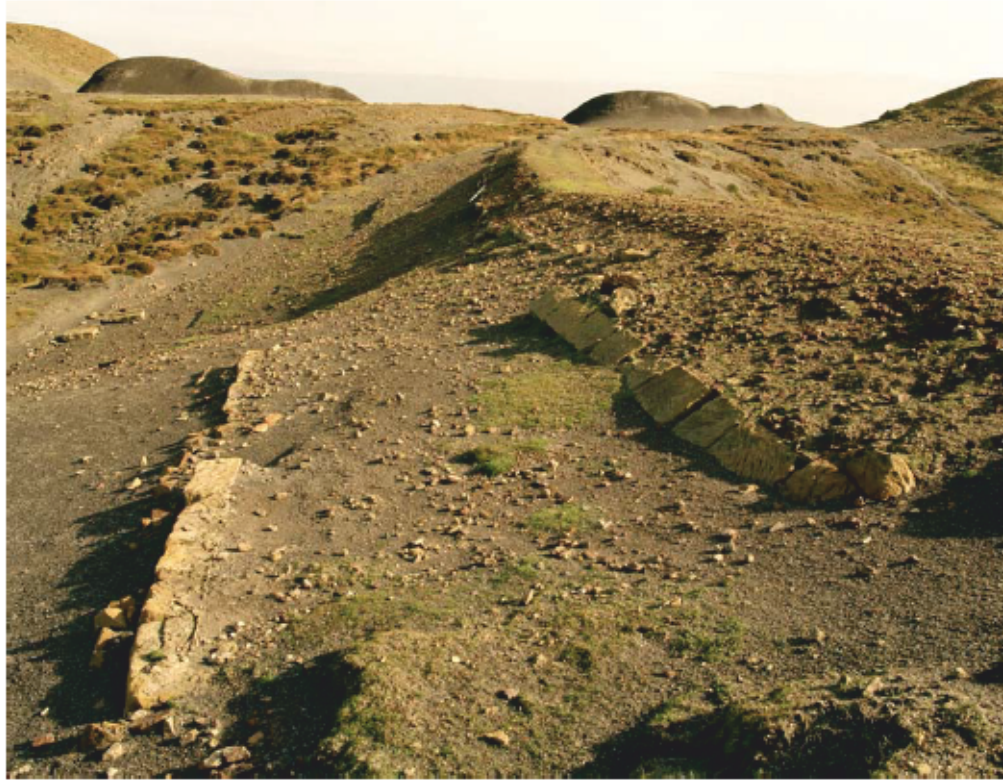
Figure 40. Building 2 from the south-west. Note the traces of rendering on the inside of the left-hand wall (NMR AA040270)
