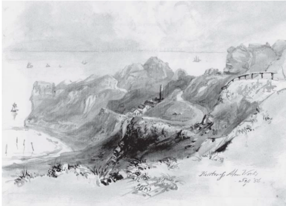
Figure 9. Sketch of Kettleless Alum Works (WLPSL PEF351), dated September 1856 and thought to be by Mary Weatherill (Whitby Literary and Philosophical Society, copyright reserved)
