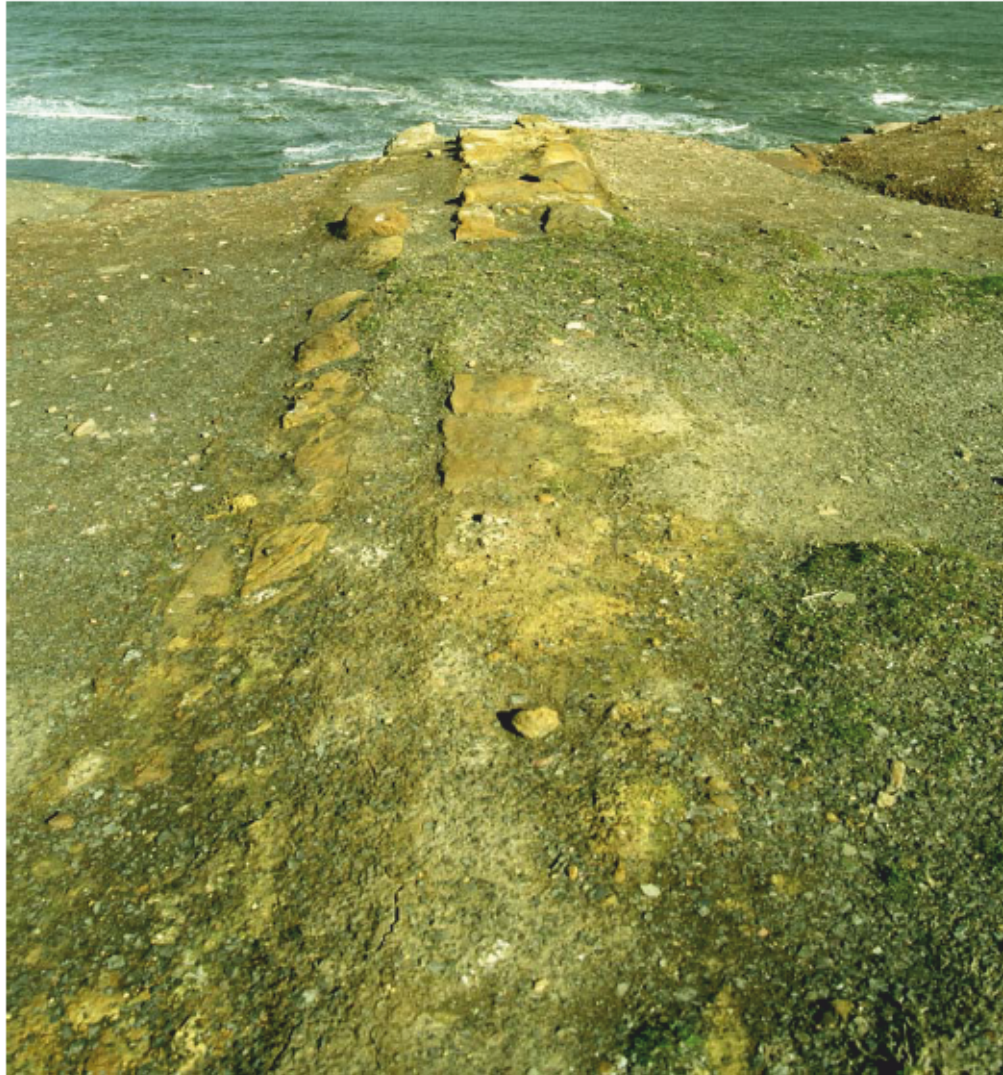
Figure 26. Detail of the void between the side walls of steeping pits 5 and 6. (NMR AA040259)
