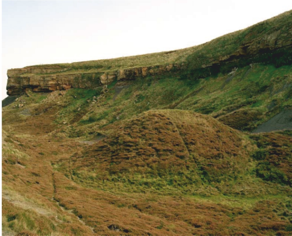
Figure 13. General view of the east end of the main quarry face, showing the eroded shale undercliff and the surviving dесс in the sandstone cap. The mound in the foreground is allegedly an undismantled calcining clamp, but is more probably a simple spoil heap. (NMR AA040208)
