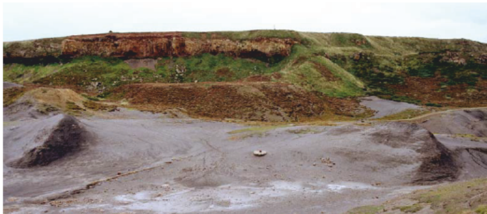
Figure 14. General view of the central portion of main quarry face, showing in-situ and eroding sections of the sandstone cap. The shale baulks in the foreground are the remains of calcining places 3 and 4. The two ends of the coastguard breeches buoy are also visible. (NMR AA040261)
