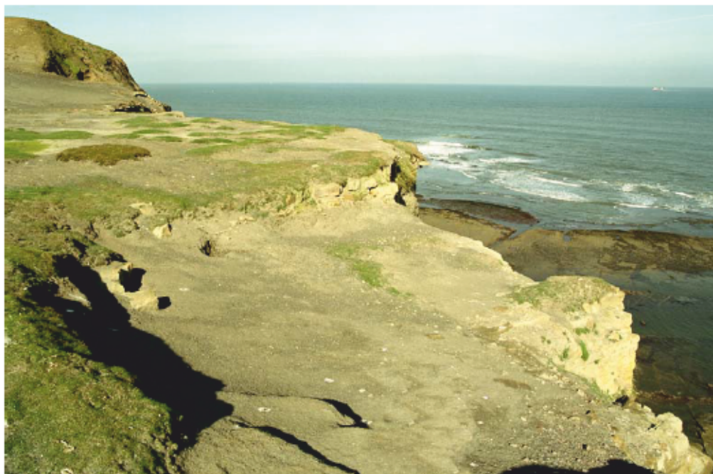
Figure 41. The surviving south- western end of building 3. The roof of the liquor-trough tunnel is just visible at left of frame. (NMR AA040223)
