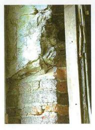
Figure 24. Cut through window head on the first floor of the 1670-72 south range
