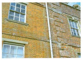
Figure 23. Detail of the south front showing the south west corner of the 1650s building and quoins (right) and the 1670-72 addition (centre and left). The orange brickwork is a recent alteration following the removal of a mid-19th-century bay window.
