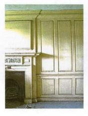
Figure 30. Early 18th-century panelling in a closet off the Japan Room on the first floor
