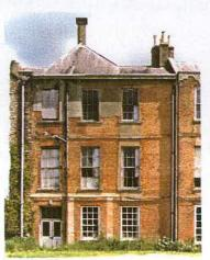
Figure 40. West elevation of the White Hall range, from the service court, showing the former loggia at basement level
