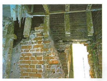
Figure 7. Part of the south end wall of the White Hall range (foreground) built against the earlier gable end wall of the Green Room range. The cut-away timber framing dates from the 1740s
