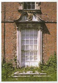
Figure 22. Detail of the doorway in the centre of the east front. Note the scars of an earlier and wider opening
