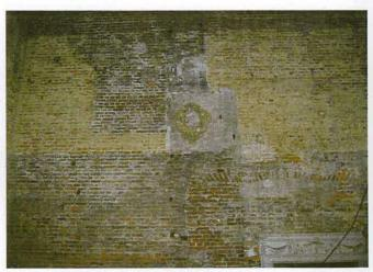
Figure 28. Detail of the south wall of the great dining room showing (bottom right) the round arch of the early 17th-century fireplace opening, and within that a later, flatter arch of c.1670
