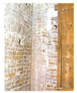
Figure 9. The south-west corner of the great dining room showing (centre and right) the former external wall of the White Hall range and bricked up window (behind board) area which, perhaps in the late 17th century, was converted into a servants' hall. For a discussion of the main rooms in this part of the house, see below, **p. 19**.
