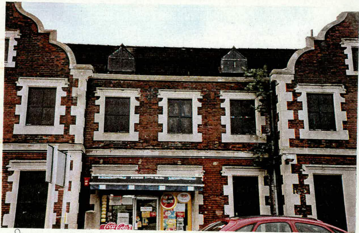
fig. 10 Detail of storefront and windows on west elevation of Hampton Court Station.
