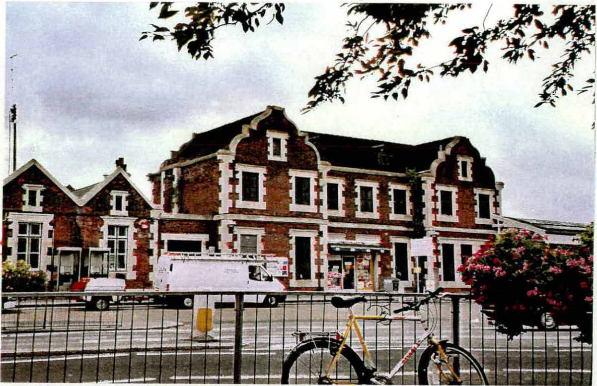
fig. 4 west elevation of Hampton Court Station
