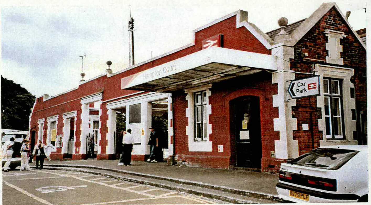
Fig. 6 Screen wall and entrance at north end of Hampton Court Station.
